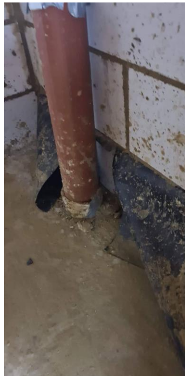
Plate 6. Utility Service Cast Into Raft Construction
