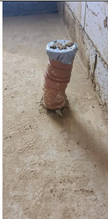
Plate 5. Utility Service Cast Into Raft Construction
