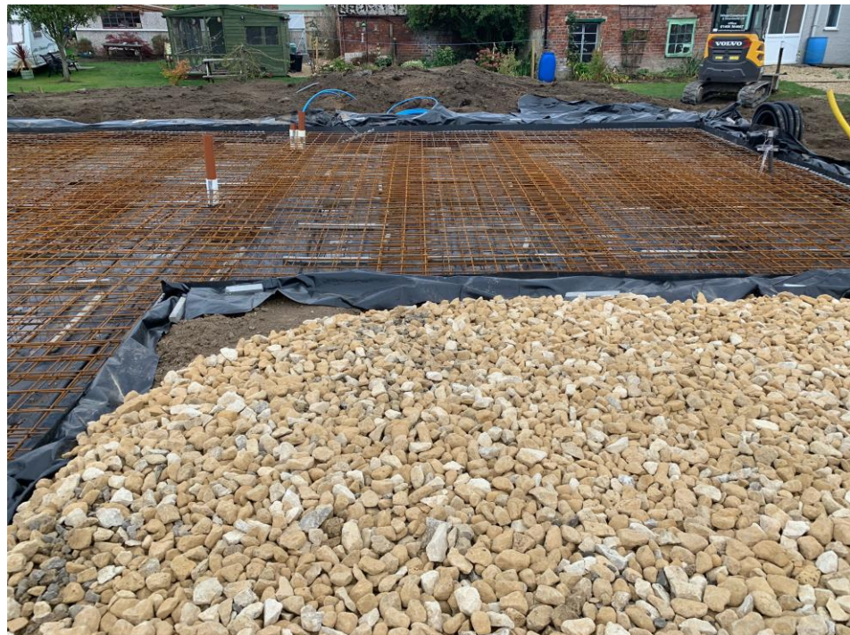
Plate 4. DPM and Reinforcement Placed
