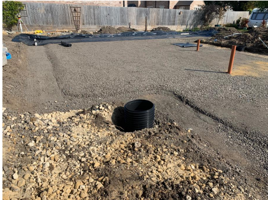
Plate 1. Topsoil Removed, Utilities Installed and Compacted Hardcore Placed
