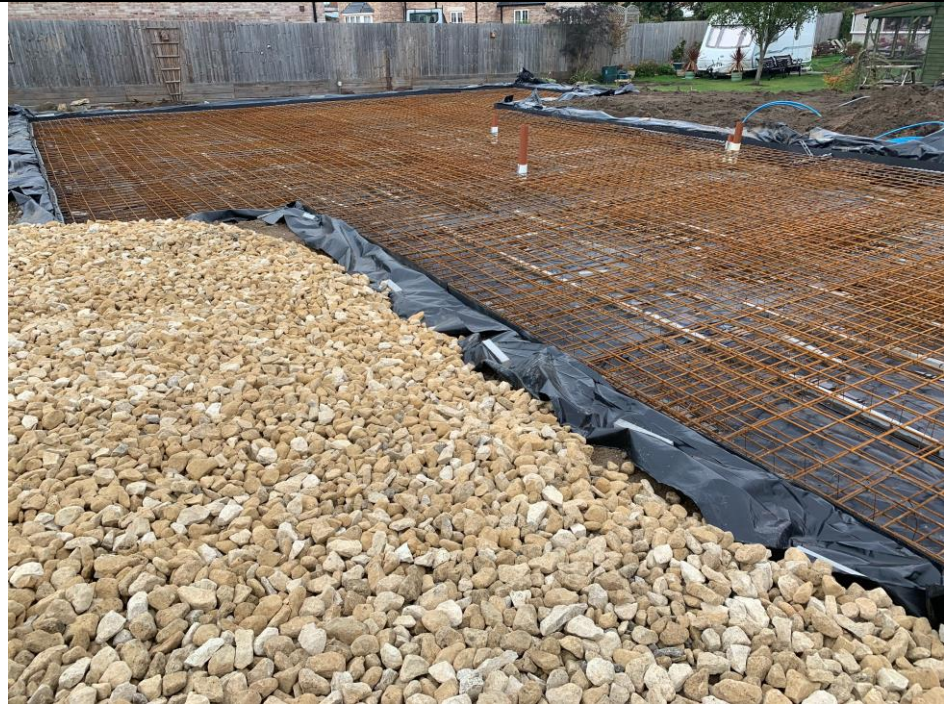
Plate 3. DPM and Reinforcement Placed
