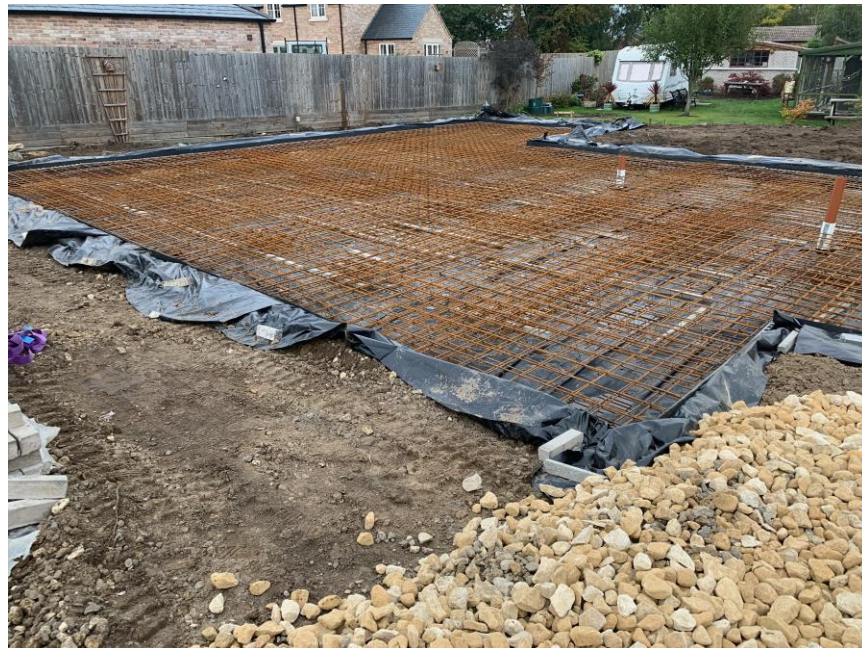
Plate 2. DPM and Reinforcement Placed
