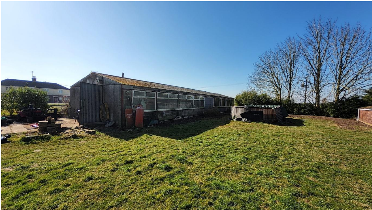
Photo 1. Existing garage/car workshop (26777804)
