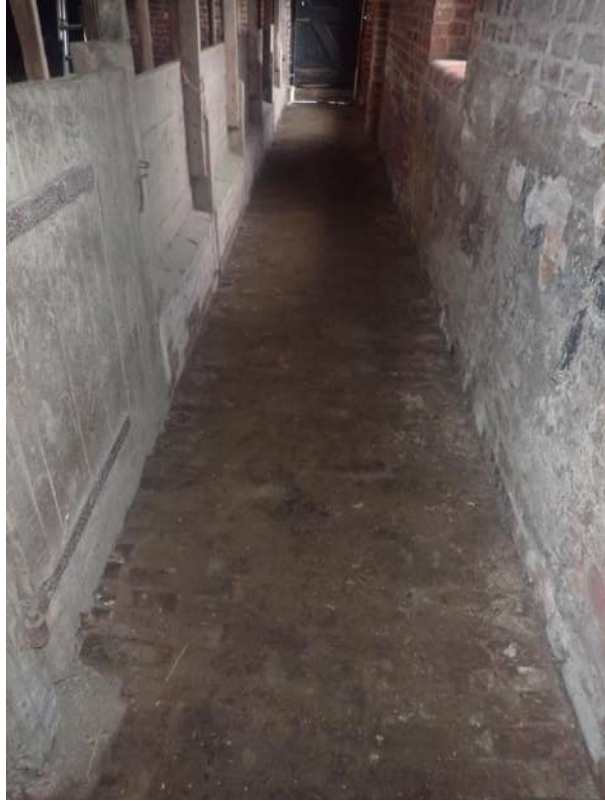
Plate 233: View of the flooring of the northern passageway of Cell 6, from the east
