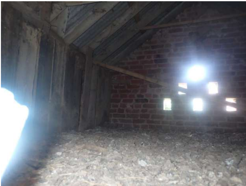
Plate 199: View of the interior of the former dovecote, from the east
