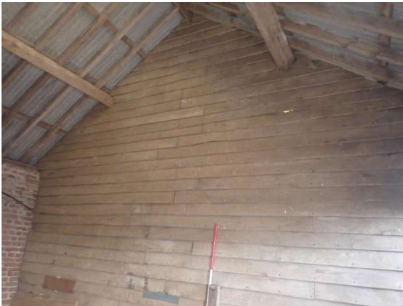
Plate 155: View of the west wall of Cell 4, from the east
