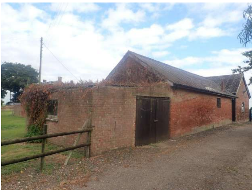
Plate 9: General view of the outbuilding complex, from the south-east
