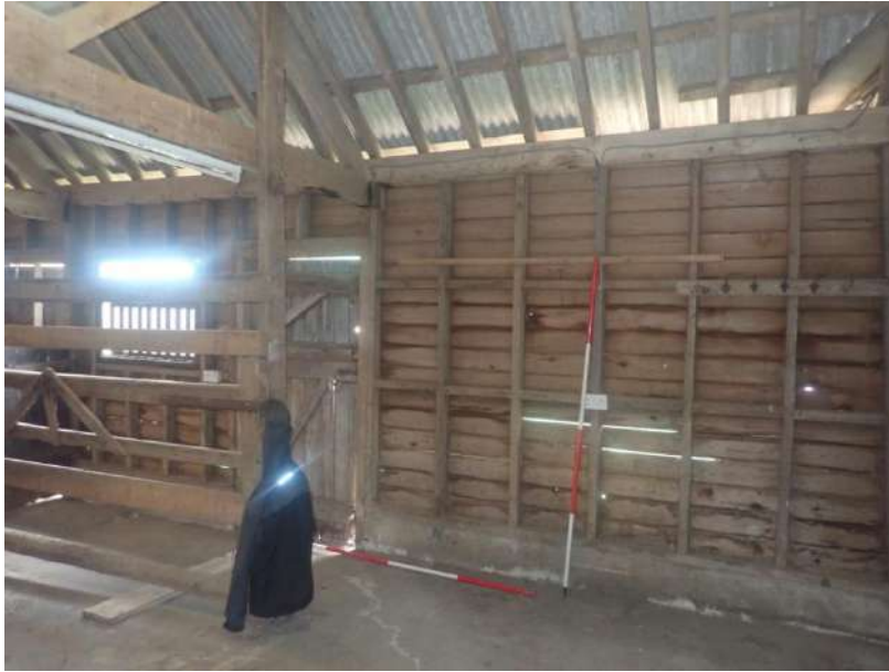
Plate 59: View of the west wall of Cell 1, from the east
