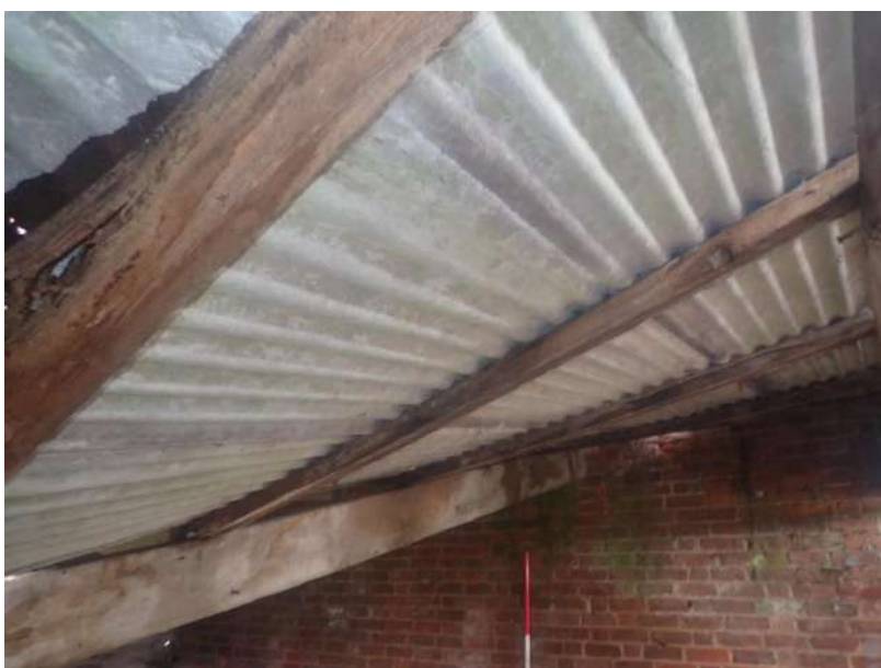
Plate 16: View of the roof supporting structure of the modern lean-to/garage, from the east
