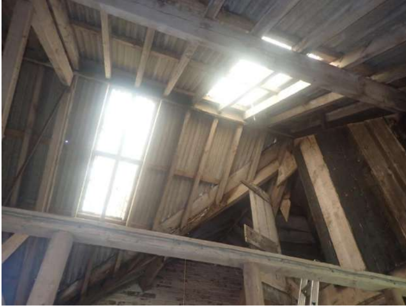
Plate 229: View of the roof supporting structure of Cell 6, from the north
