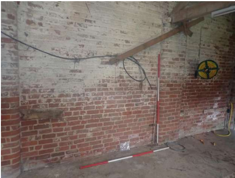
Plate 197: View of the south wall of Cell 6, from the north-east
