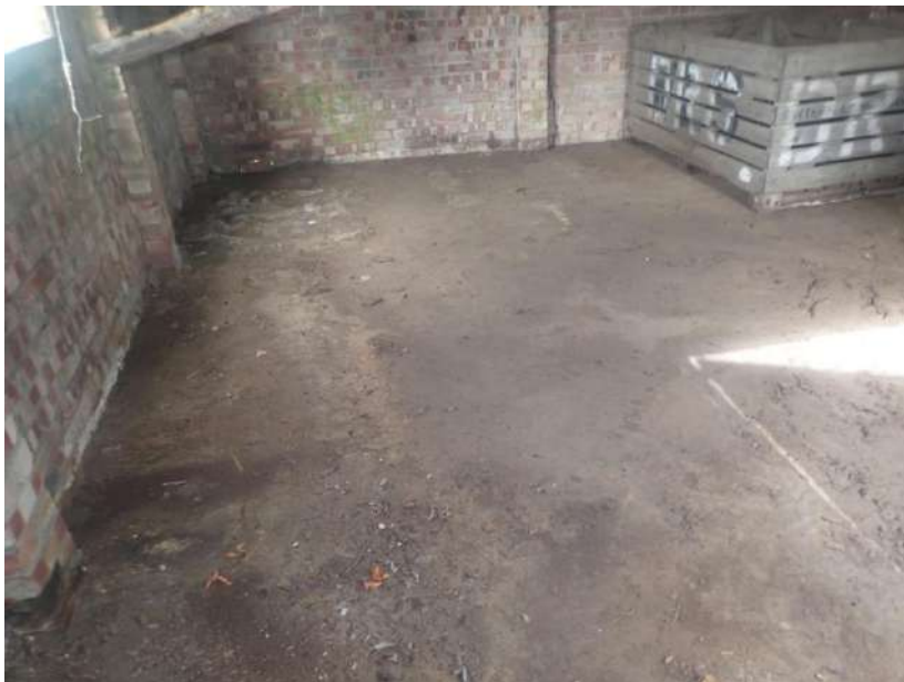
Plate 14: View of the flooring of the modern lean-to/garage, from the east
