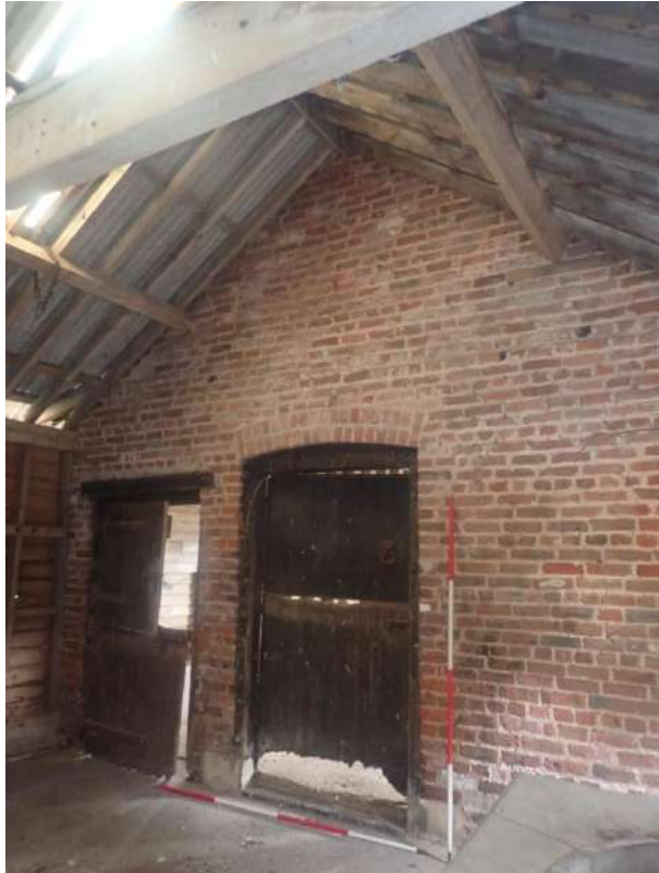
Plate 45: View of the north wall of Cell 1, from the south
