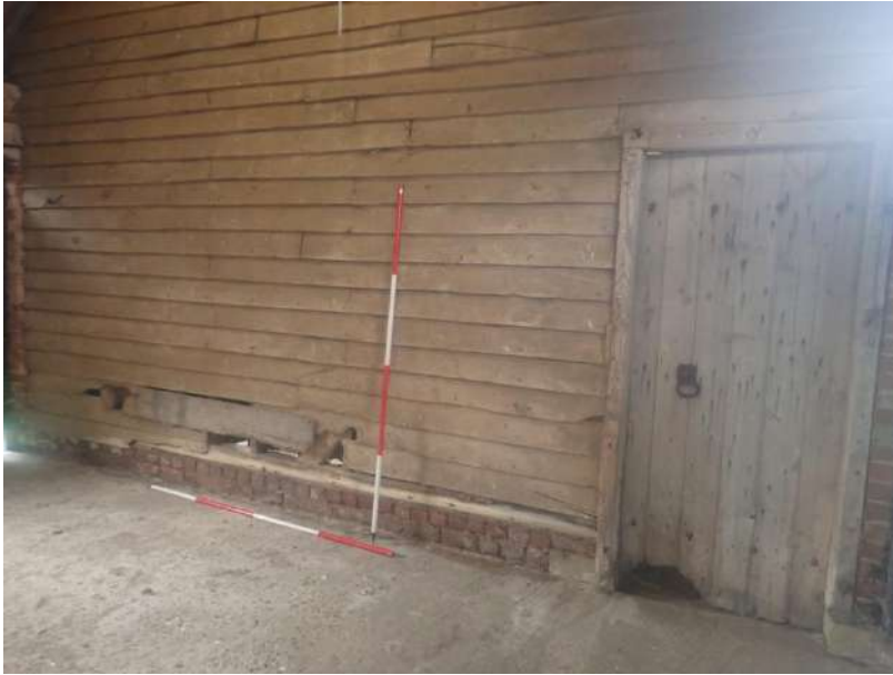
Plate 176: View of the west wall of Cell 5, from the east
