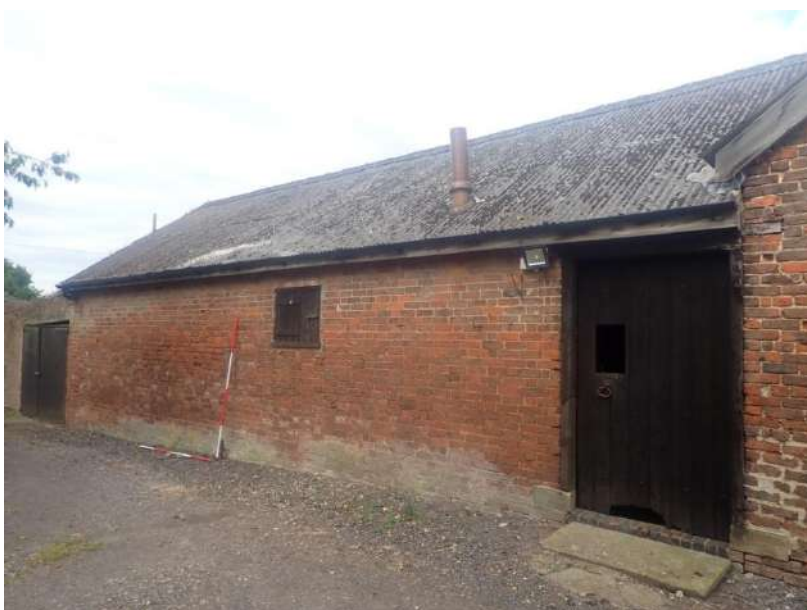
Plate 30: View of the East Elevation of Outbuilding 1, from the north-east
