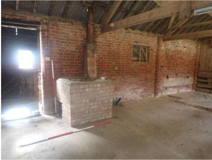
Plate 51: View of the east wall of Cell 1, from the north-west
