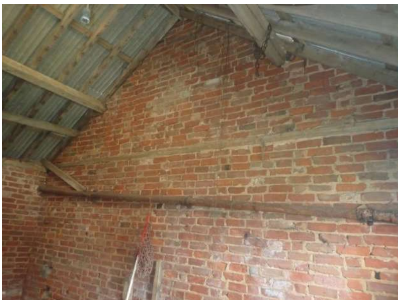
Plate 95: View of the south wall of Cell 2, from the north-west
