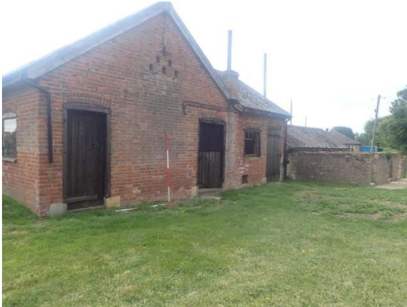
Plate 104: View of the West Elevation of the North Range, from the north-west
