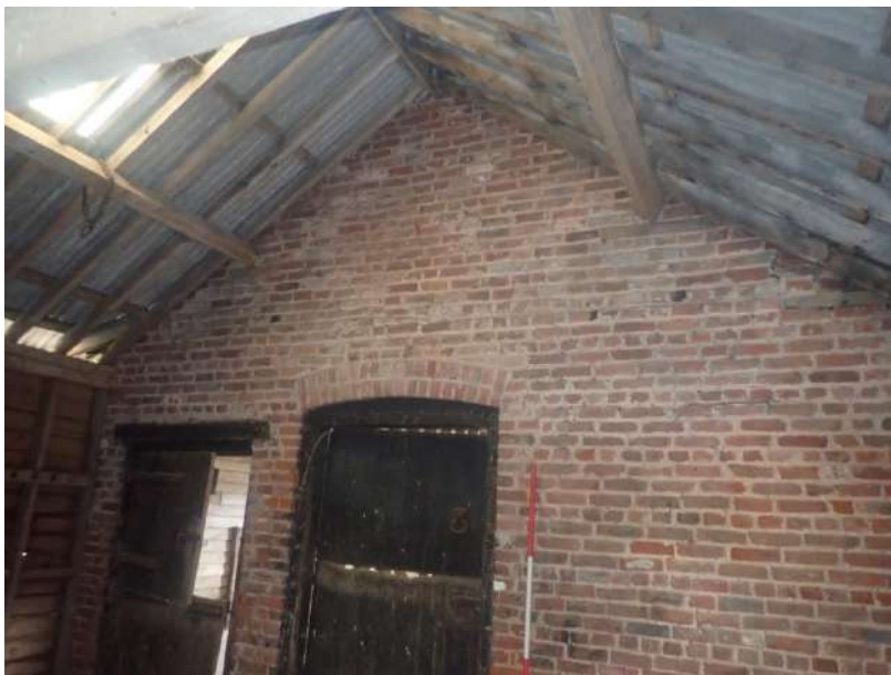
Plate 44: View of the north wall of Cell 1, from the south
