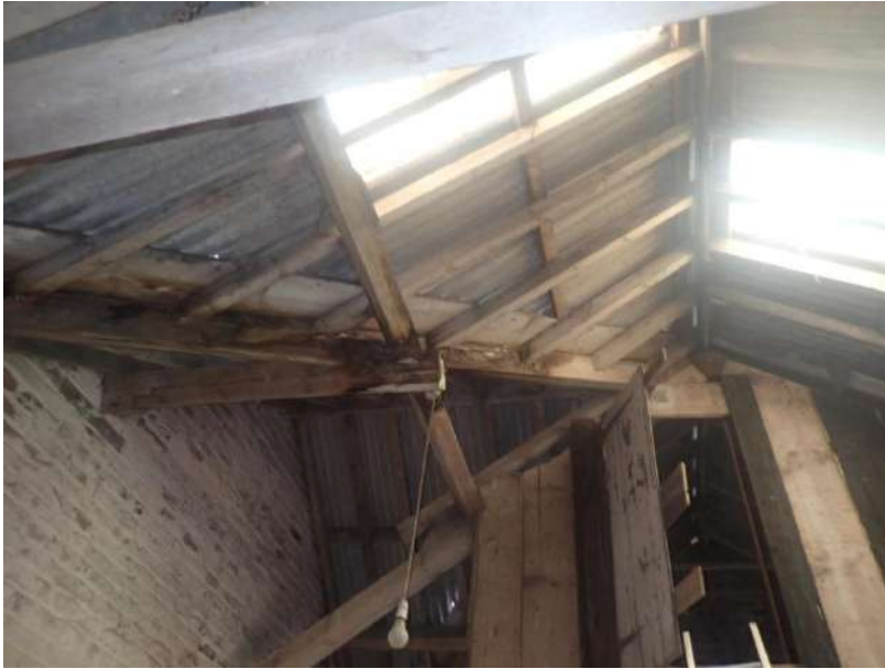
Plate 223: View of the roof supporting structure of Cell 6, from the east
