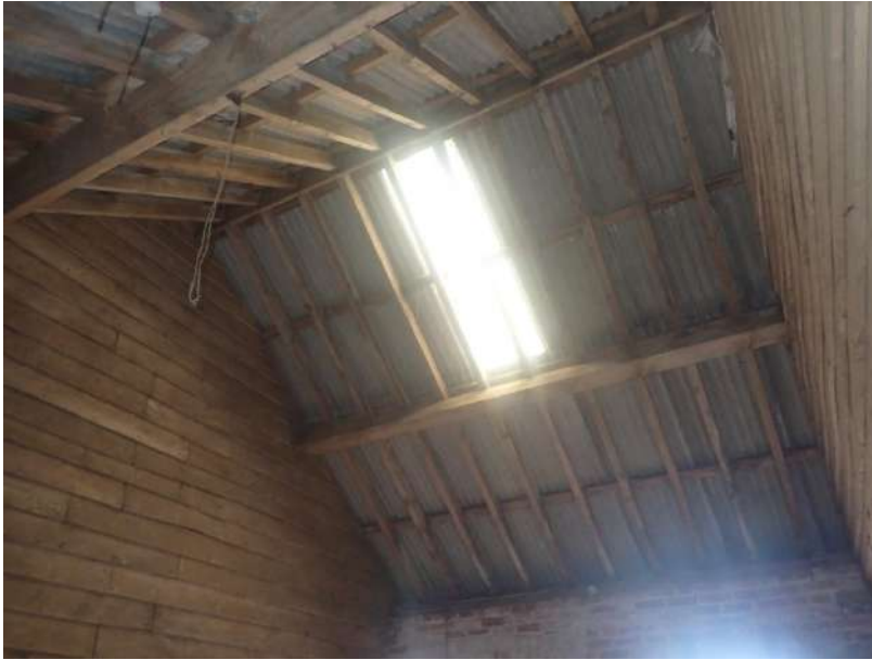
Plate 138: View of the roof supporting structure of Cell 4, from the south
