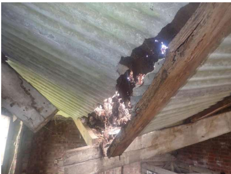
Plate 17: View of the roof supporting structure of the modern lean-to/garage, from the east
