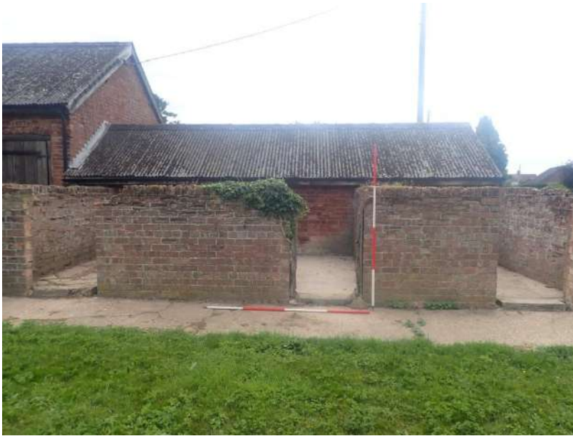
Plate 266: View of the western boundary wall of the piggery, from the west
