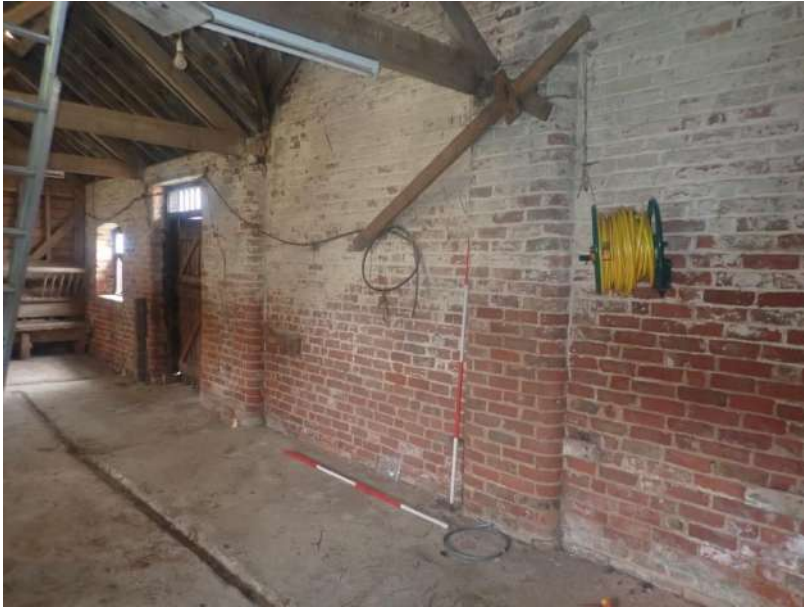
Plate 196: View of the south wall of Cell 6, from the north-west
