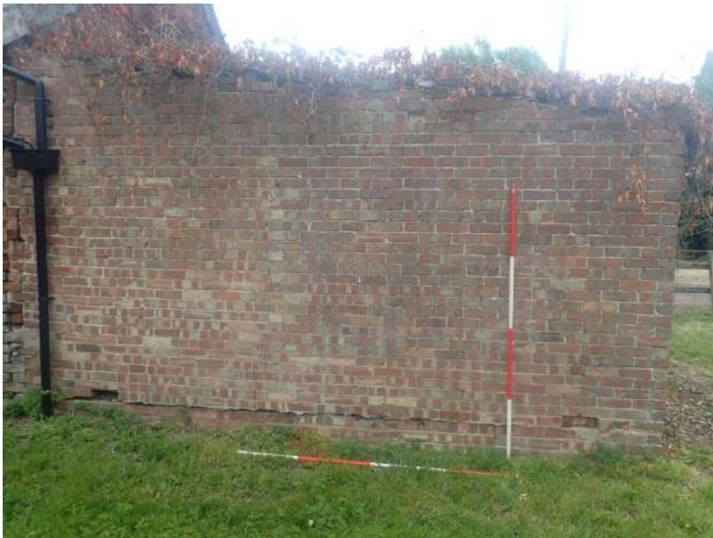
Plate 12: View of the West Elevation of the Modern Lean-to/Garage, from the west
