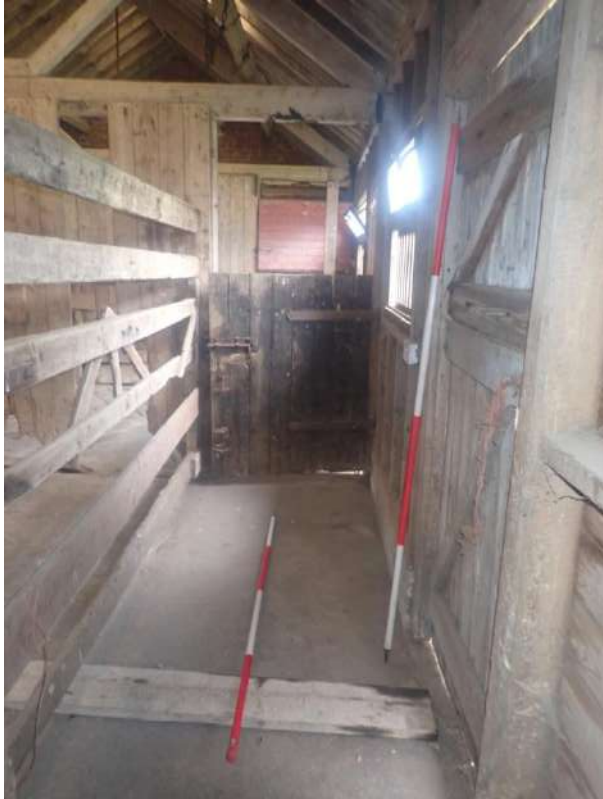
Plate 61: View of the interior of Cell 1, from the north
