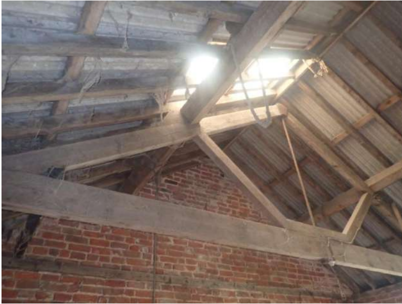
Plate 290: View of the roof supporting structure of Cell 7, from the north
