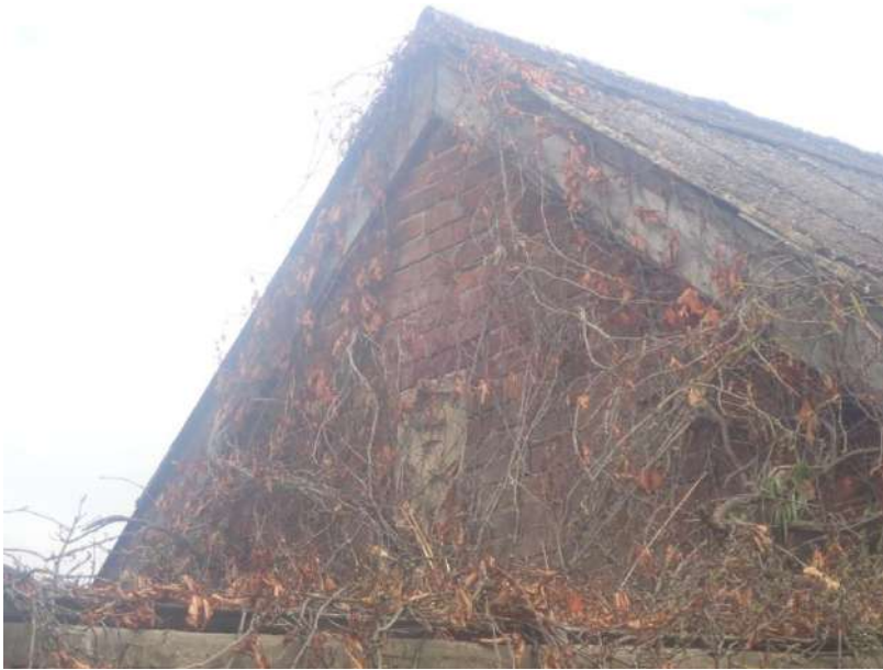
Plate 27: View of the South Elevation of Outbuilding 1, from the south-east
