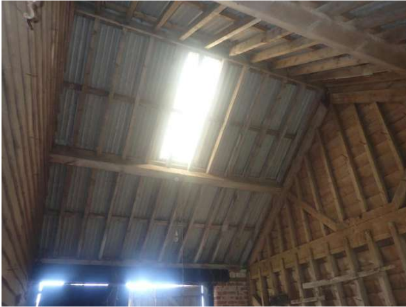
Plate 160: View of the roof supporting structure of Cell 5, from the south
