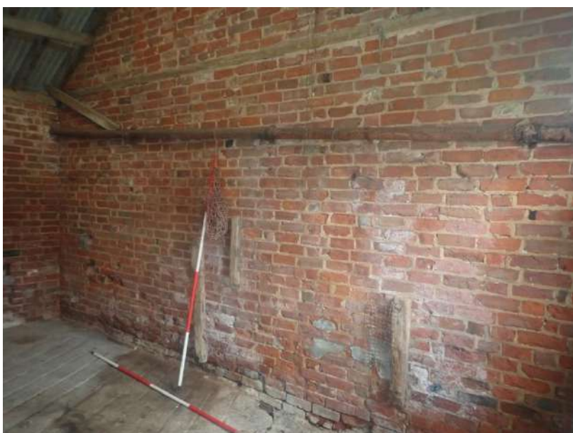
Plate 94: View of the south wall of Cell 2, from the north-west
