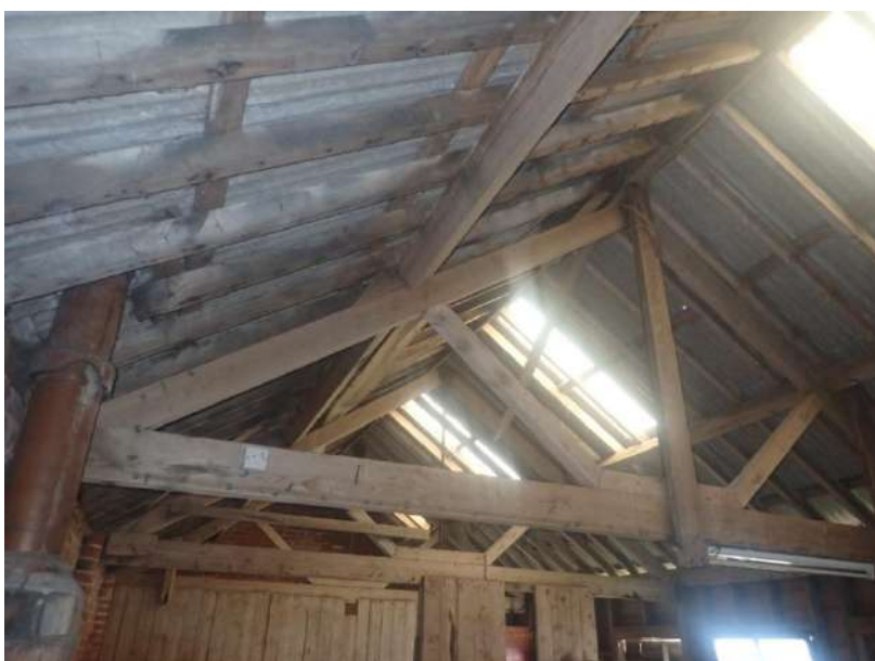
Plate 72: View of the roof supporting structure of Cell 1, from the north
