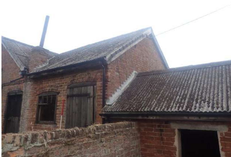
Plate 261: View of the South Elevation of Outbuilding 2, from the south-west
