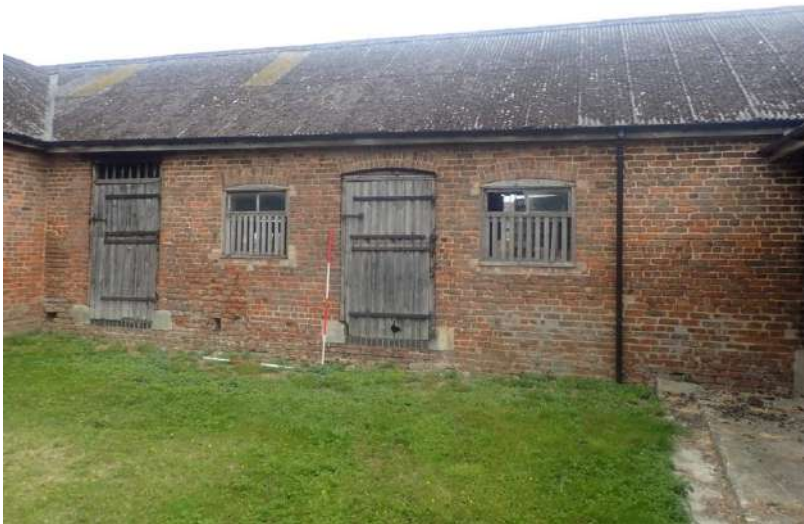
Plate 108: View of the South Elevation of the North Range, from the south
