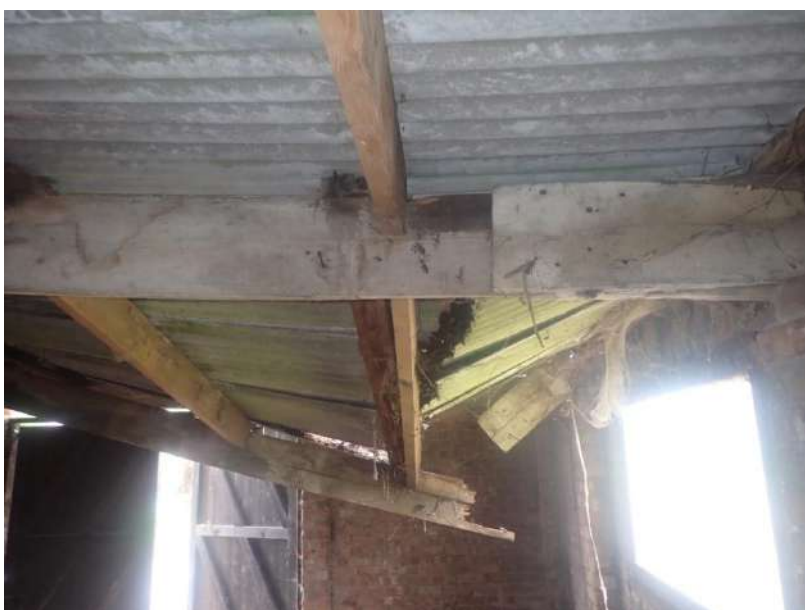
Plate 20: View of the roof supporting structure of the modern lean-to/garage, from the west
