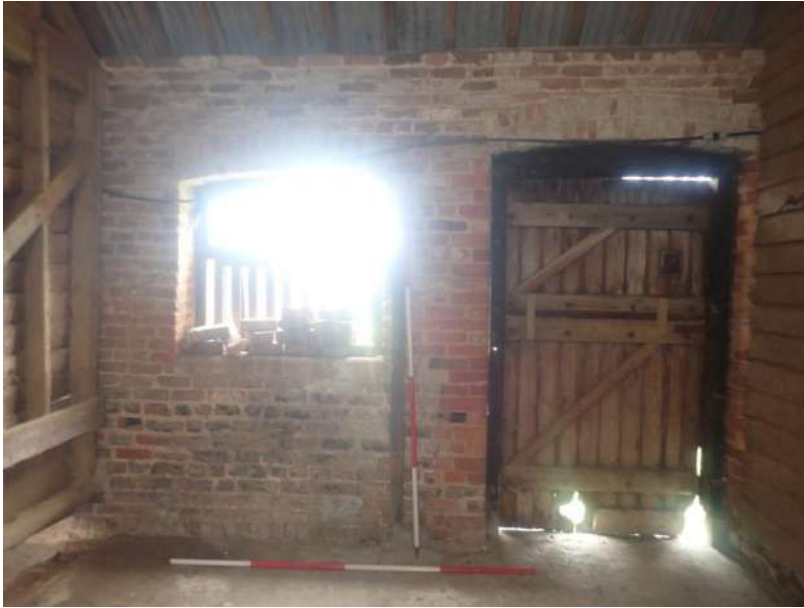
Plate 168: View of the south wall of Cell 5, from the north
