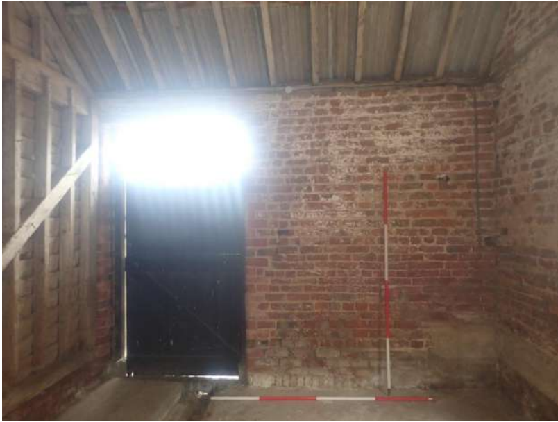
Plate 122: View of the north wall of Cell 3, from the south
