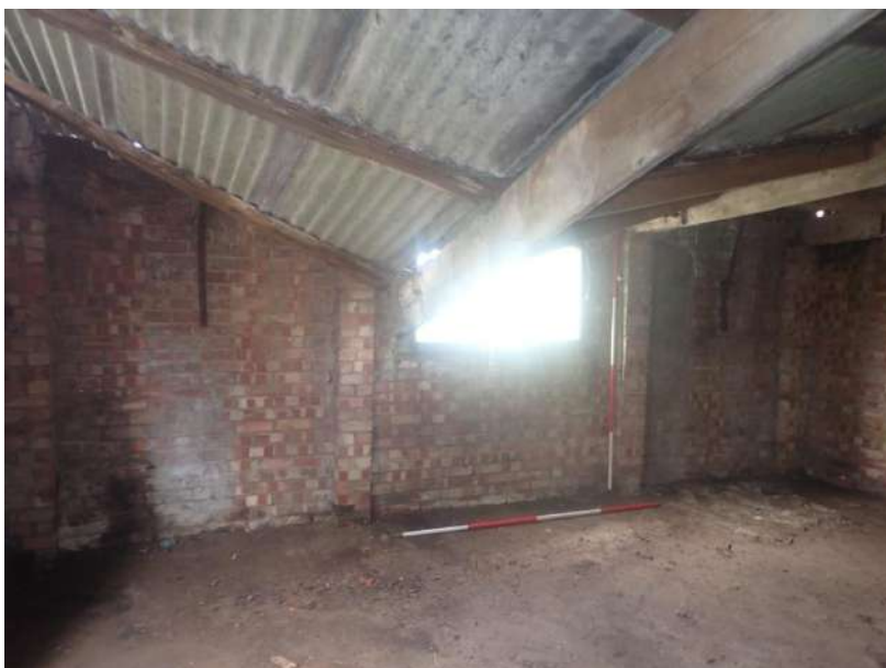
Plate 23: View of the south wall of the modern lean-to/garage, from the north
