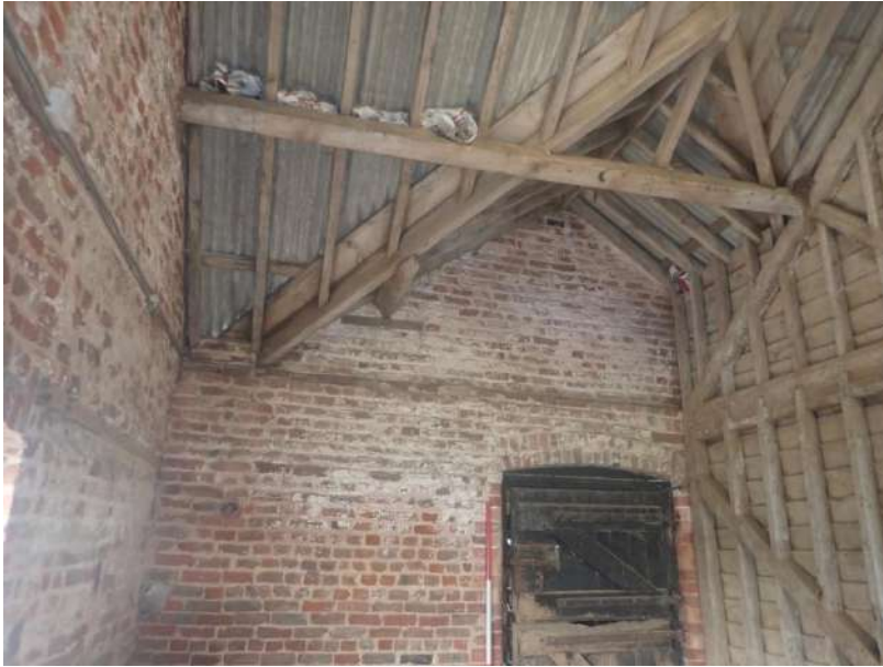
Plate 124: View of the south wall of Cell 3, from the north
