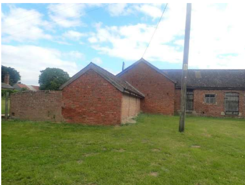
Plate 4: General view of the outbuilding complex, from the south
