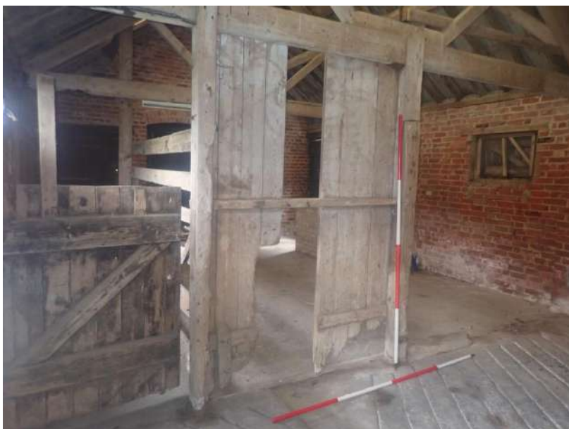
Plate 47: View of the internal timber partition within Cell 1, from the south-west
