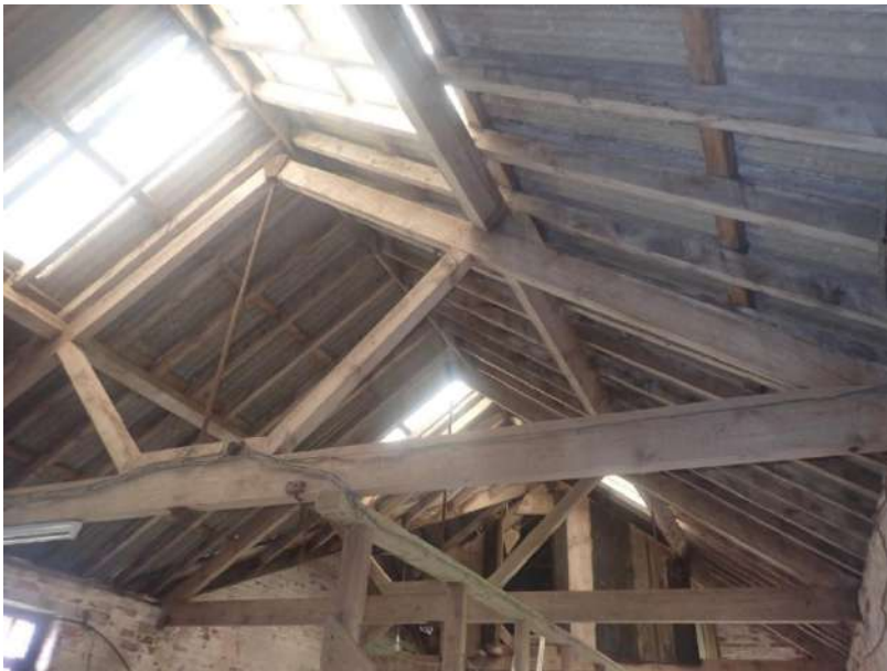
Plate 226: View of the roof supporting structure of Cell 6, from the east
