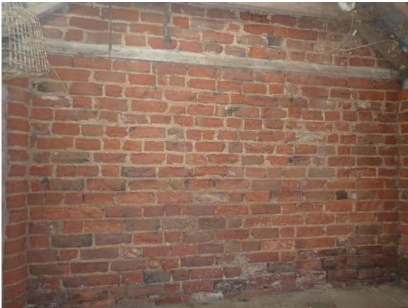
Plate 324: View of the south wall of Stie 3, from the north
