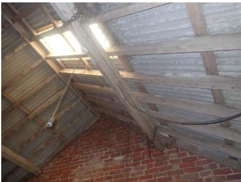
Plate 83: View of the roof supporting structure of Cell 2, from the north
