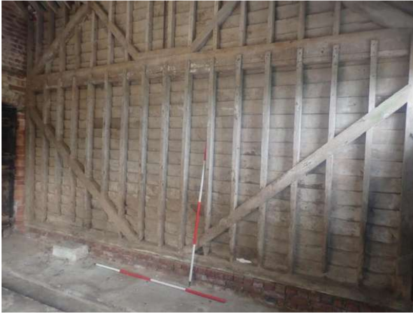
Plate 128: View of the west wall of Cell 3, from the east
