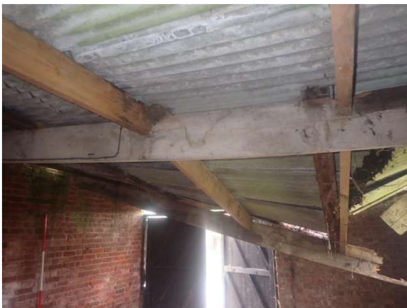
Plate 19: View of the roof supporting structure of the modern lean-to/garage, from the west
