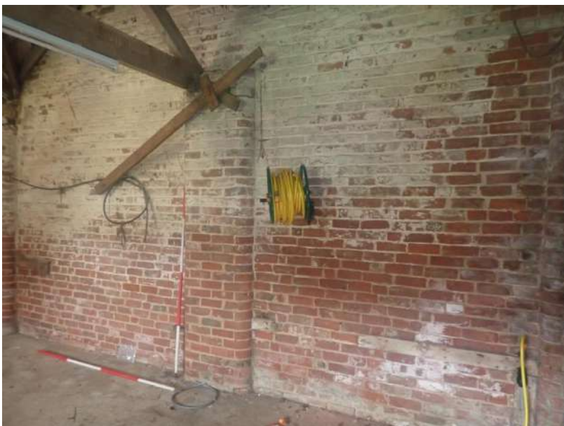
Plate 195: View of the south wall of Cell 6, from the north-west
