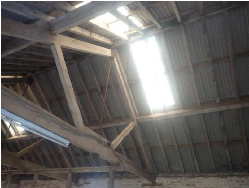
Plate 218: View of the roof supporting structure of Cell 6, from the north-west
