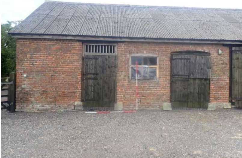
Plate 100: View of the North Elevation of the North Range, from the north
