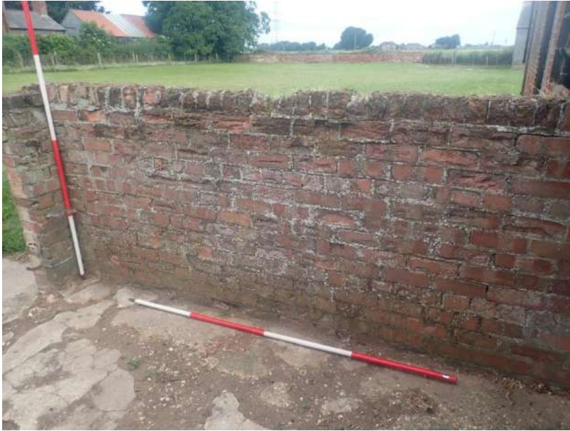
Plate 272: View of the northern yard wall of the first sty, from the south
