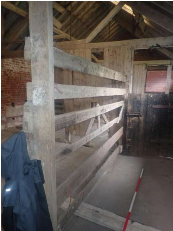
Plate 62: View of the interior of Cell 1, from the north
