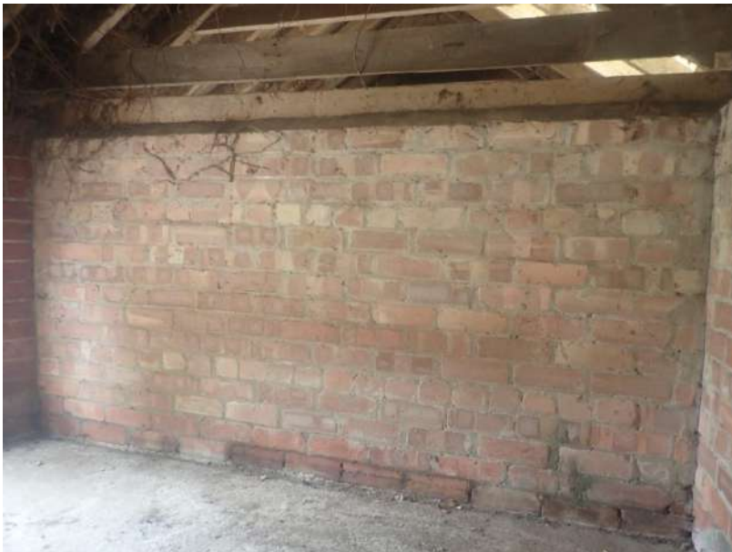
Plate 316: View of the north wall of Stie 2, from the south
