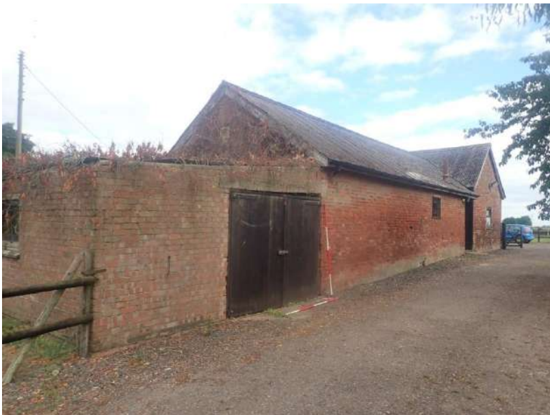
Plate 28: General view of the East Range of the outbuilding complex, from the south-east
