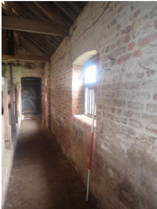
Plate 247: View of the north wall of Cell 6, from the east
