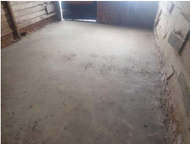
Plate 137: View of the flooring of Cell 4, from the south
