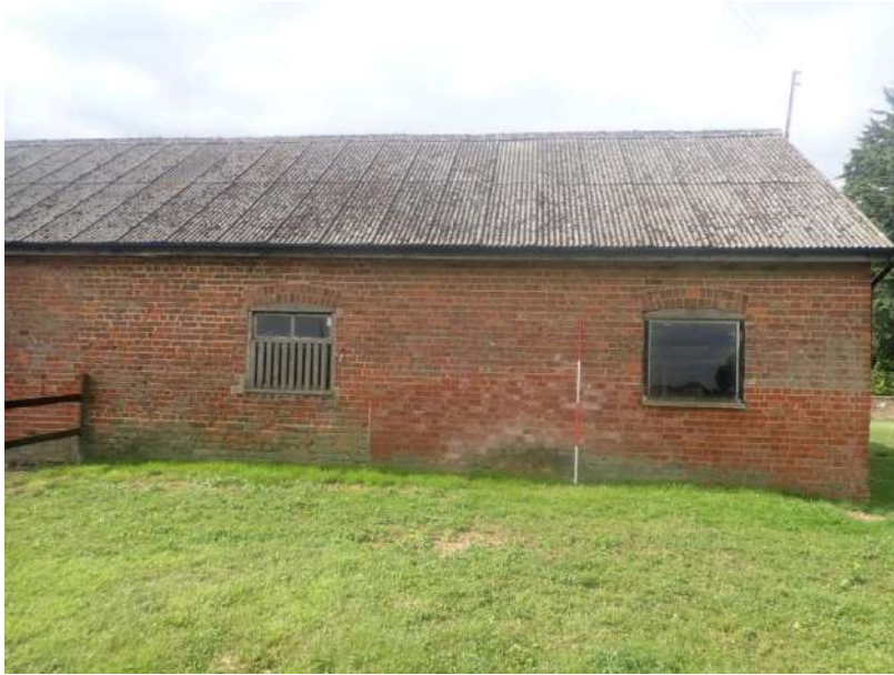
Plate 102: View of the North Elevation of the North Range, from the north
