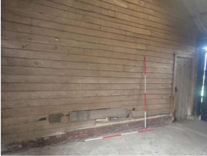
Plate 174: View of the west wall of Cell 5, from the east
