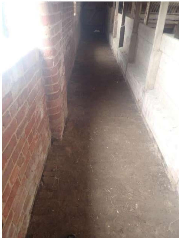
Plate 232: View of the flooring of the northern passageway of Cell 6, from the west
