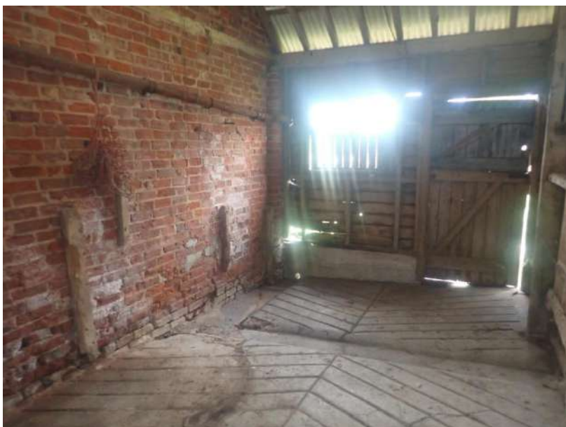
Plate 77: General view of the interior of Cell 2, from the east
