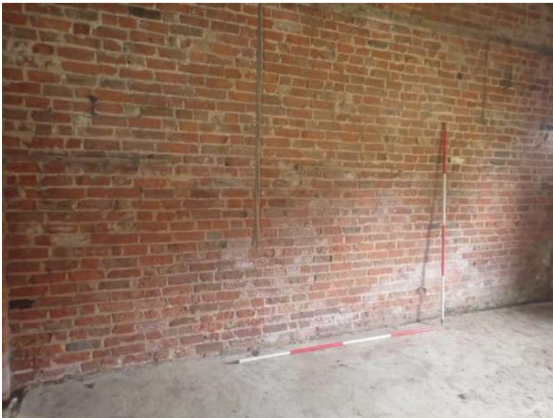
Plate 298: View of the south wall of Cell 7, from the north-east
