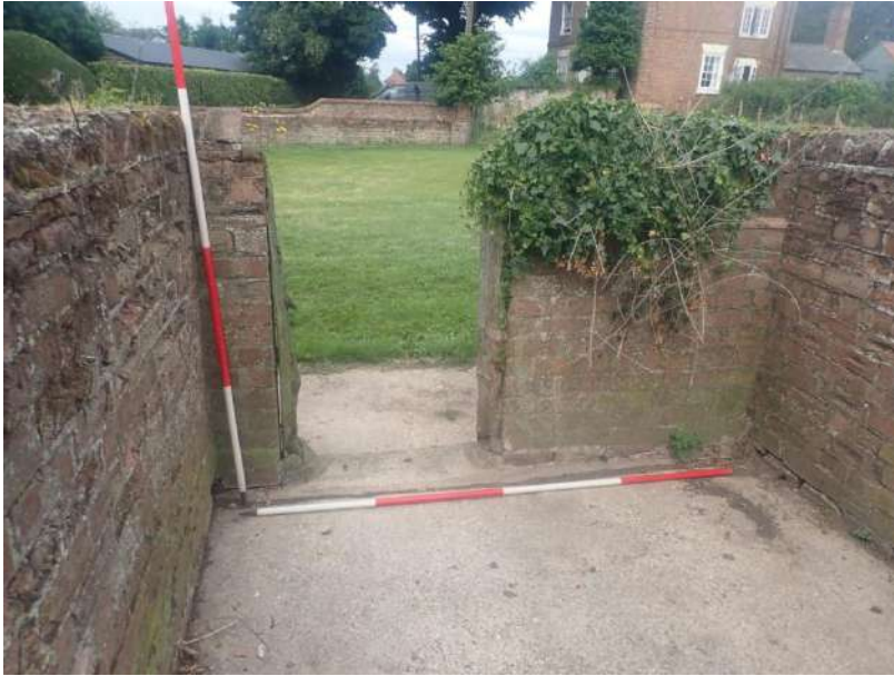
Plate 276: View of the western yard wall of the second sty, from the east
