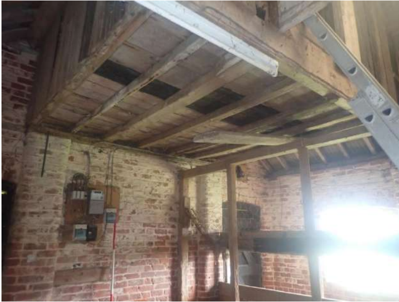
Plate 186: View of the west wall of Cell 6, from the south-east
