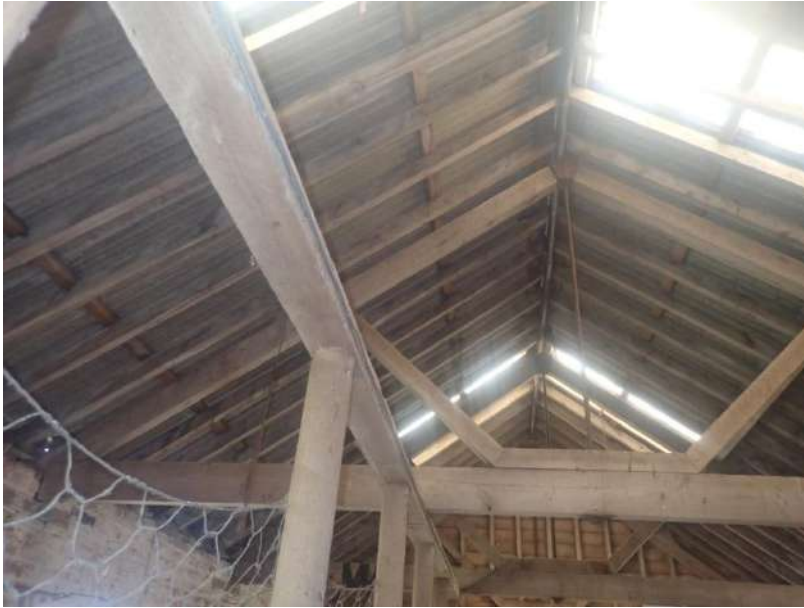
Plate 219: View of the roof supporting structure of Cell 6, from the west
