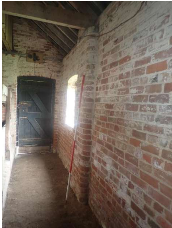
Plate 249: View of the north wall of Cell 6, from the east
