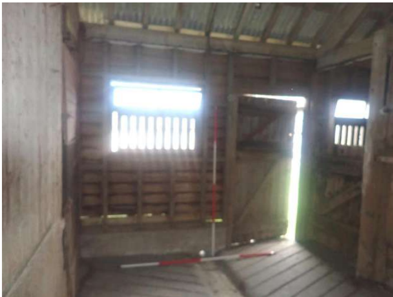
Plate 64: View of the west wall of Cell 1, from the east
