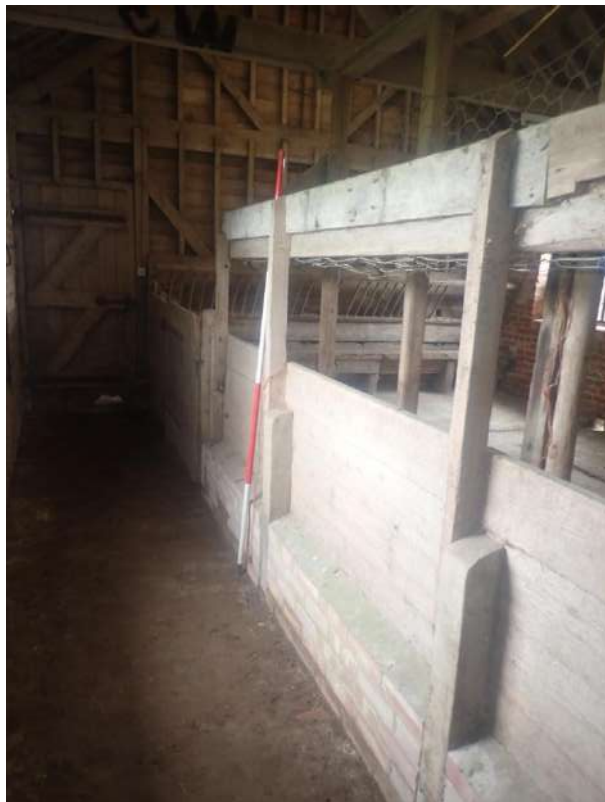
Plate 242: View of the timber fence along the southern side of the northern passageway of Cell 6, from the west
