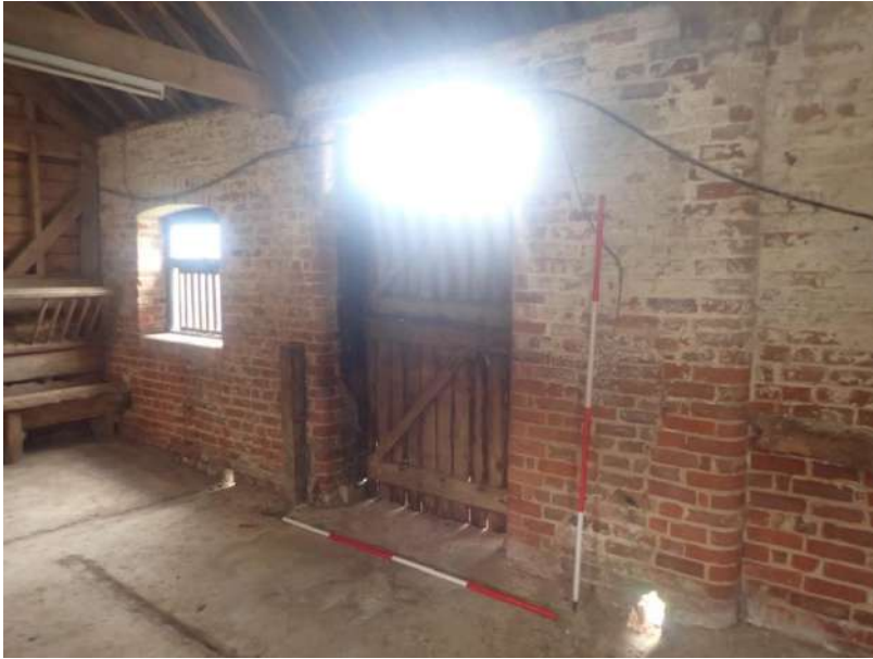
Plate 194: View of the south wall of Cell 6, from the north-west
