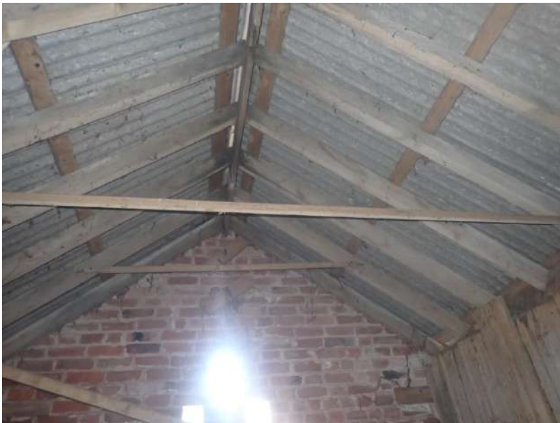
Plate 203: View of the interior of the former dovecote, from the east
