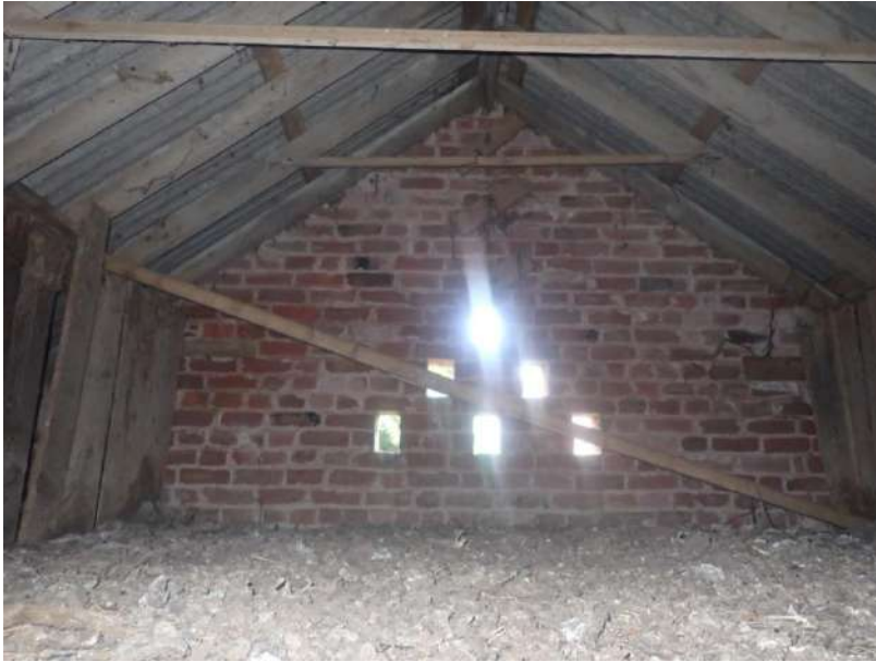
Plate 200: View of the interior of the former dovecote, from the east
