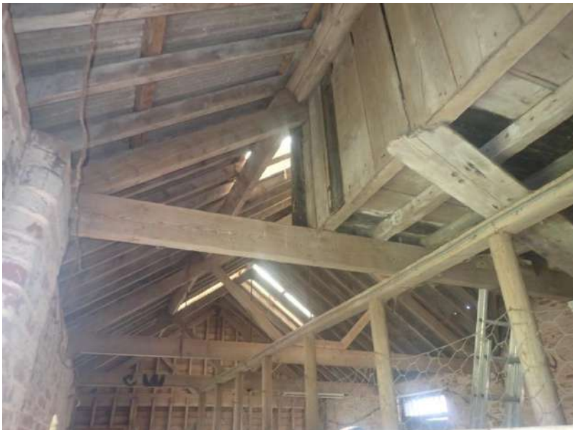
Plate 236: View of the roof supporting structure of Cell 6, from the west
