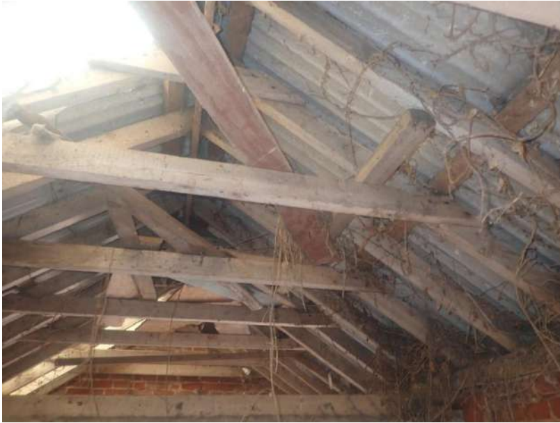
Plate 313: View of the roof supporting structure of Sties 2-3, from the north
