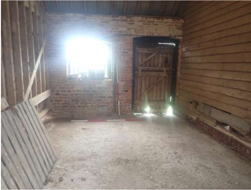
Plate 156: General view of the interior of Cell 5, from the north
