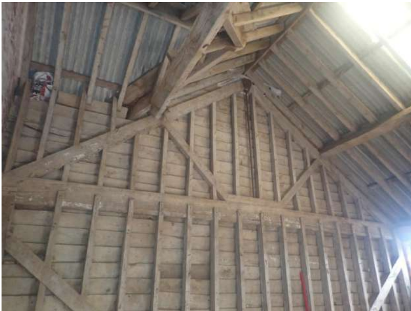
Plate 127: View of the west wall of Cell 3, from the east
