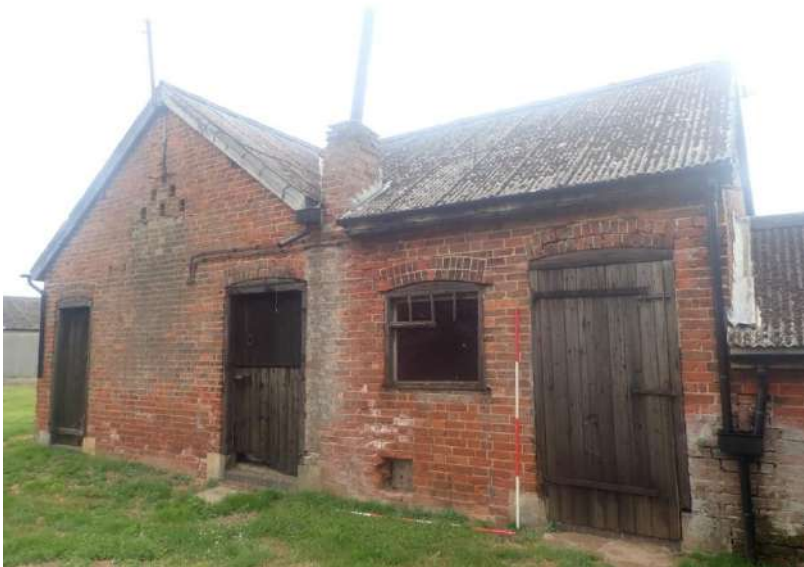
Plate 259: View of the West Elevation of Outbuilding 2, from the west
