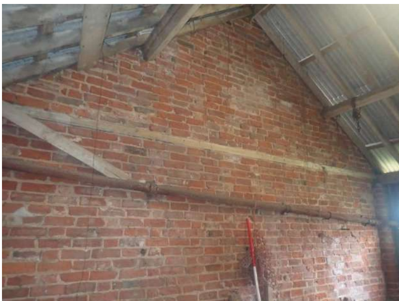
Plate 93: View of the south wall of Cell 2, from the north-east
