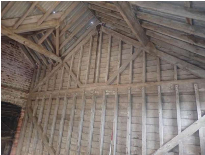
Plate 129: View of the west wall of Cell 3, from the east
