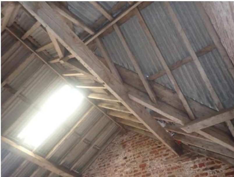
Plate119: View of the roof supporting structure of Cell 3, from the west
