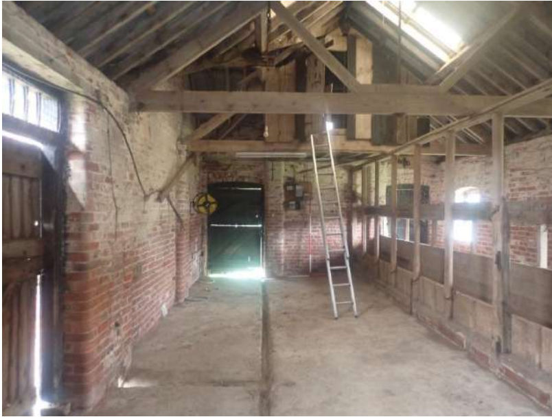
Plate 178: General view of the interior of Cell 6, from the east
