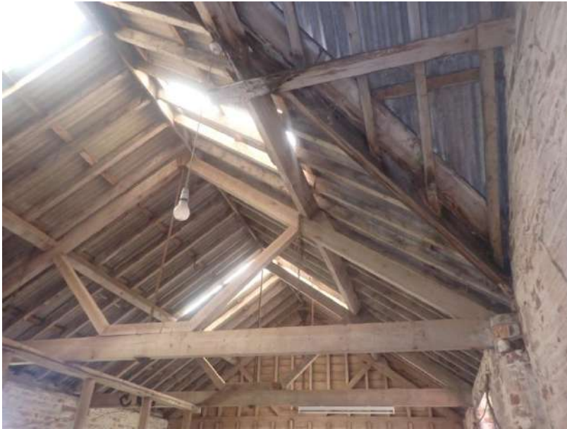
Plate 215: View of the roof supporting structure of Cell 6, from the west
