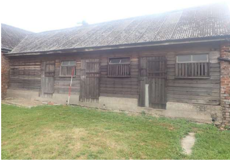
Plate 31: View of the West Elevation of Outbuilding 1, from the south-west
