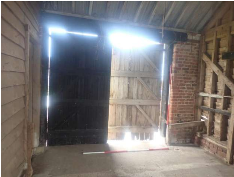
Plate 169: View of the north wall of Cell 5, from the south
