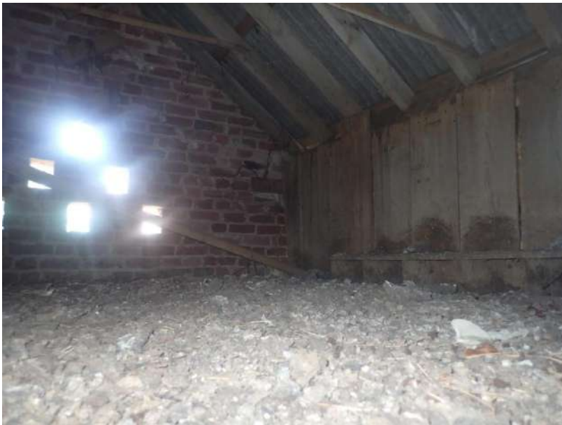
Plate 201: View of the interior of the former dovecote, from the east
