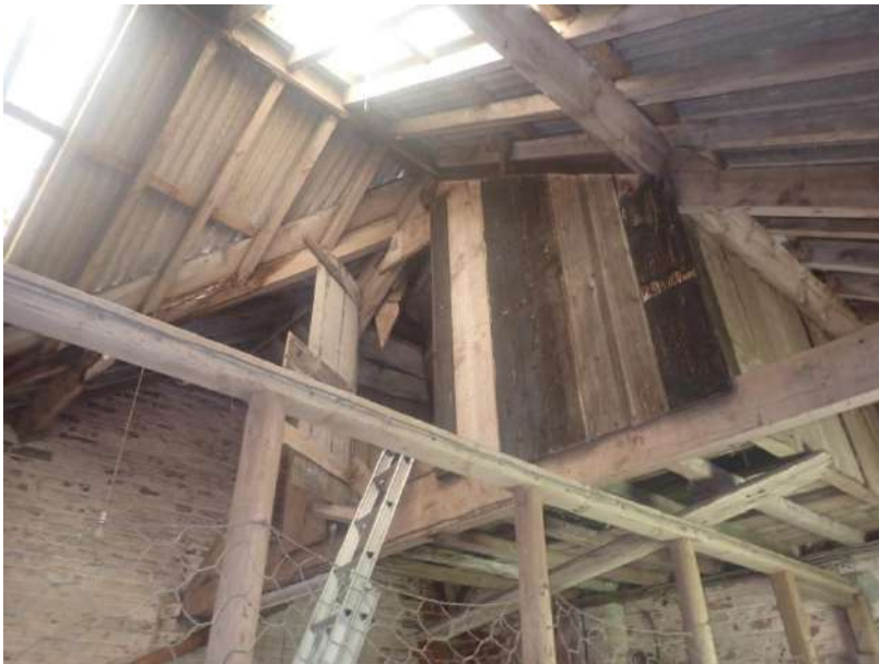
Plate 228: View of the roof supporting structure of Cell 6, from the north-west
