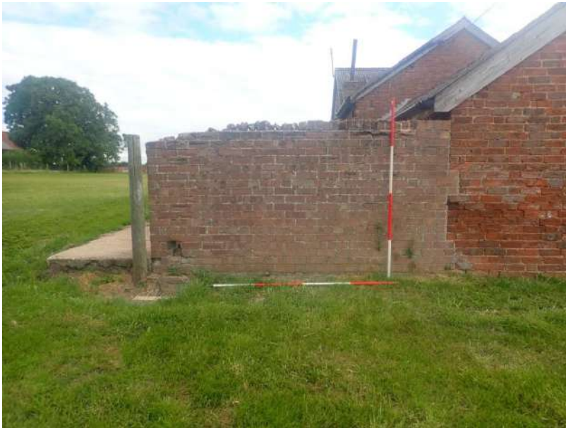
Plate 267: View of the southern boundary wall of the piggery, from the south
