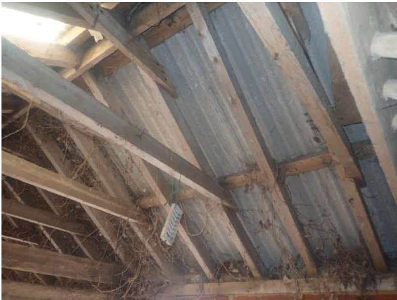
Plate 308: View of the roof supporting structure of Sties 1-3, from the north
