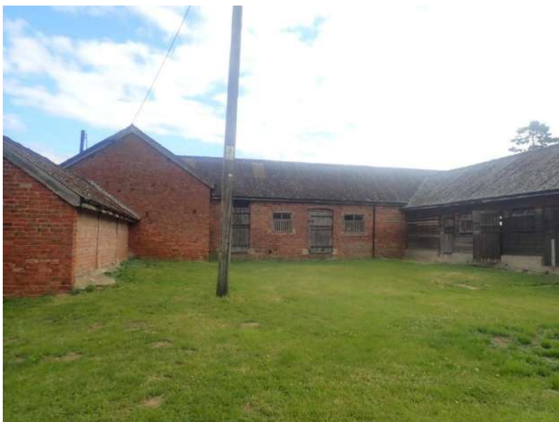
Plate 5: General view of the outbuilding complex, from the south
