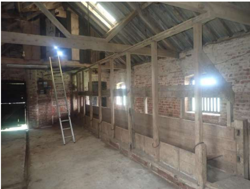
Plate 179: General view of the interior of Cell 6, from the east
