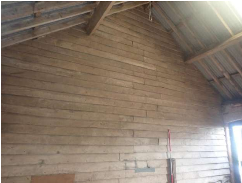
Plate 153: View of the west wall of Cell 4, from the east
