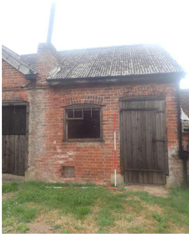
Plate 260: View of the West Elevation of Outbuilding 2, from the west
