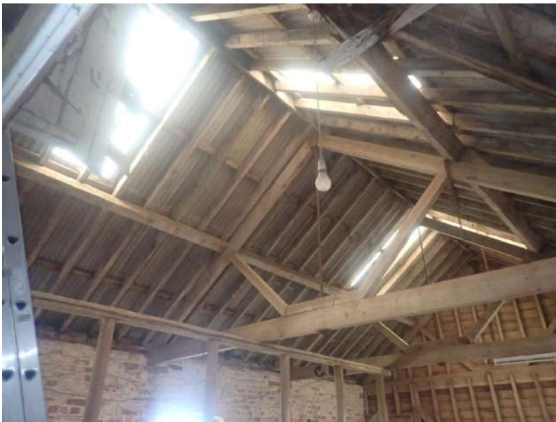
Plate 216: View of the roof supporting structure of Cell 6, from the west
