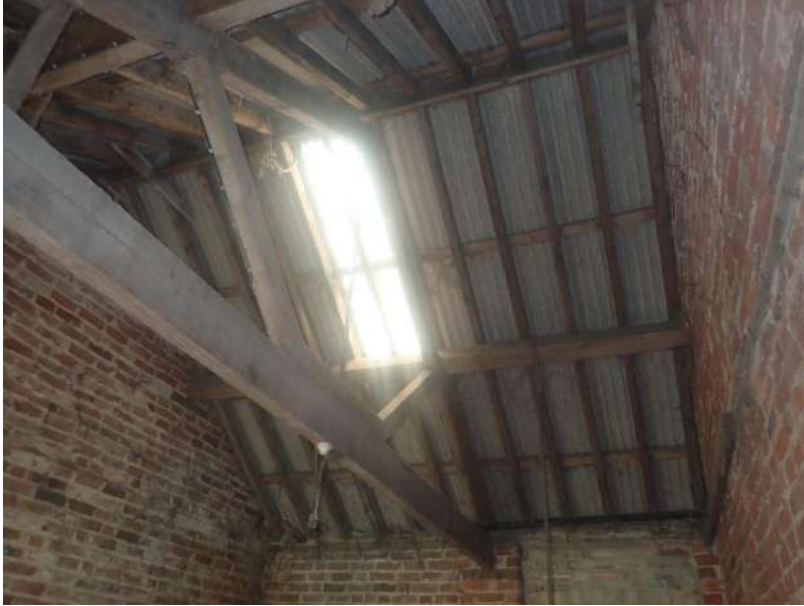
Plate 292: View of the roof supporting structure of Cell 7, from the west
