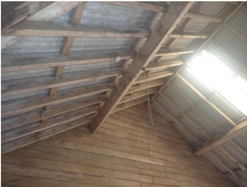
Plate 139: View of the roof supporting structure of Cell 4, from the east
