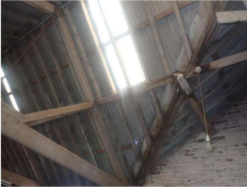
Plate 221: View of the roof supporting structure of Cell 6, from the north-west
