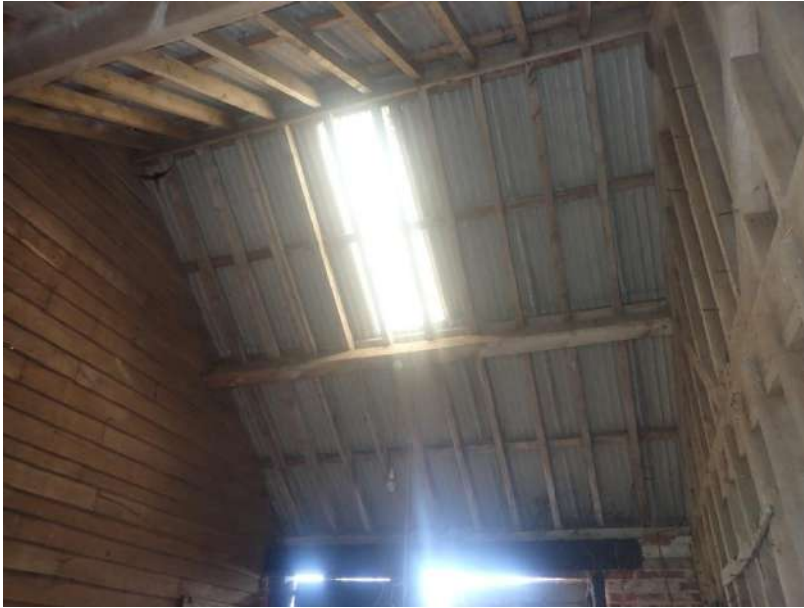
Plate 162: View of the roof supporting structure of Cell 5, from the south
