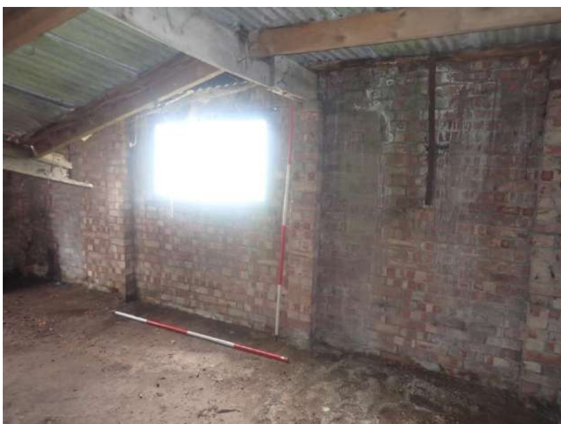
Plate 24: View of the south wall of the modern lean-to/garage, from the north-west
