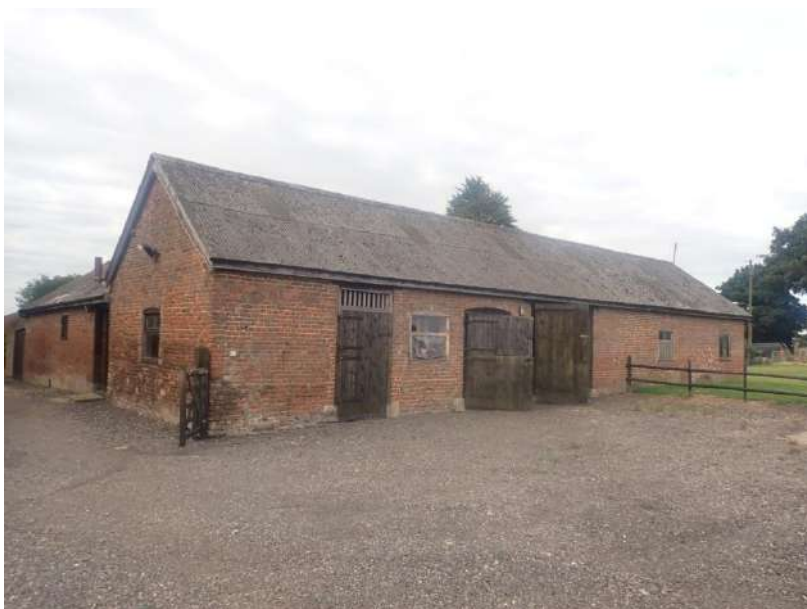
Plate 7: General view of the outbuilding complex, from the north-east
