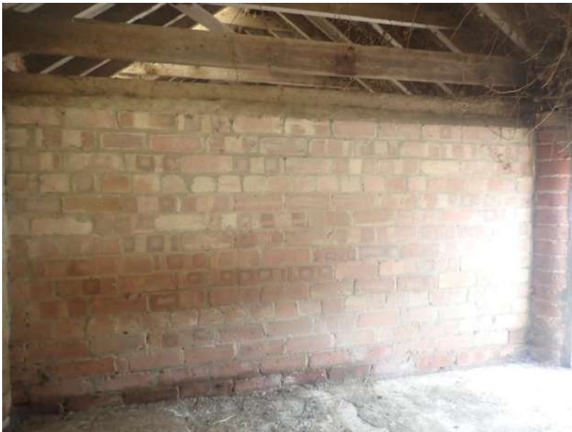
Plate 306: View of the south wall of Stie 1, from the north
