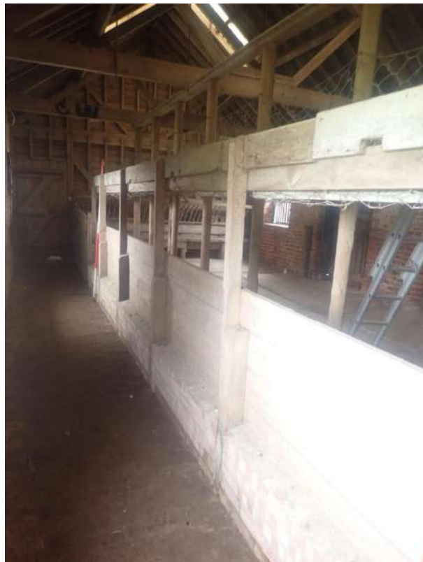
Plate 240: View of the timber fence along the southern side of the northern passageway of Cell 6, from the west
