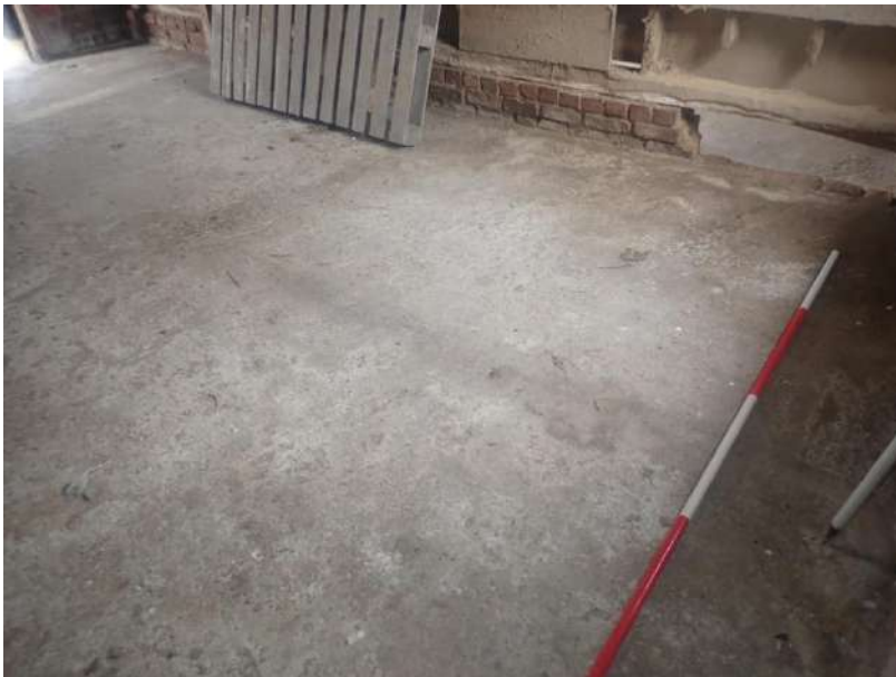
Plate 159: View of the flooring of Cell 5, from the south-west
