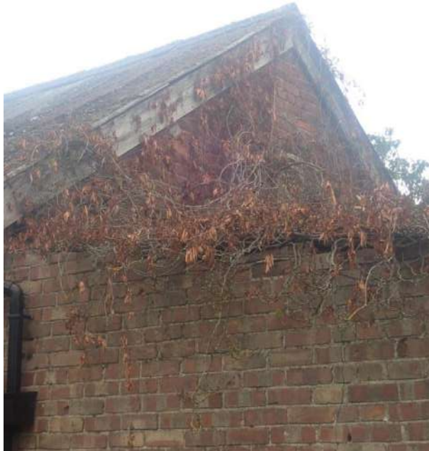
Plate 33: View of the South Elevation of Outbuilding 1, from the south-west
