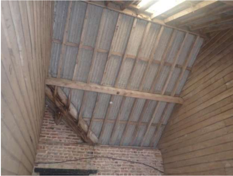
Plate 140: View of the roof supporting structure of Cell 4, from the north
