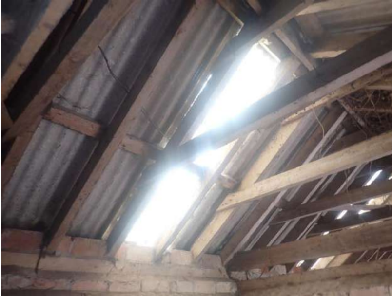
Plate 309: View of the roof supporting structure of Sties 1-3, from the north
