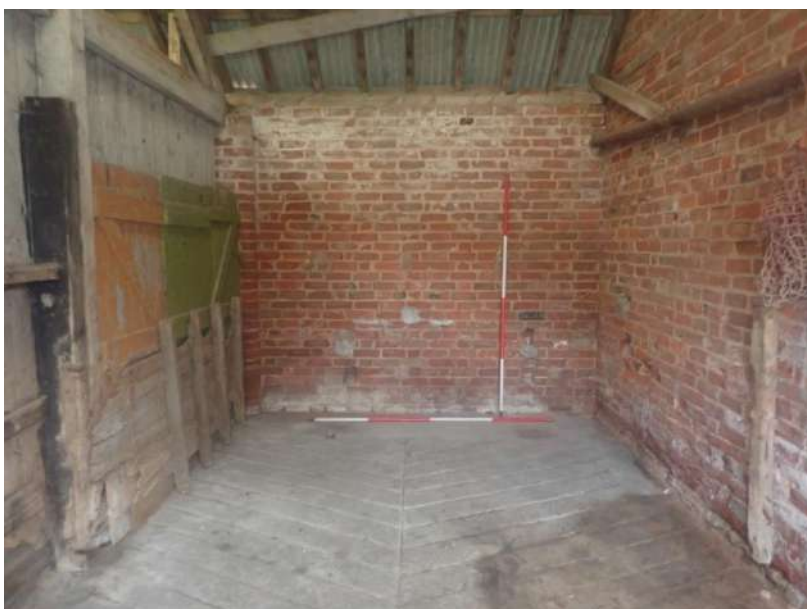
Plate 76: General view of the interior of Cell 2, from the west
