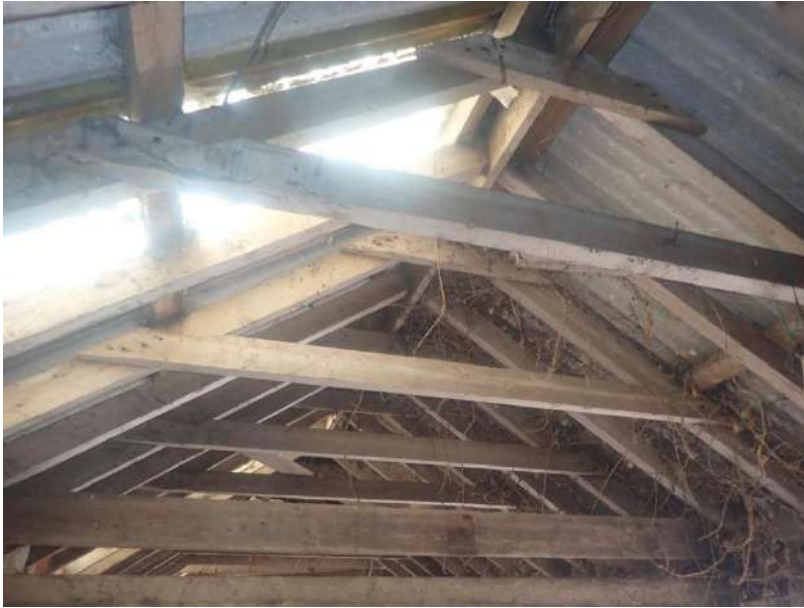
Plate 307: View of the roof supporting structure of Sties 1-3, from the north
