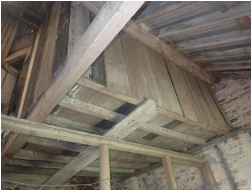
Plate 230: View of the former dovescote attached to the west wall of Cell 6, from the north
