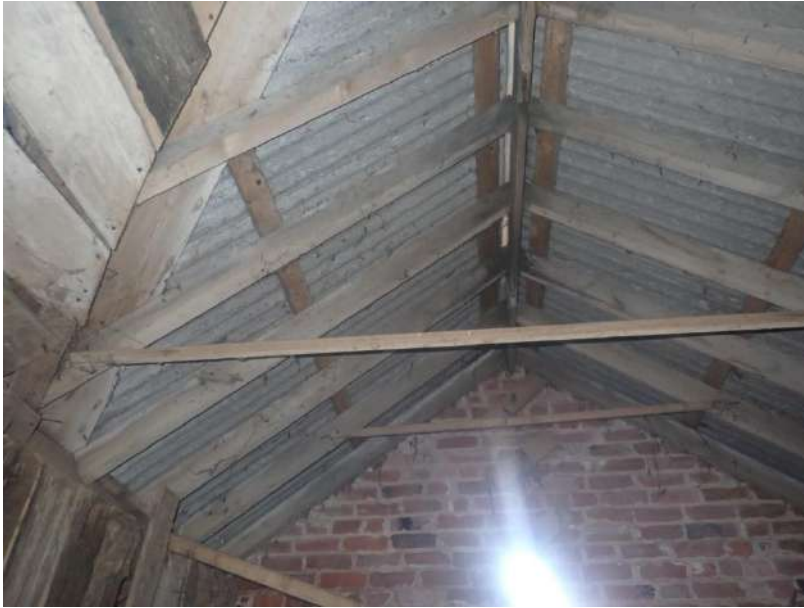
Plate 202: View of the interior of the former dovecote, from the east
