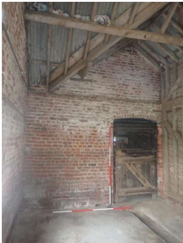
Plate 125: View of the south wall of Cell 3, from the north
