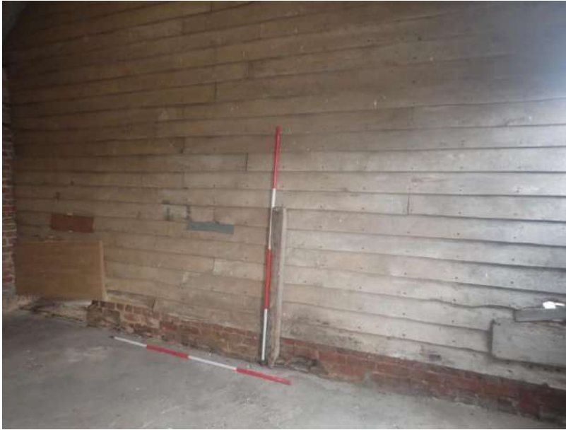
Plate 154: View of the west wall of Cell 4, from the east
