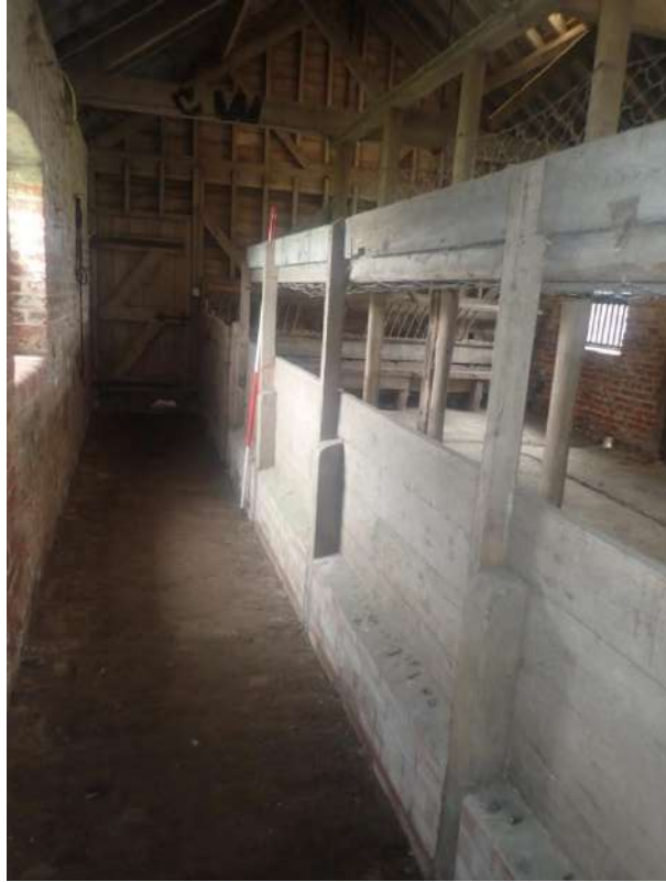
Plate 241: View of the timber fence along the southern side of the northern passageway of Cell 6, from the west
