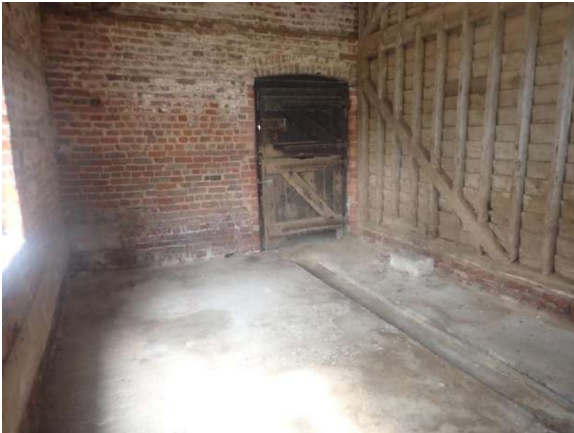
Plate 110: General view of the interior of Cell 3, from the north
