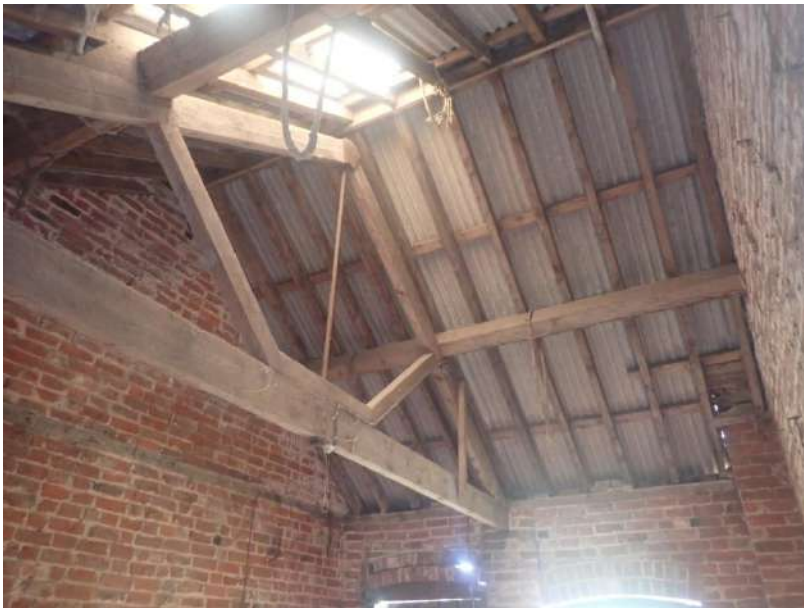
Plate 289: View of the roof supporting structure of Cell 7, from the east
