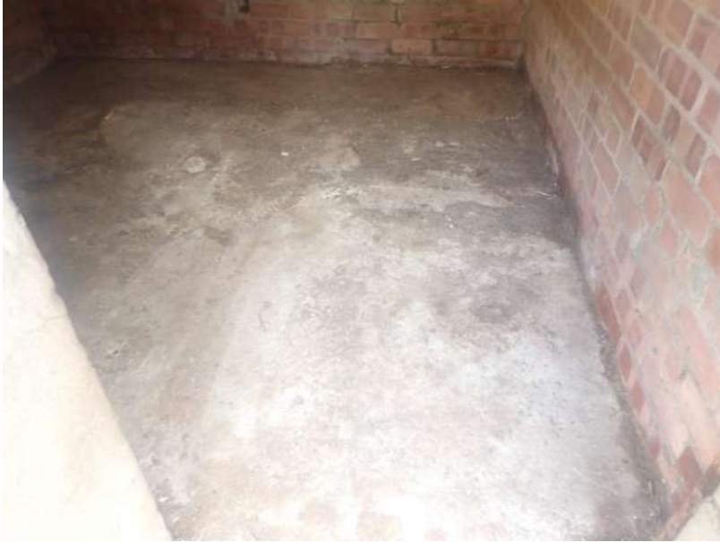
Plate 317: View of the flooring of Stie 2, from the west
