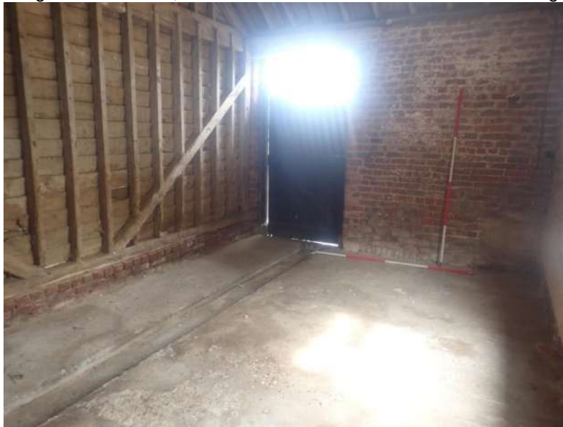
Plate 109: General view of the interior of Cell 3, from the south
