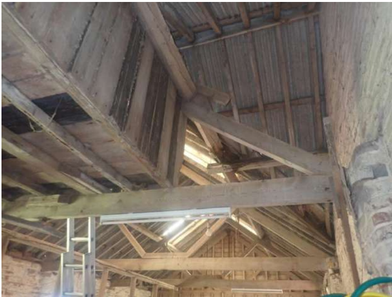
Plate 214: View of the roof supporting structure of Cell 6, from the west
