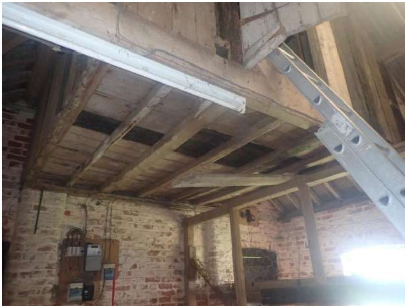
Plate 189: View of the former dovecote attached to the west wall of Cell 6, from the east
