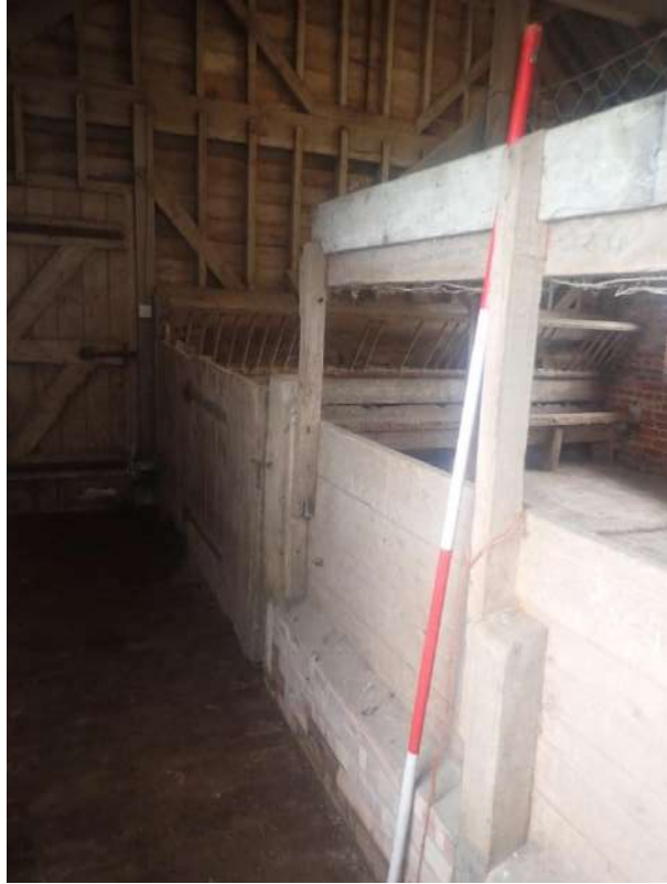
Plate 243: View of the timber fence along the southern side of the northern passageway of Cell 6, from the west
