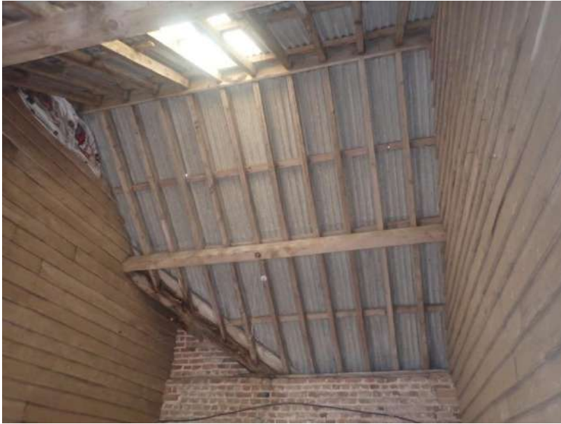
Plate 142: View of the roof supporting structure of Cell 4, from the north
