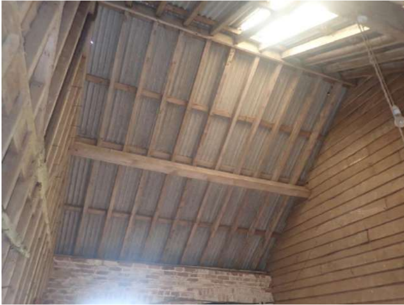
Plate 164: View of the roof supporting structure of Cell 5, from the north
