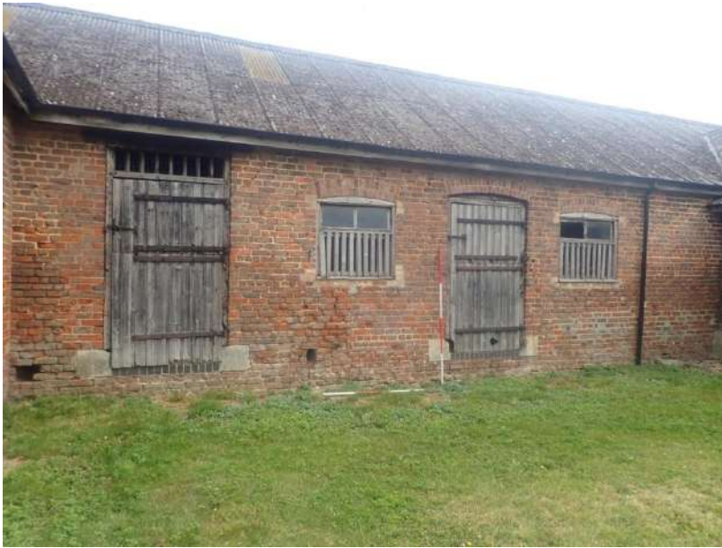
Plate 107: View of the South Elevation of the North Range, from the south
