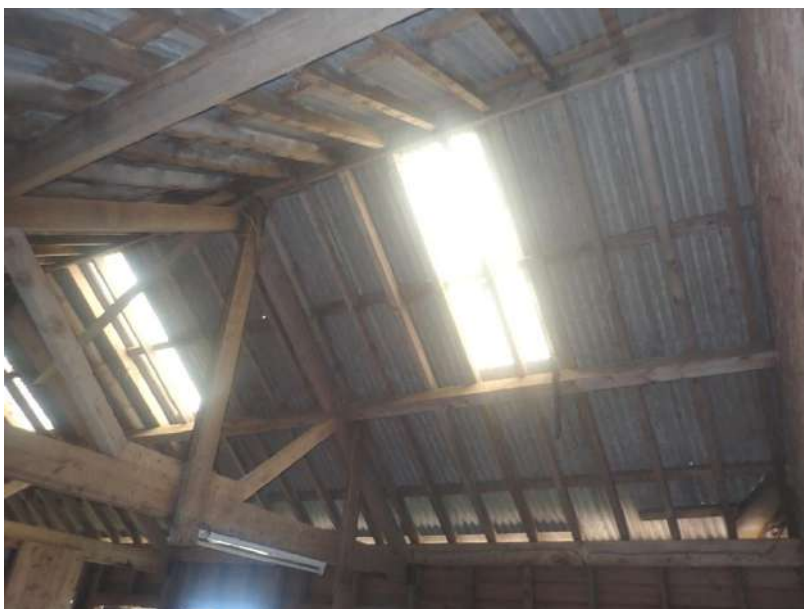
Plate 73: View of the roof supporting structure of Cell 1, from the east
