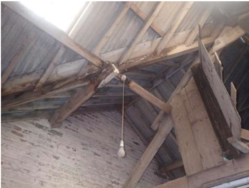
Plate 222: View of the roof supporting structure of Cell 6, from the north-east
