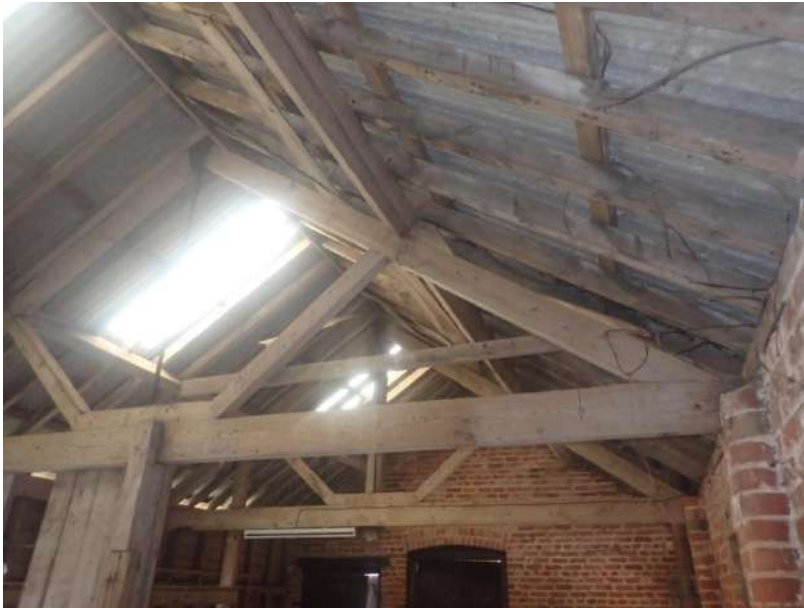
Plate 65: View of the roof supporting structure of Cell 1, from the south
