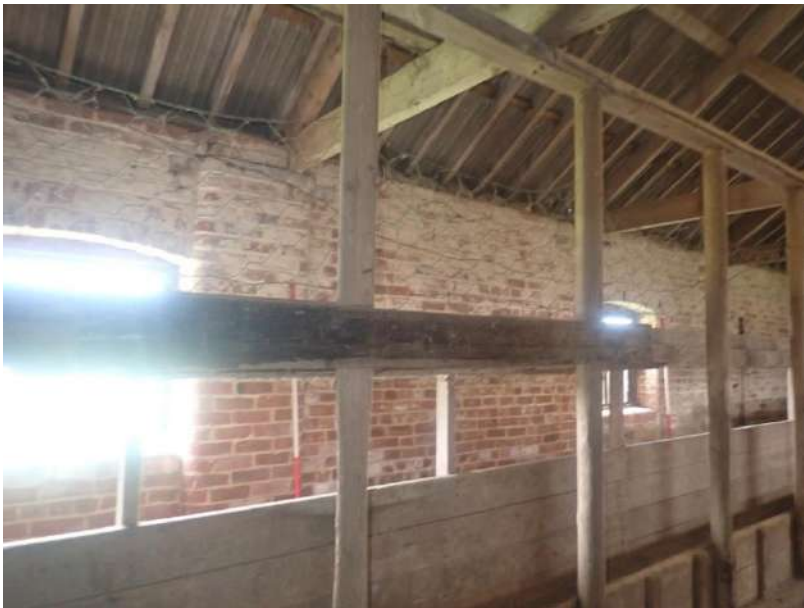
Plate 257: View of the north wall of Cell 6, from the south
