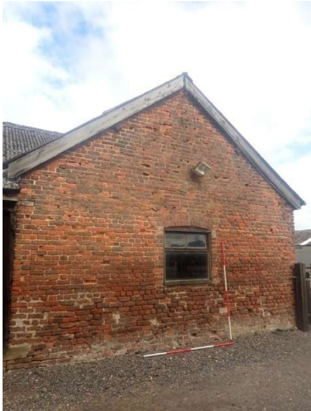
Plate 97: View of the East Elevation of the North Range, from the east
