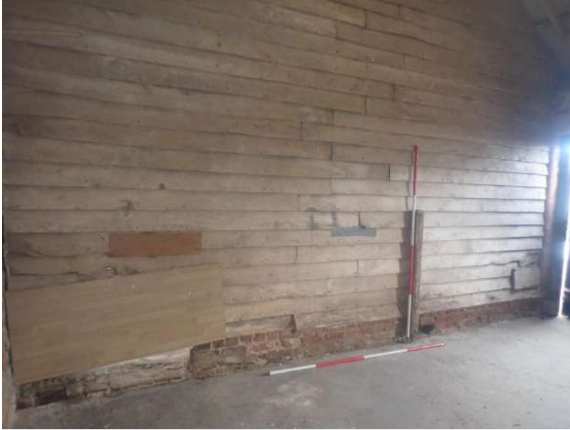
Plate 152: View of the west wall of Cell 4, from the east
