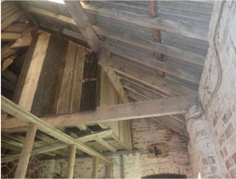
Plate 227: View of the roof supporting structure of Cell 6, from the east
