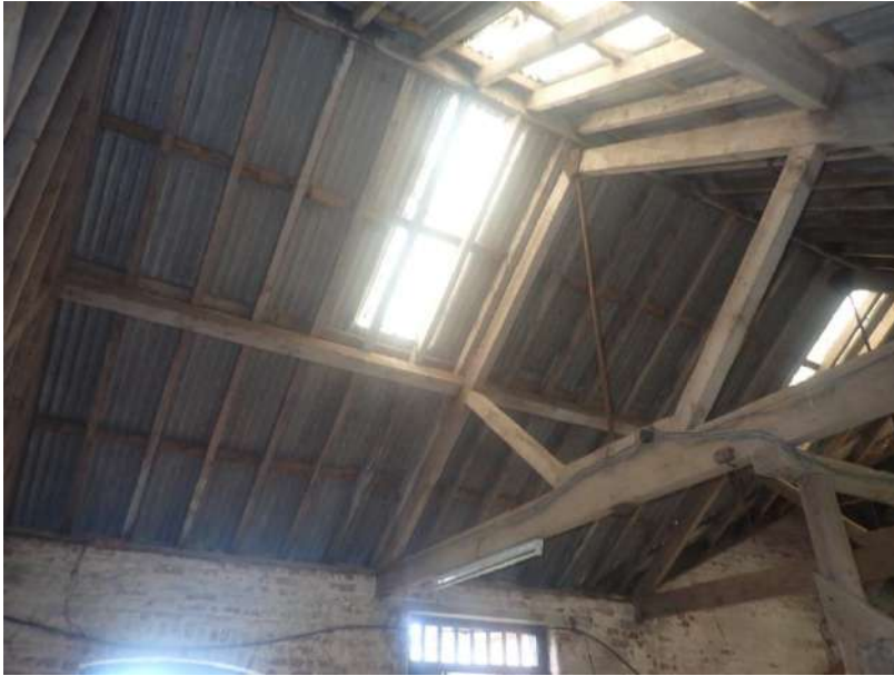
Plate 225: View of the roof supporting structure of Cell 6, from the north-east
