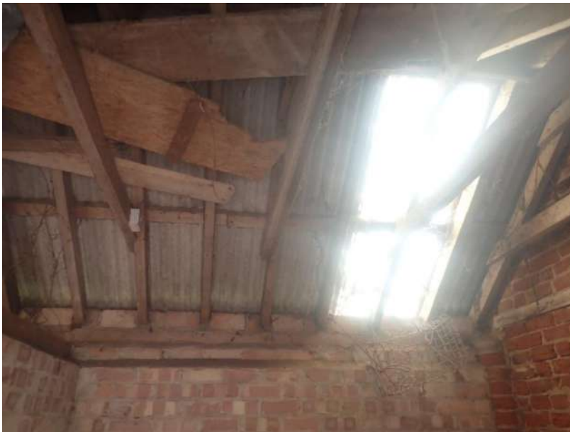
Plate 320: View of the roof supporting structure above Stie 3, from the west
