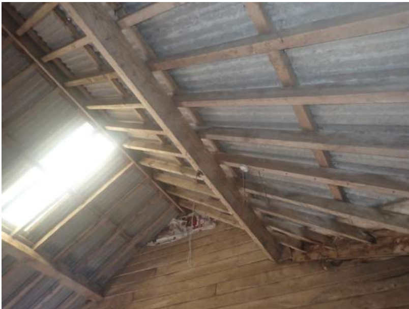
Plate 145: View of the roof supporting structure of Cell 4 , from the west
