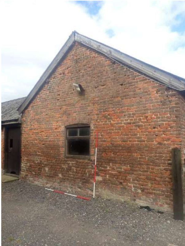
Plate 98: View of the East Elevation of the North Range, from the north-east
