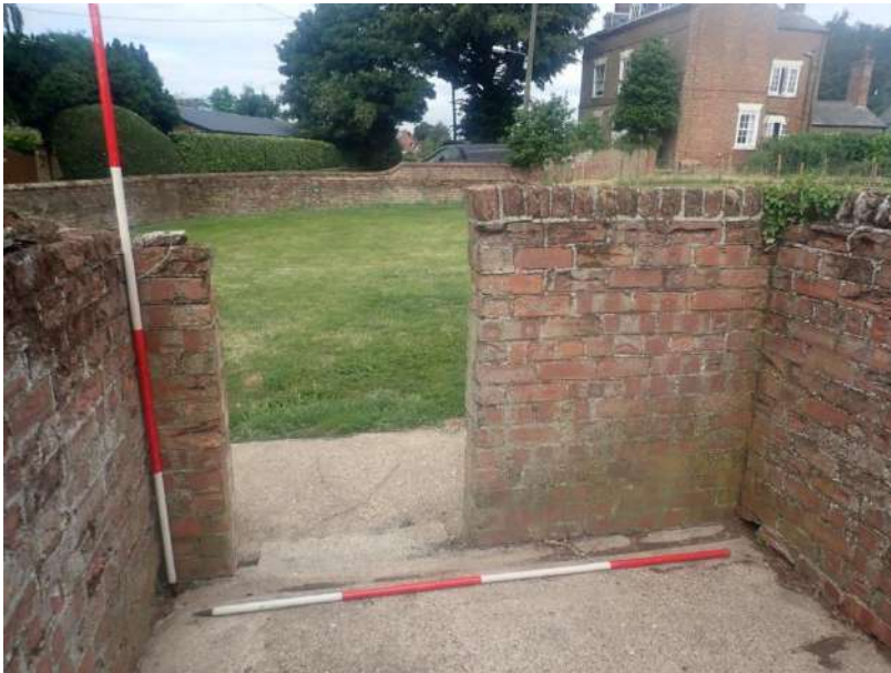
Plate 281: View of the western yard wall of the third sty, from the east
