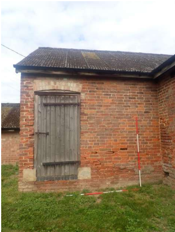
Plate 263: View of the East Elevation of Outbuilding 2, from the east
