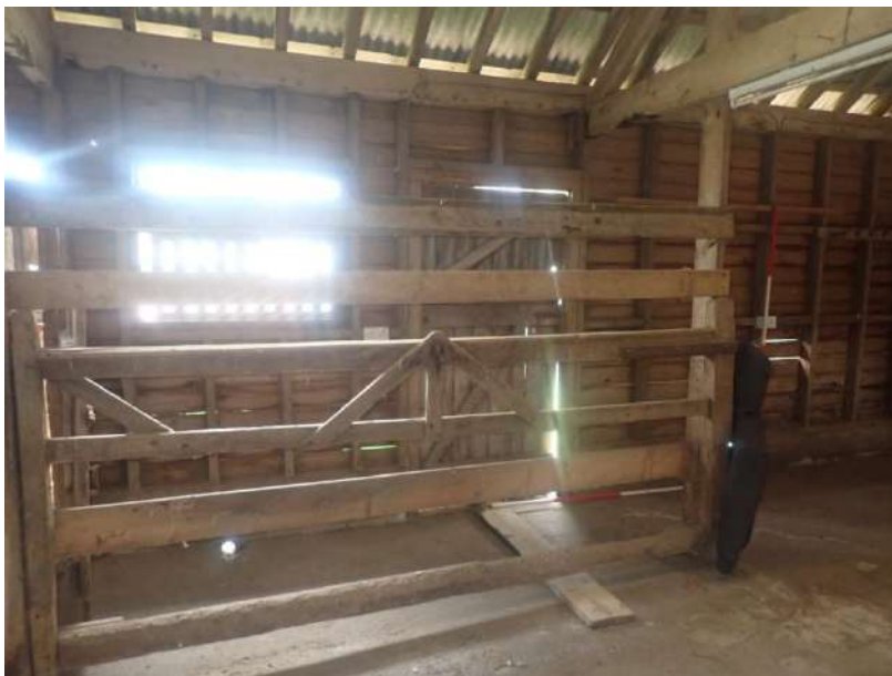
Plate 60: View of the west wall of Cell 1, from the east
