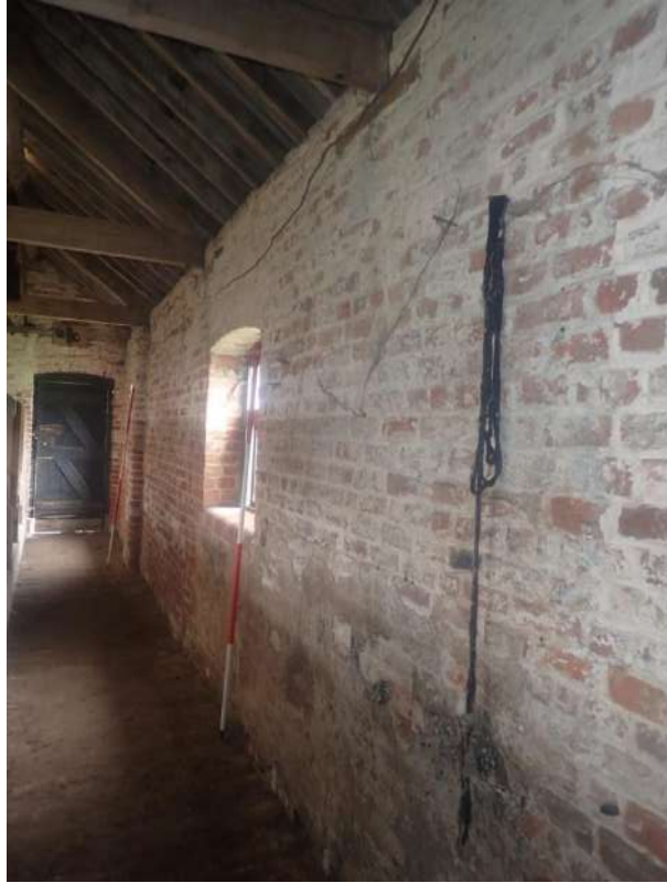
Plate 246: View of the north wall of Cell 6, from the east
