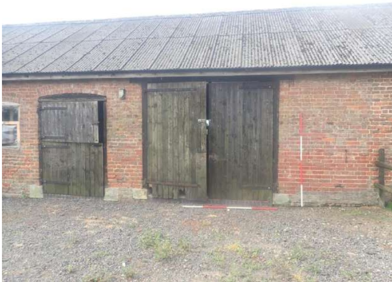
Plate 101: View of the North Elevation of the North Range, from the north
