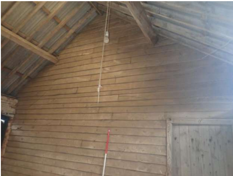
Plate 177: View of the west wall of Cell 5, from the east
