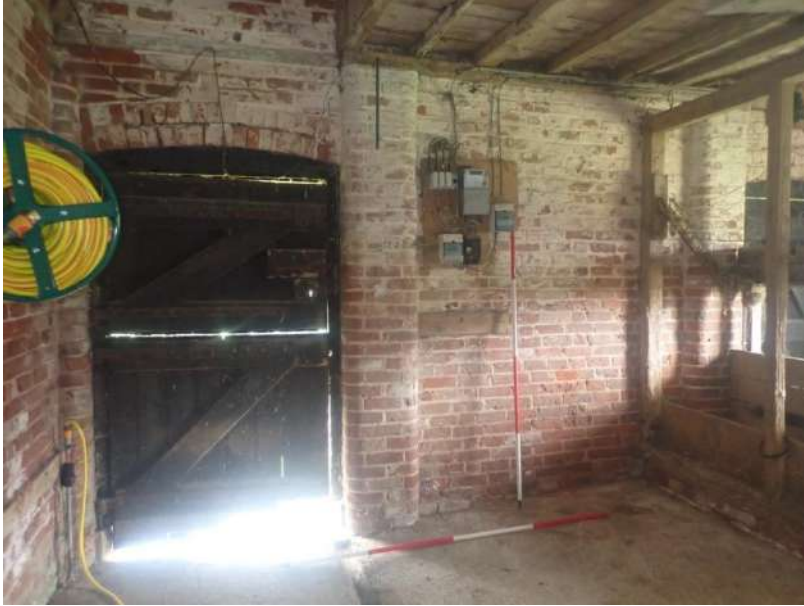
Plate 184: View of the west wall of Cell 6, from the east
