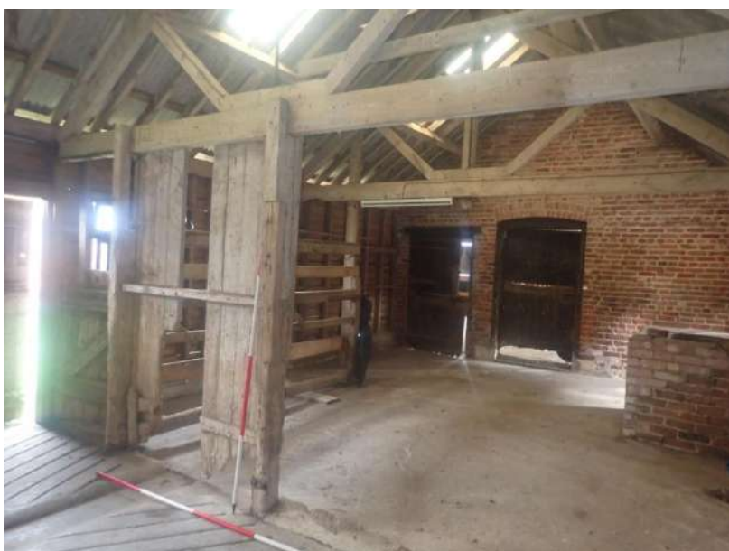
Plate 48: View of the internal timber partition within Cell 1, from the south-east
