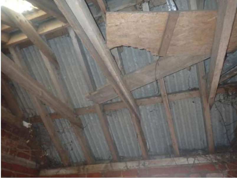
Plate 323: View of the roof supporting structure above Stie 3, from the east
