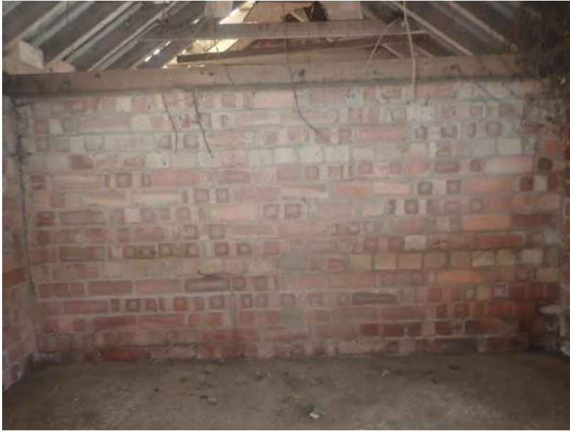
Plate 311: View of the south wall of Stie 2, from the north
