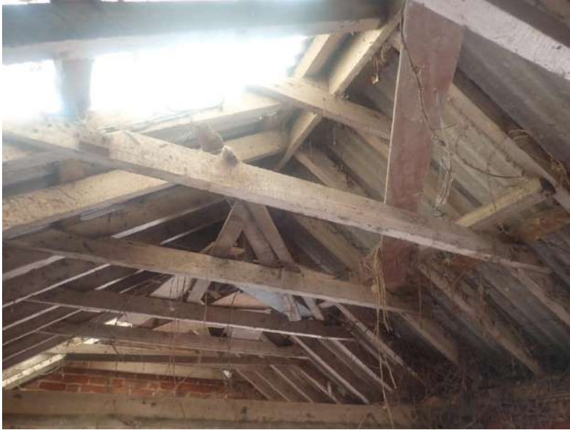
Plate 315: View of the roof supporting structure of Sties 1-2, from the south
