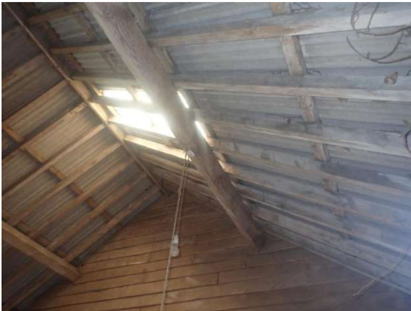
Plate 165: View of the roof supporting structure of Cell 5, from the east
