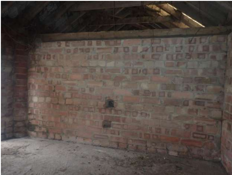
Plate 327: View of the north wall of Stie 3, from the south
