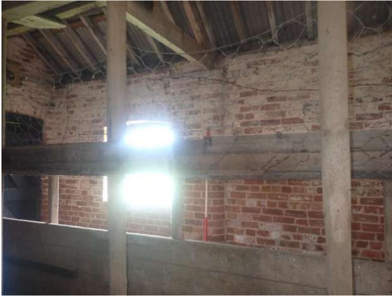
Plate 258: View of the north wall of Cell 6, from the south
