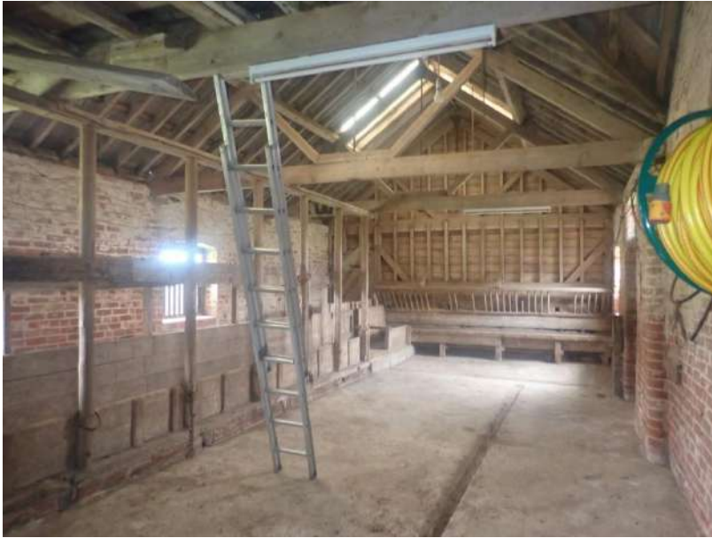
Plate 180: General view of the interior of Cell 6, from the west
