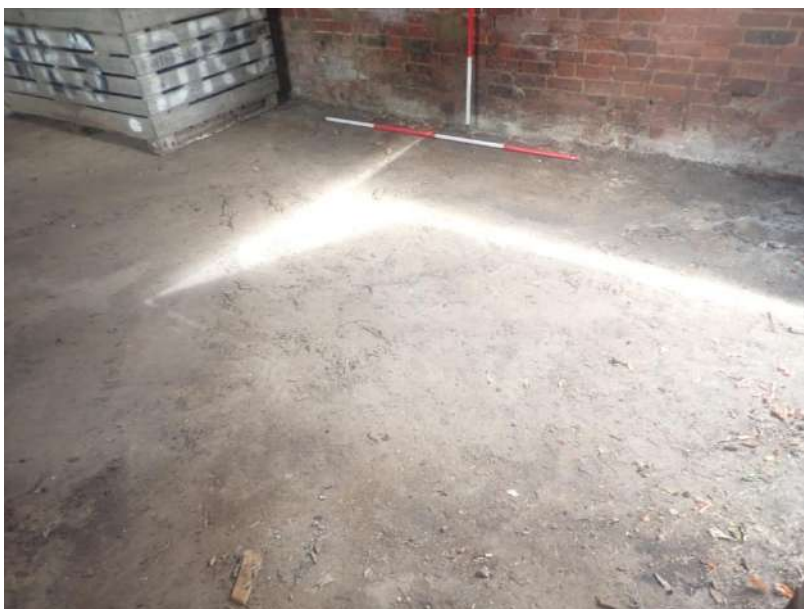
Plate 15: View of the flooring of the modern lean-to/garage, from the south-east
