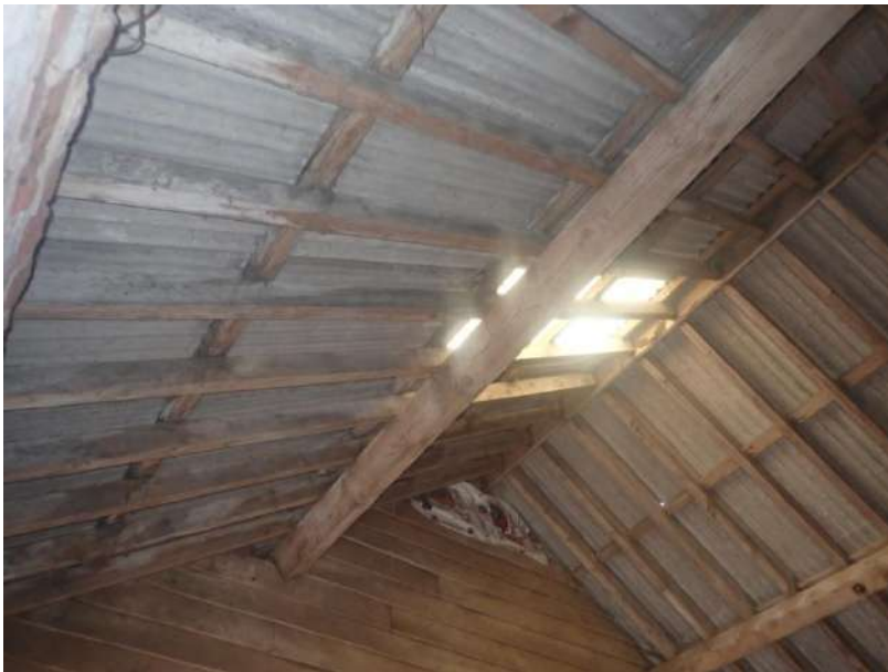
Plate 143: View of the roof supporting structure of Cell 4, from the west
