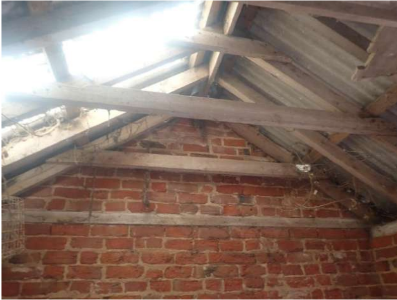
Plate 325: View of the south wall of Stie 3, from the north
