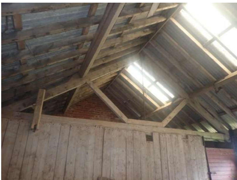
Plate 70: View of the roof supporting structure of Cell 1, from the north
