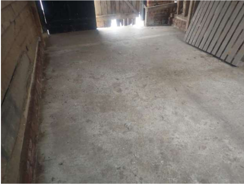
Plate 158: View of the flooring of Cell 5, from the south
