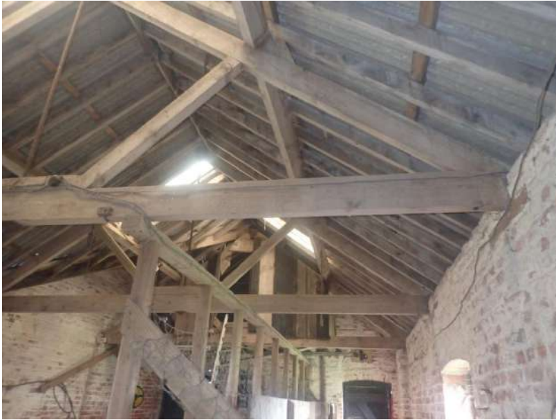
Plate 235: View of the roof supporting structure of Cell 6, from the east
