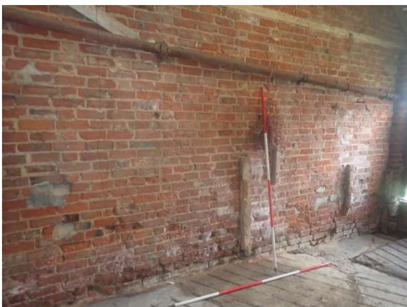
Plate 92: View of the south wall of Cell 2, from the north-east
