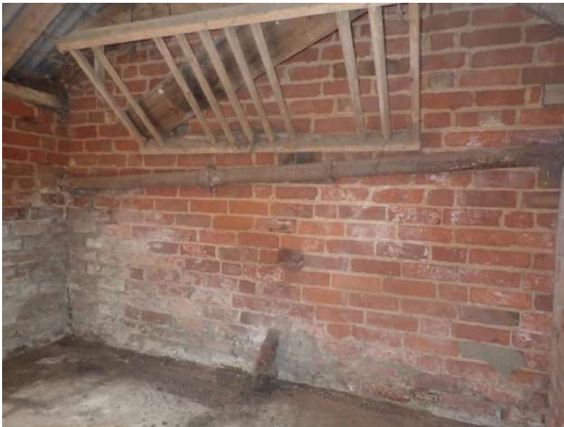
Plate 304: View of the north wall of Stie 1, from the south
