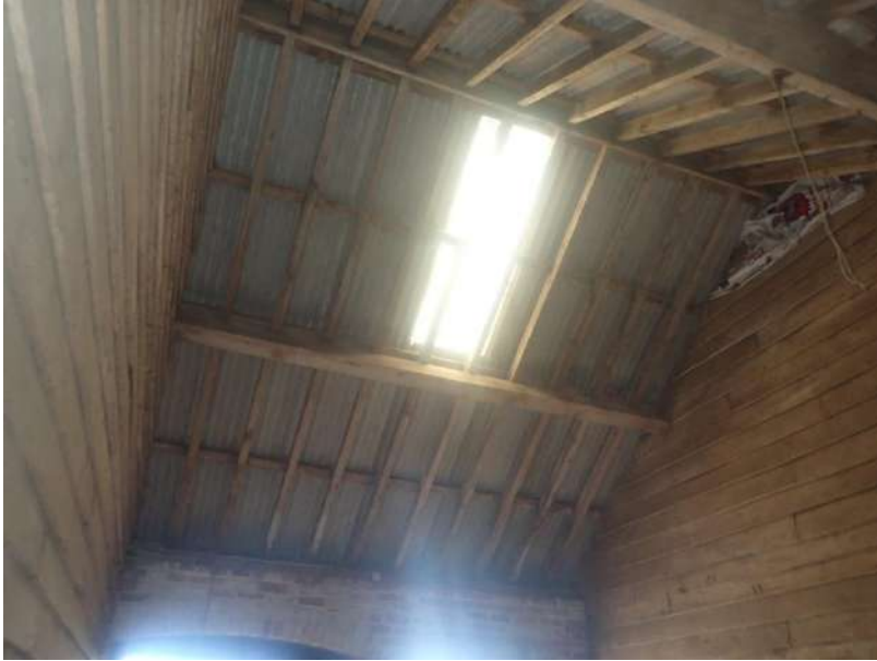
Plate 144: View of the roof supporting structure of Cell 4 , from the south
