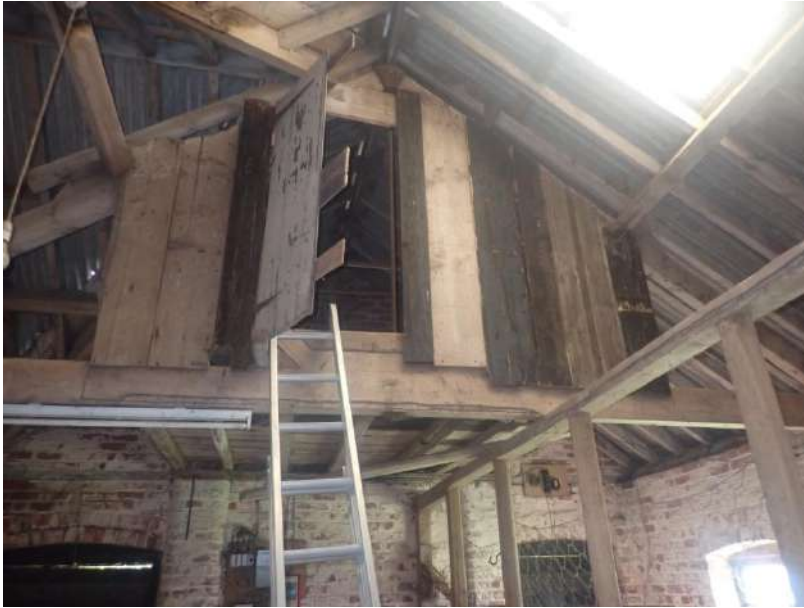
Plate 188: View of the former dovecote attached to the west wall of Cell 6, from the east
