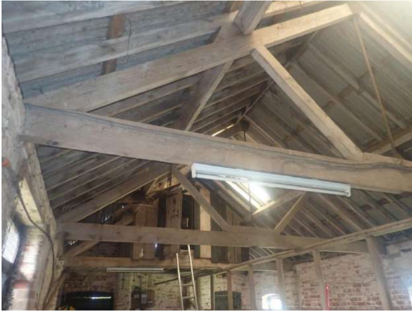
Plate 217: View of the roof supporting structure of Cell 6, from the west
