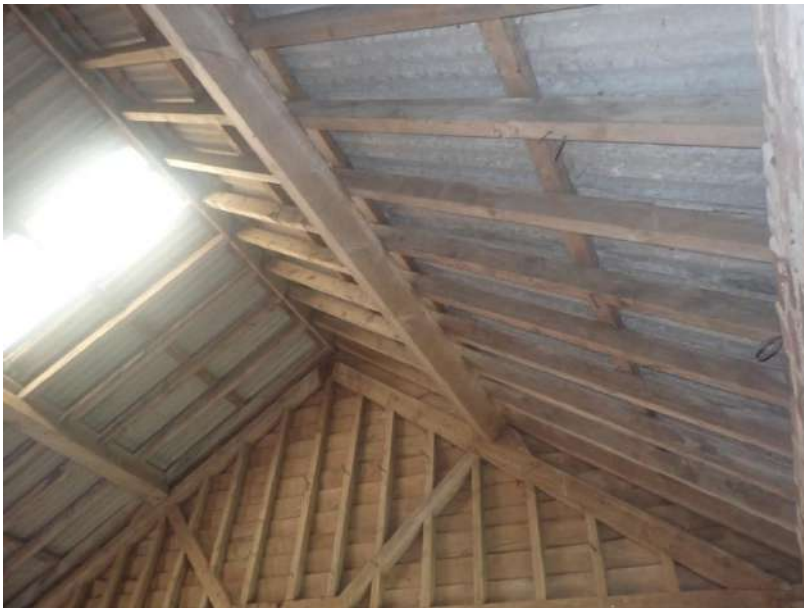
Plate 161: View of the roof supporting structure of Cell 5, from the west
