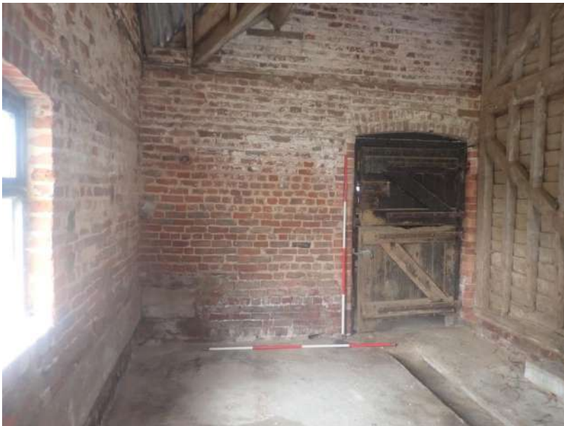
Plate 123: View of the south wall of Cell 3, from the north
