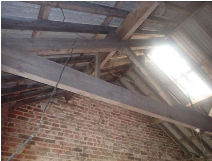
Plate 291: View of the roof supporting structure of Cell 7, from the south
