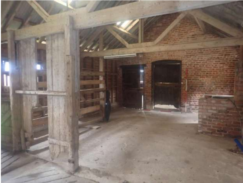
Plate 35: General view of the interior of Cell 1, from the south
