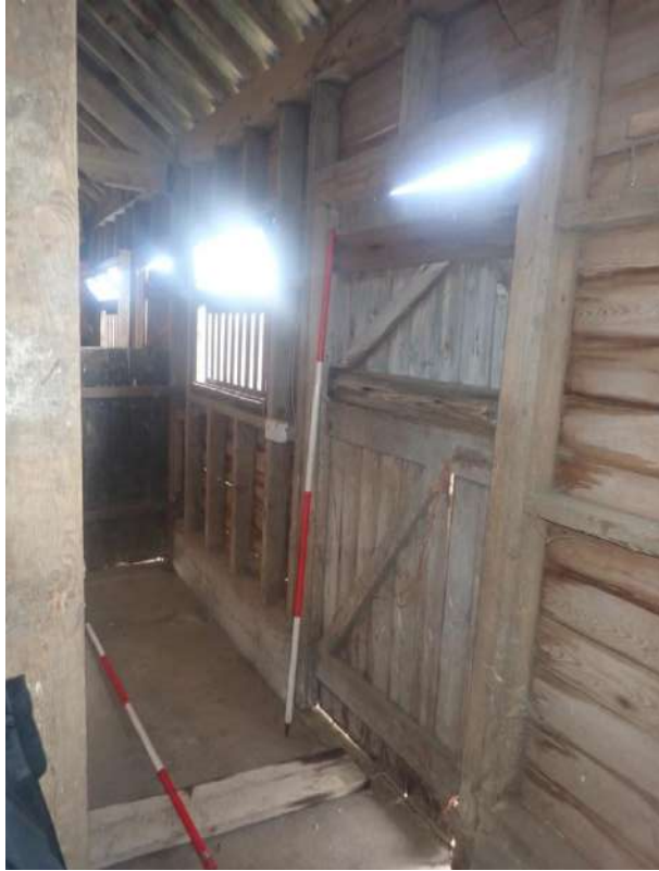
Plate 63: View of the interior of Cell 1, from the north
