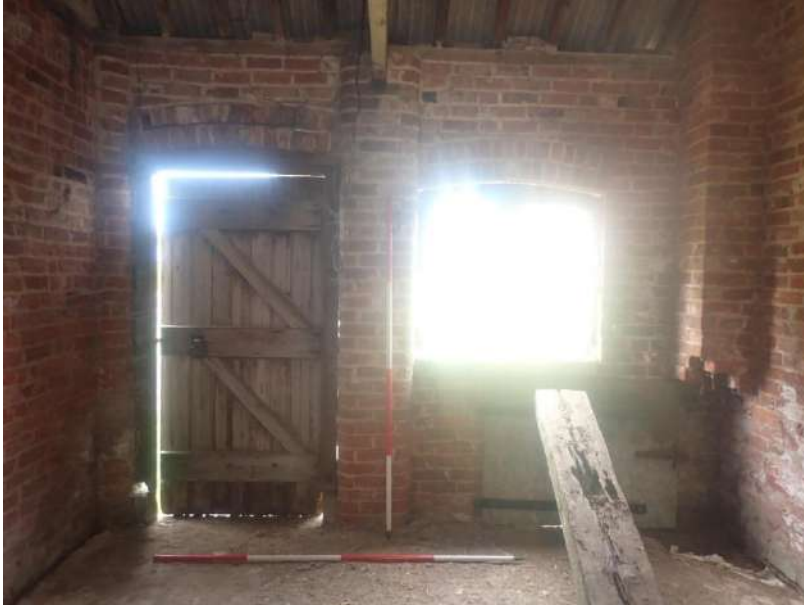
Plate 294: View of the west wall of Cell 7, from the east
