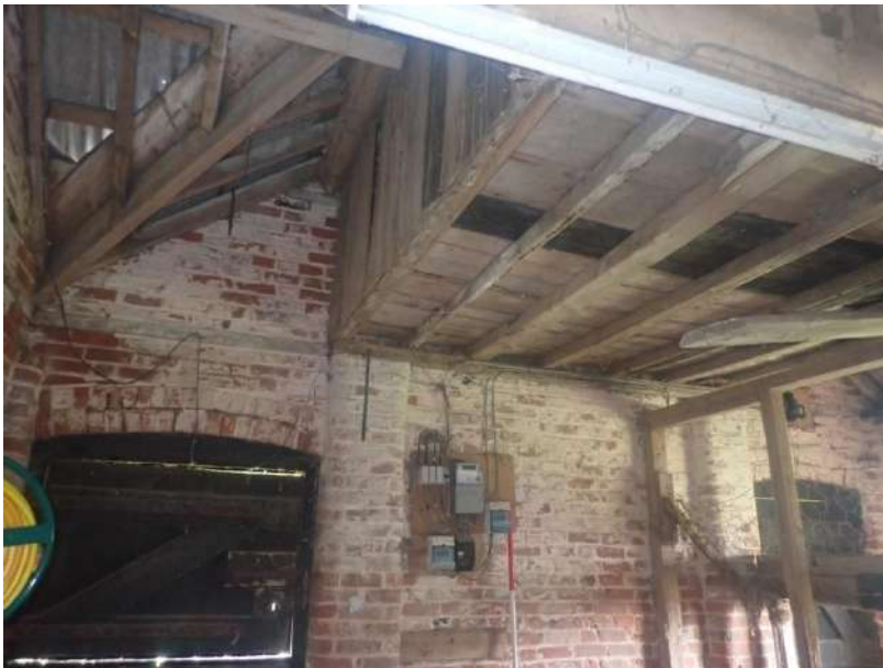
Plate 185: View of the west wall of Cell 6, from the east
