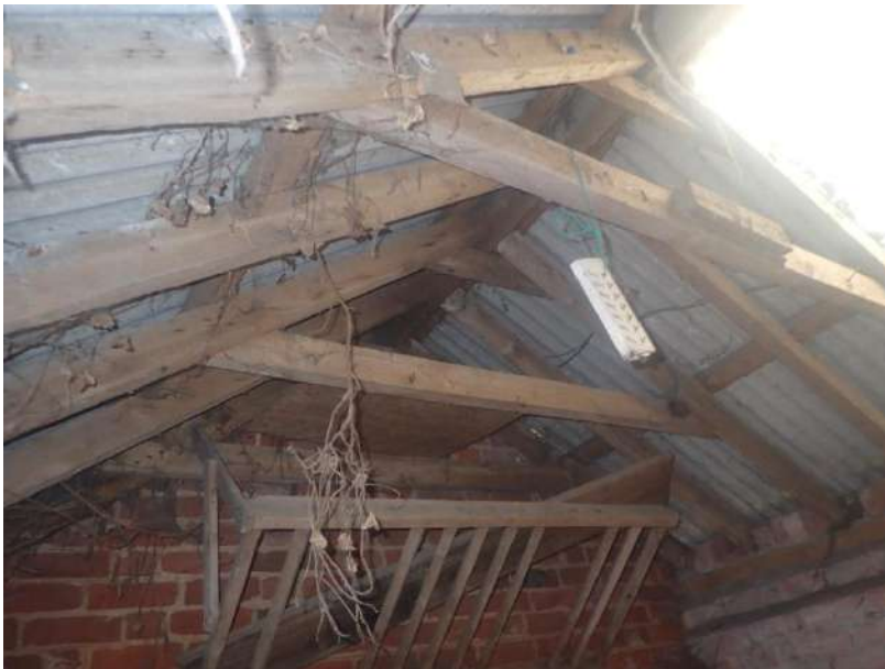
Plate 302: View of the roof supporting structure of Stie 1, from the south
