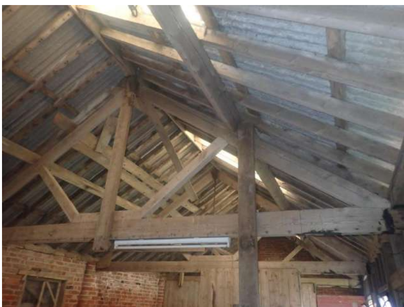
Plate 74: View of the roof supporting structure of Cell 1, from the north
