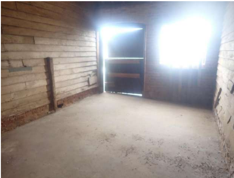
Plate 135: General view of the interior of Cell 4, from the south
