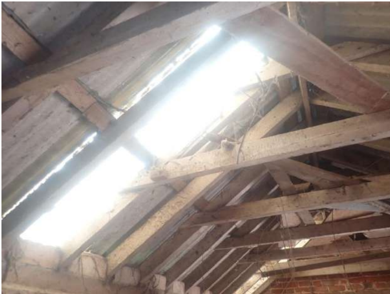
Plate 312: View of the roof supporting structure of Sties 2-3, from the north
