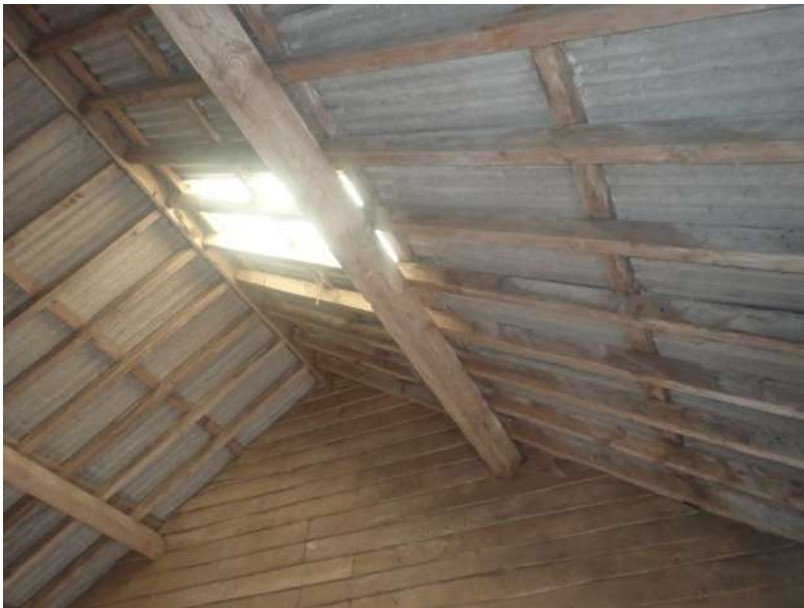
Plate 141: View of the roof supporting structure of Cell 4, from the east
