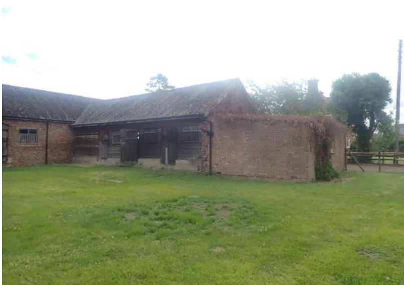
Plate 6: General view of the outbuilding complex, from the south-west
