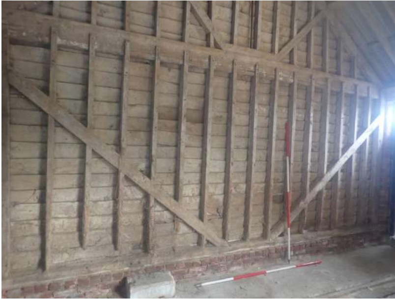
Plate 126: View of the west wall of Cell 3, from the east
