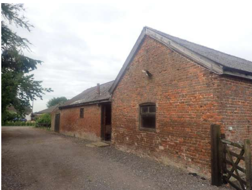
Plate 8: General view of the outbuilding complex, from the north-east
