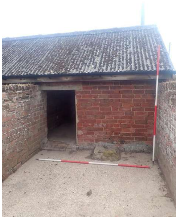
Plate 279: View of the exterior of the third sty, from the west
