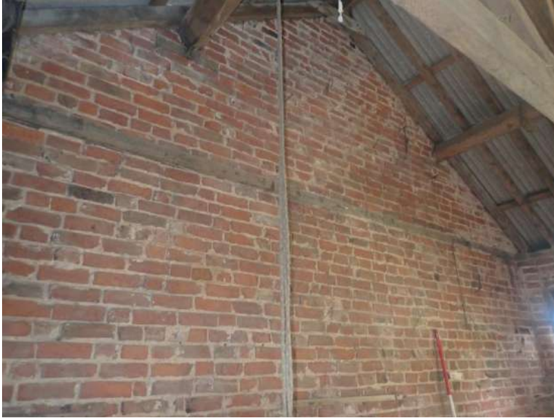
Plate 299: View of the south wall of Cell 7, from the north-east
