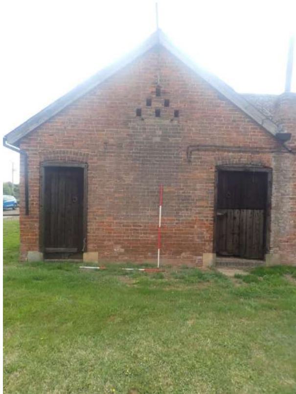
Plate 105: View of the West Elevation of the North Range, from the west
