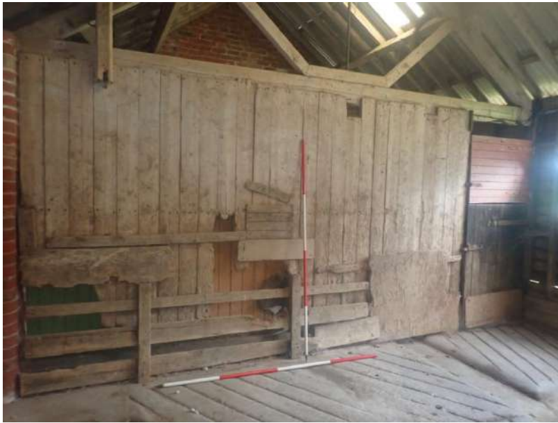
Plate 49: View of the south wall of Cell 1, from the north
