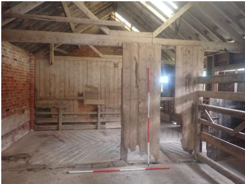
Plate 46: View of the internal timber partition within Cell 1, from the north
