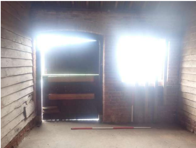
Plate 147: View of the north wall of Cell 4, from the south
