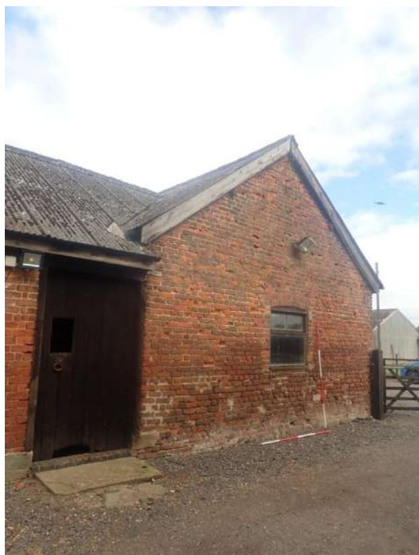
Plate 96: View of the East Elevation of the North Range, from the south-east
