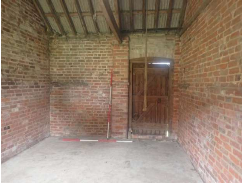
Plate 286: General view of the interior of Cell 7, from the west
