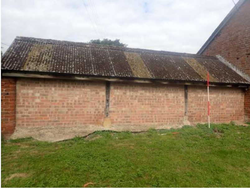
Plate 284: View of the East Elevation of the former piggery, from the east
