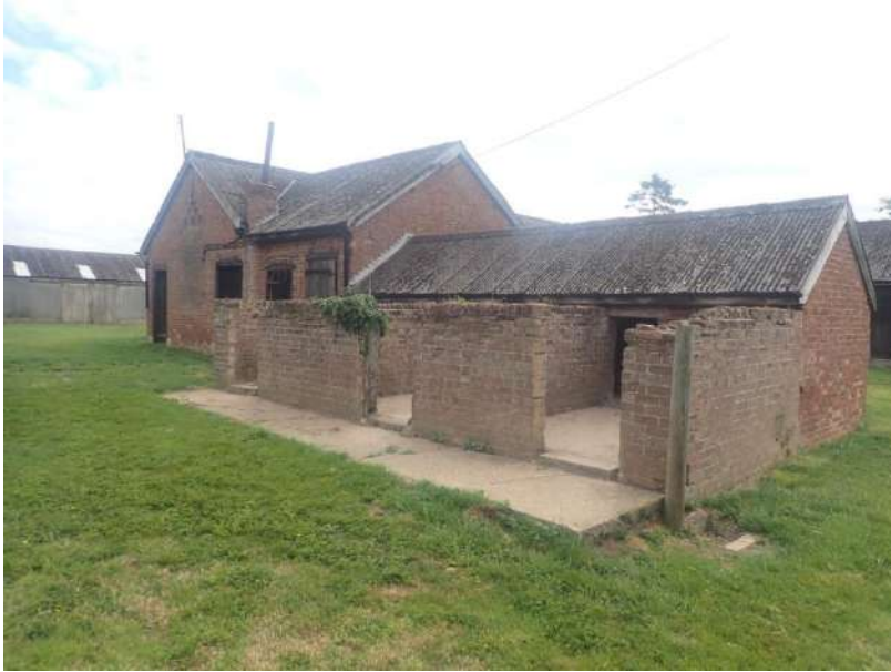
Plate 264: General view of the former piggery, from the south-west
