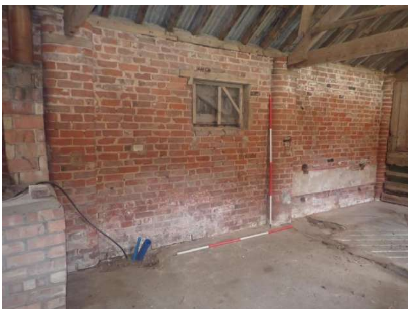
Plate 56: View of the east wall of Cell 1, from the north-west
