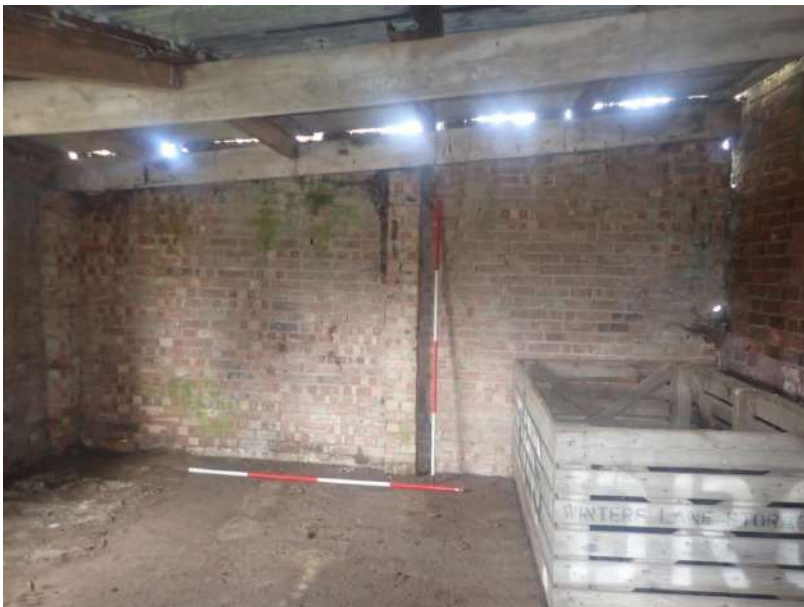
Plate 26: View of the west wall of the modern lean-to/garage, from the east
