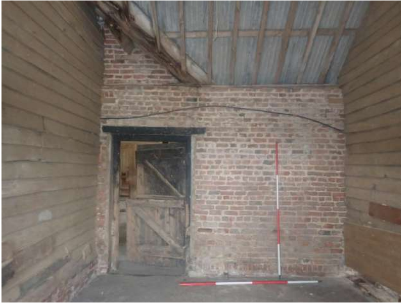
Plate 146: View of the south wall of Cell 4, from the north
