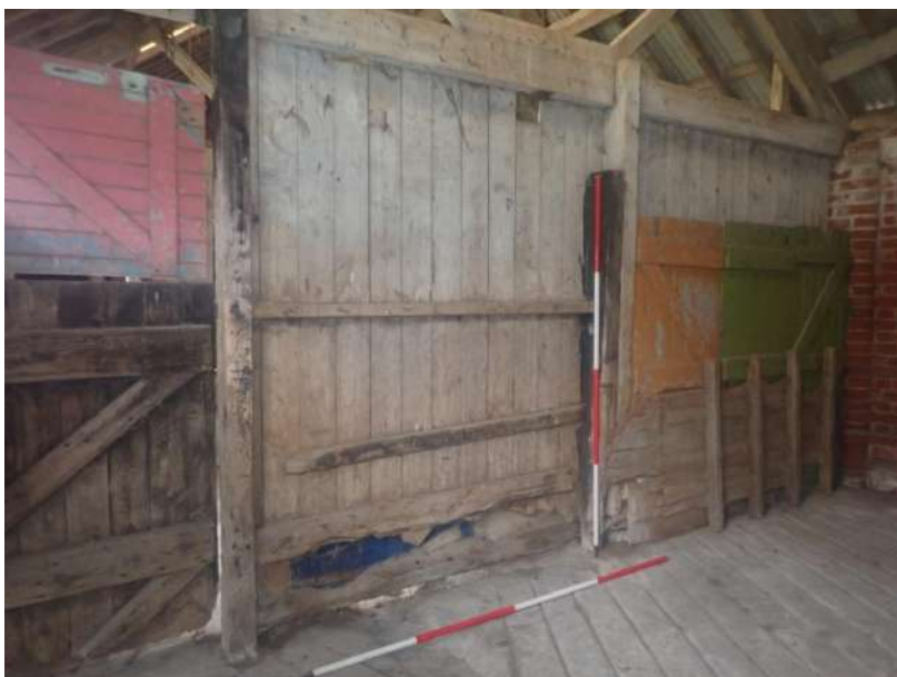
Plate 91: View of the north wall of Cell 2, from the south-west
