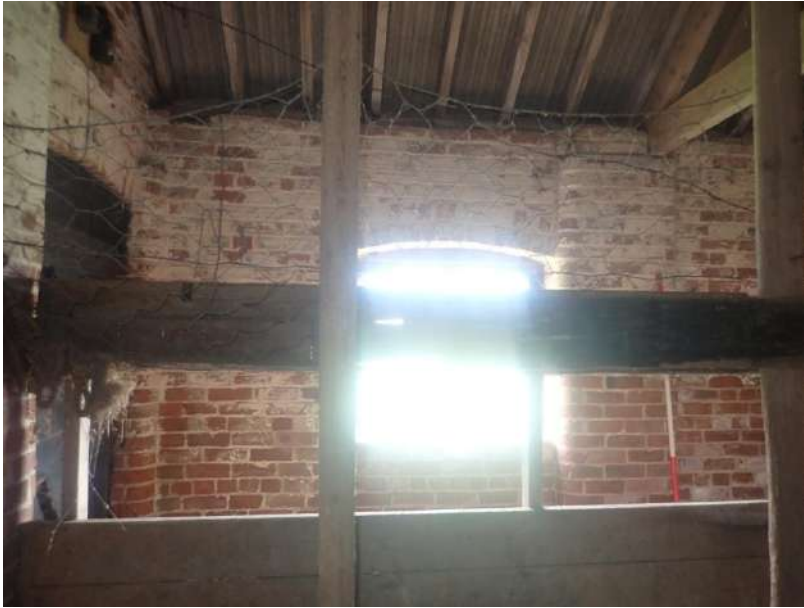
Plate 256: View of the north wall of Cell 6, from the south
