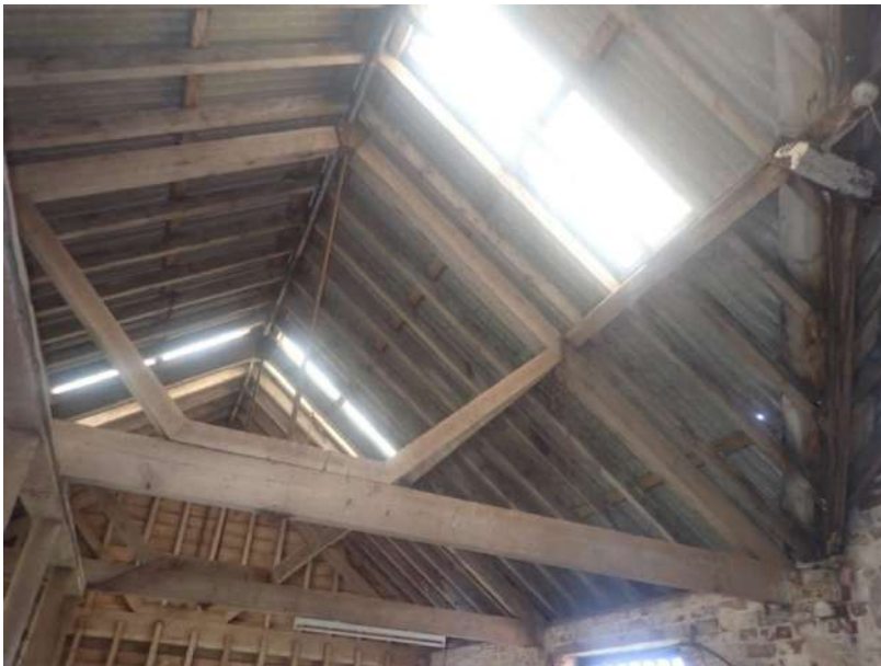
Plate 220: View of the roof supporting structure of Cell 6, from the west
