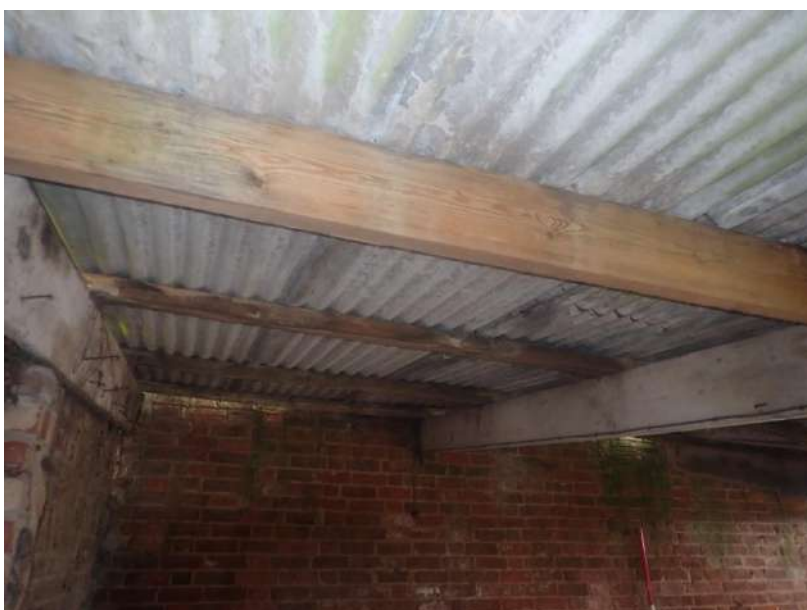
Plate 18: View of the roof supporting structure of the modern lean-to/garage, from the south
