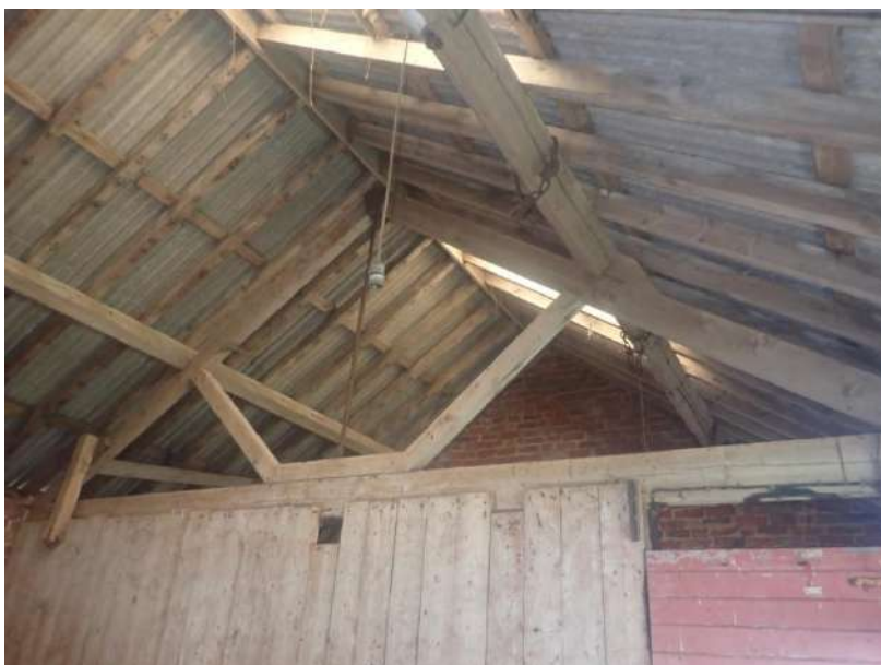
Plate 71: View of the roof supporting structure of Cell 1, from the north
