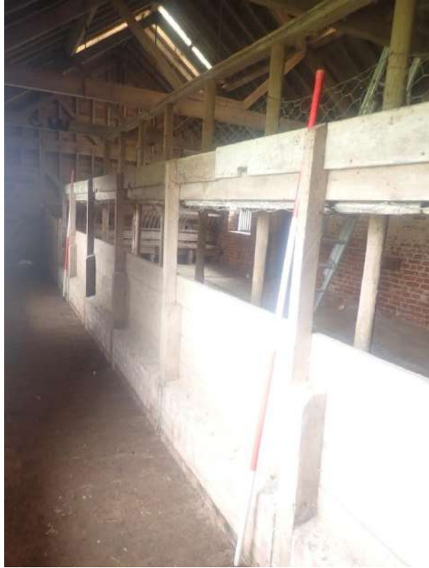
Plate 239: View of the timber fence along the southern side of the northern passageway of Cell 6, from the west
