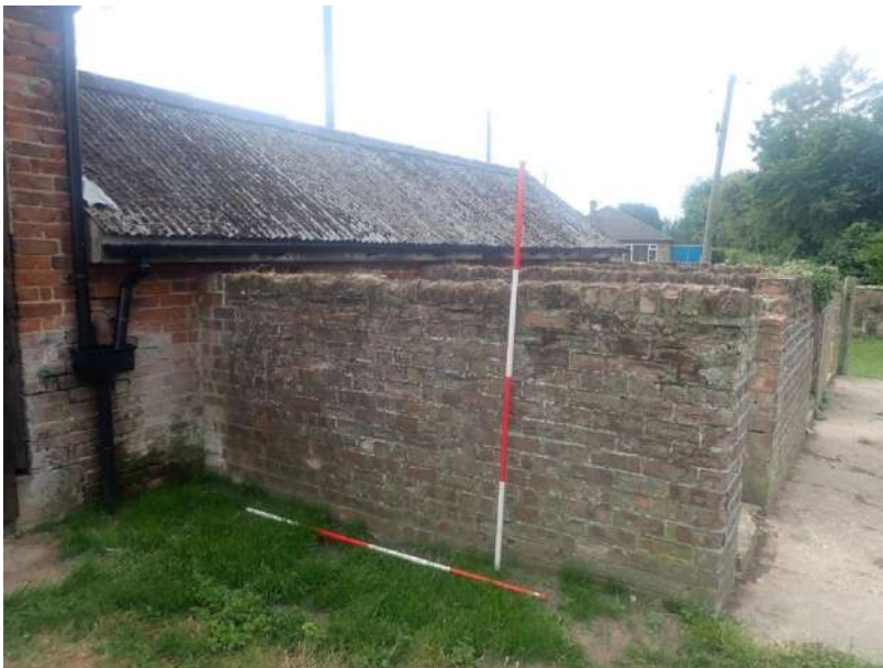
Plate 265: View of the northern boundary wall of the piggery, from the north
