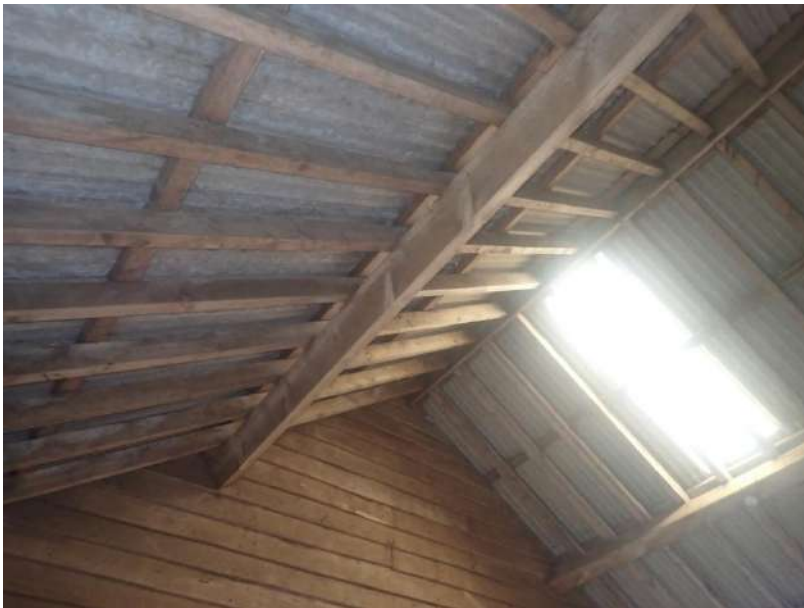
Plate 163: View of the roof supporting structure of Cell 5, from the east
