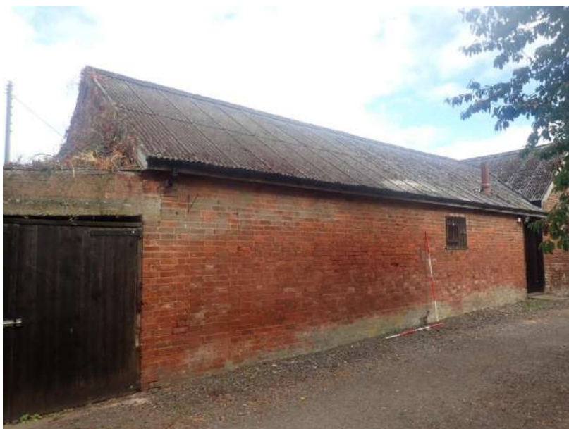
Plate 29: View of the East Elevation of Outbuilding 1, from the south-east
