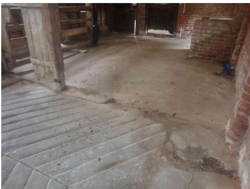
Plate 42: View of the flooring of Cell 1, from the south
