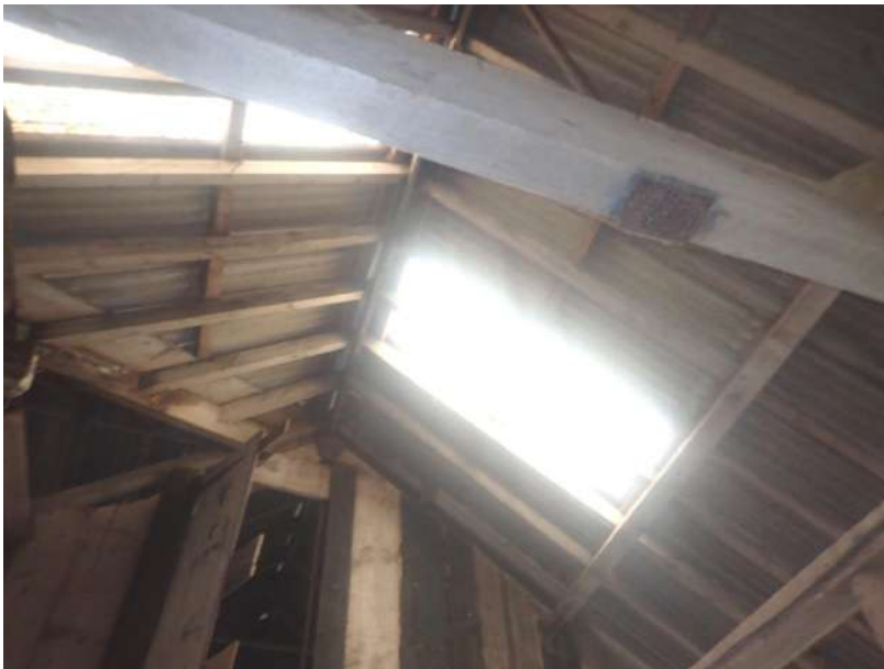
Plate 224: View of the roof supporting structure of Cell 6, from the east
