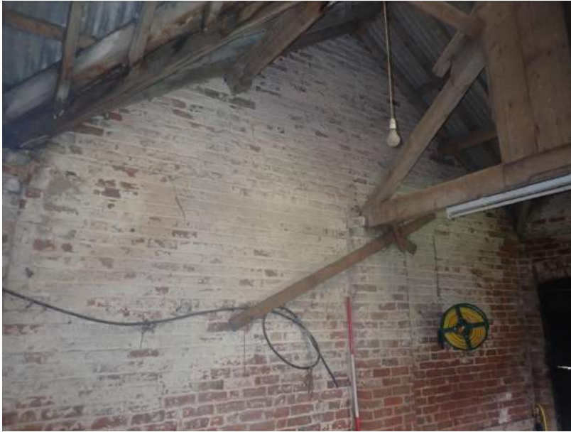
Plate 198: View of the south wall of Cell 6, from the north-east
