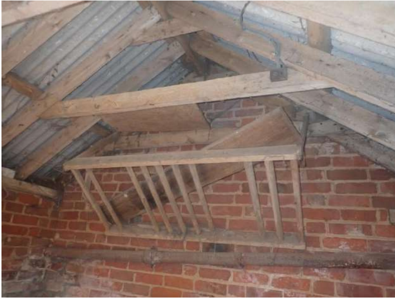
Plate 305: View of the north wall of Stie 1, from the south
