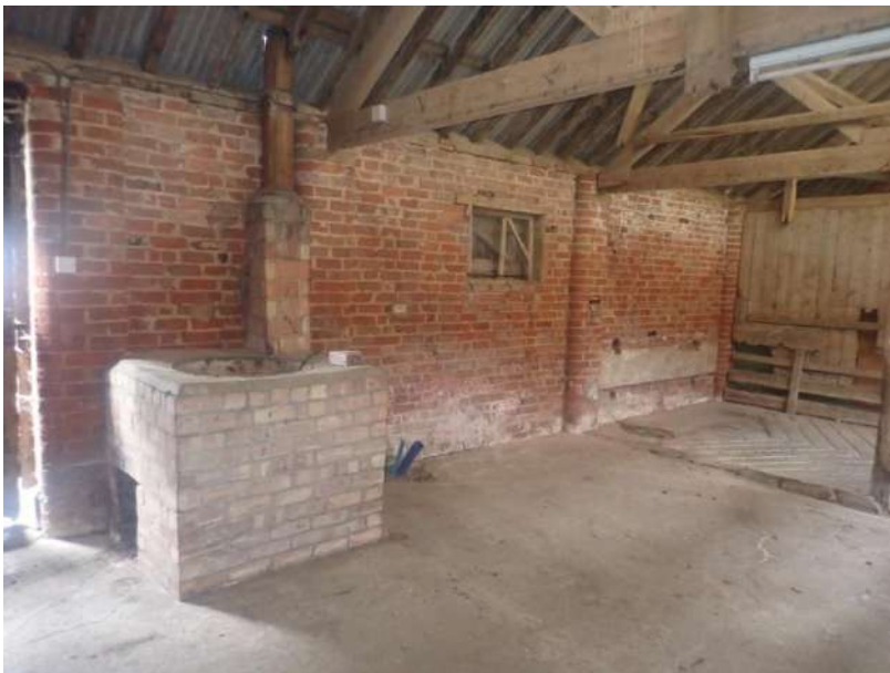
Plate 36: General view of the interior of Cell 1, from the north-west
