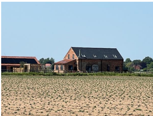
Fig. 13 – Dwelling 700m west of site.
