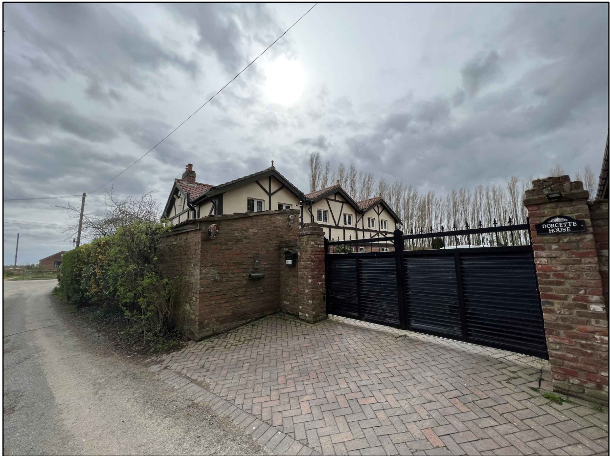
Existing gates viewed from north-east
