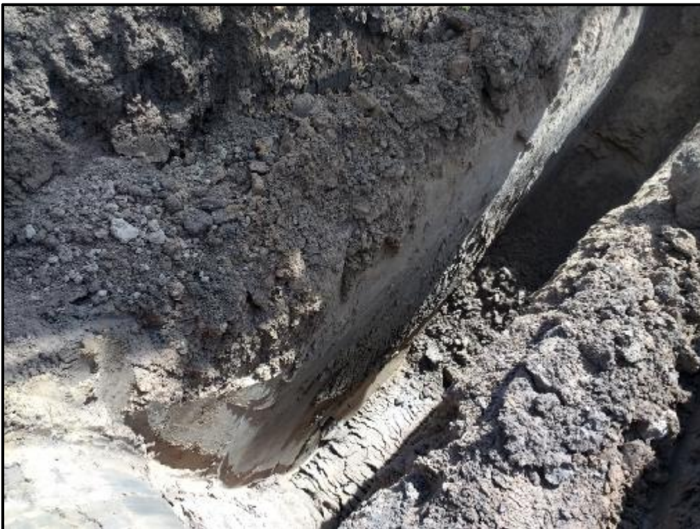
Inside of TP2
