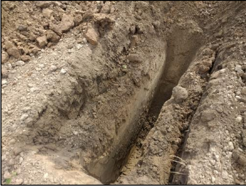
Inside of TP3
