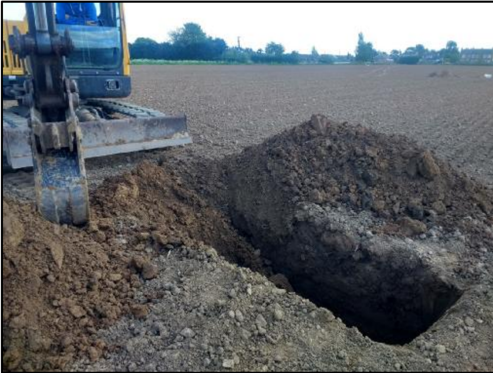
Location of TP4 (view towards south)
