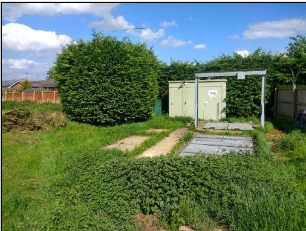
Pumping station near to southeast corner of site (view towards east)
