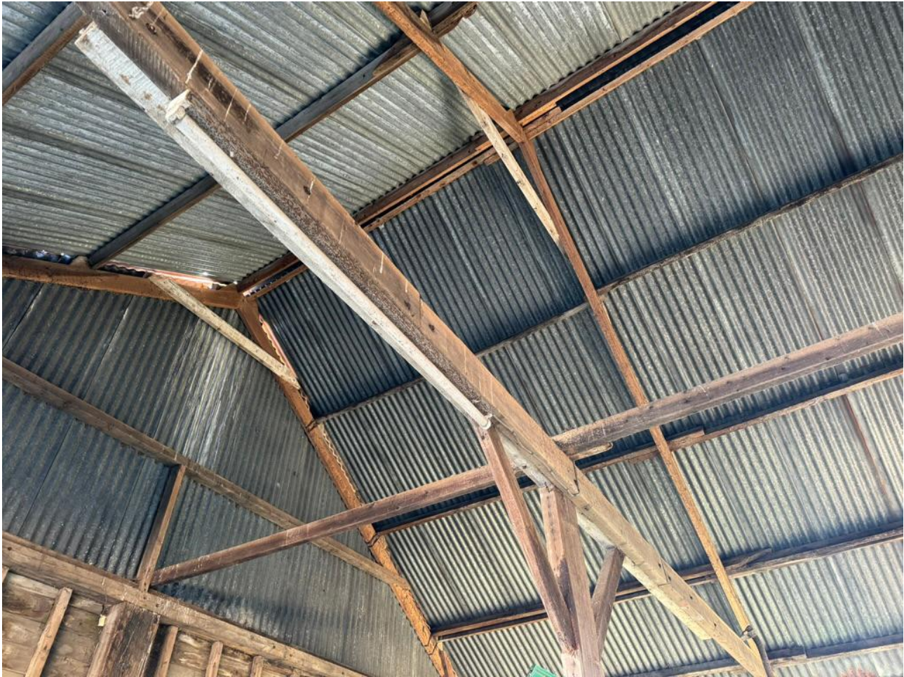
Image 13.0: Internal view of existing roof structure
