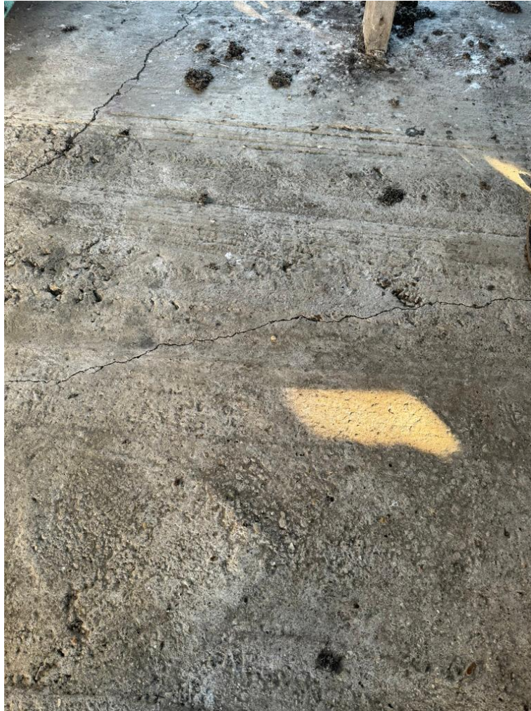
Image 15.0: View of floor slab.
