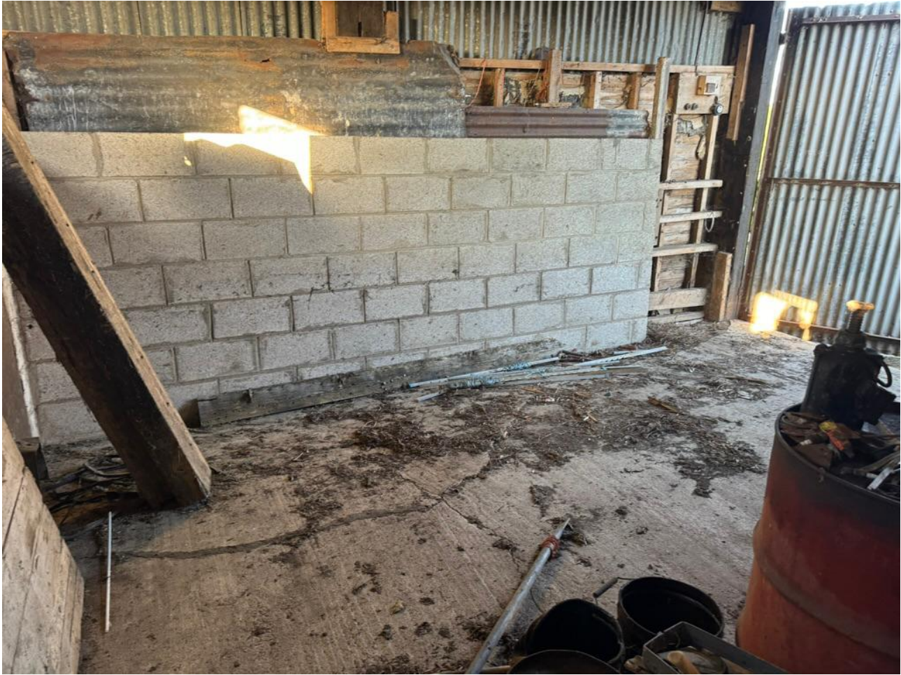
Image 22.0: Gable end of structure
