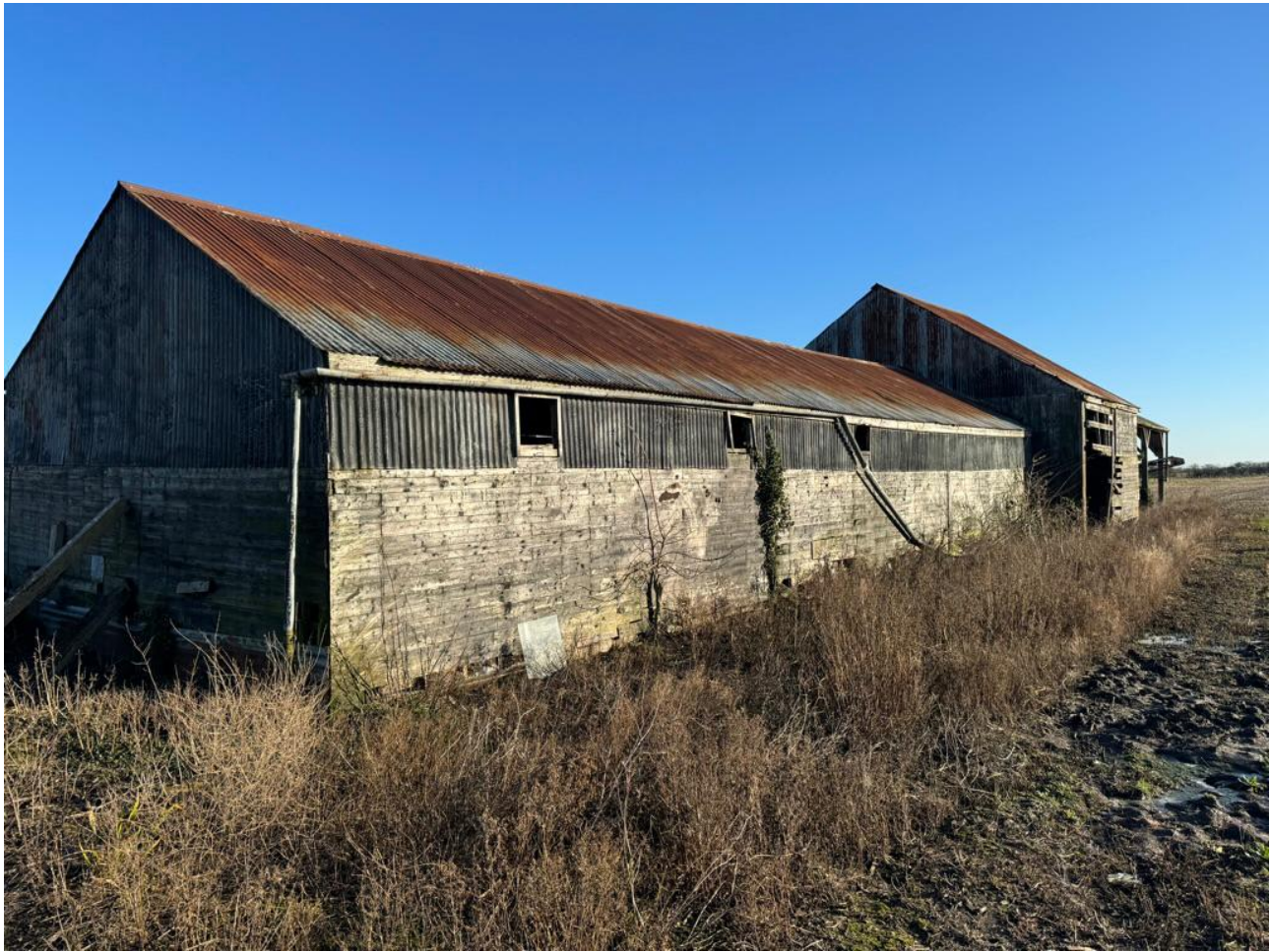
Image 18.0: View along roof and rear of Barn 4, with roof remaining intact
