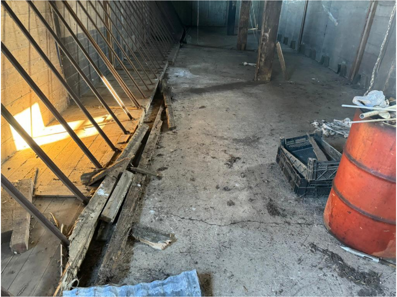
Image 21.0: View of finished concrete floor
