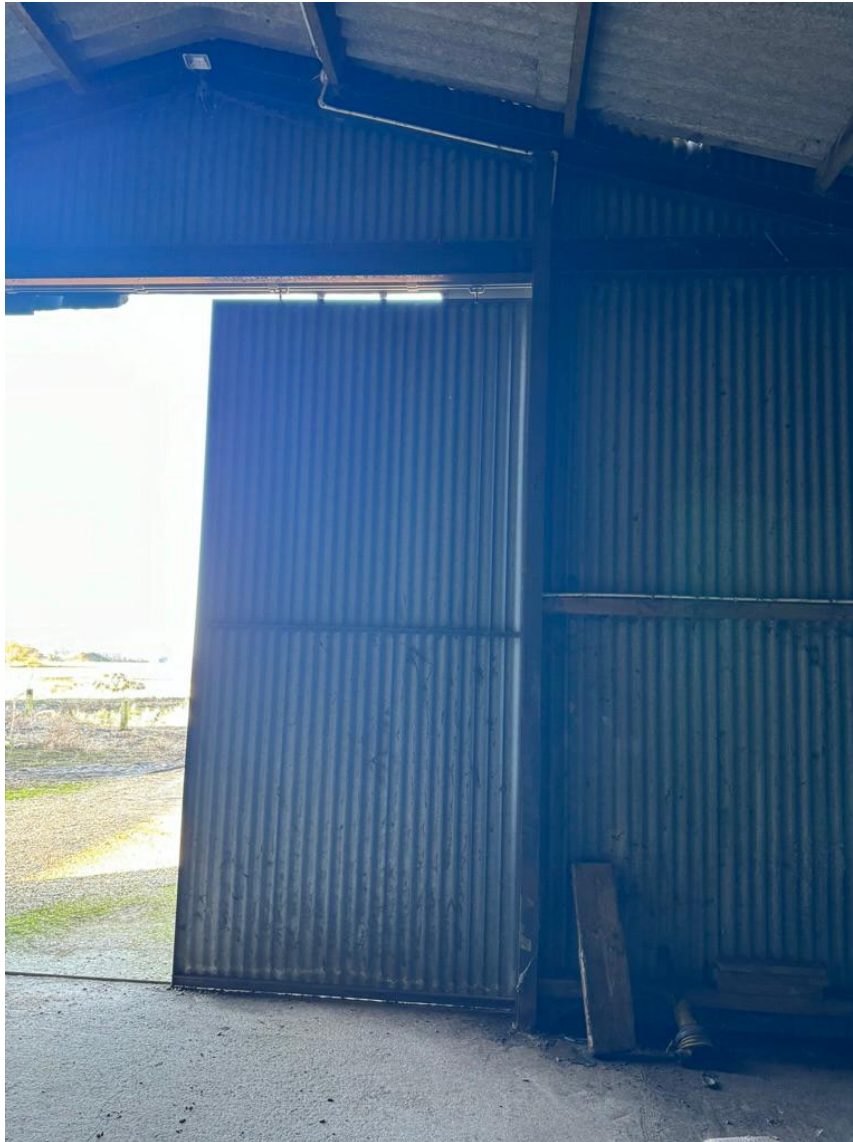
Image 4.0: Sliding doors to the front of the Barn
