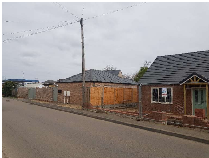
Figure 9 – New build Bungalow, Style A to the North-West on Church Gate.
