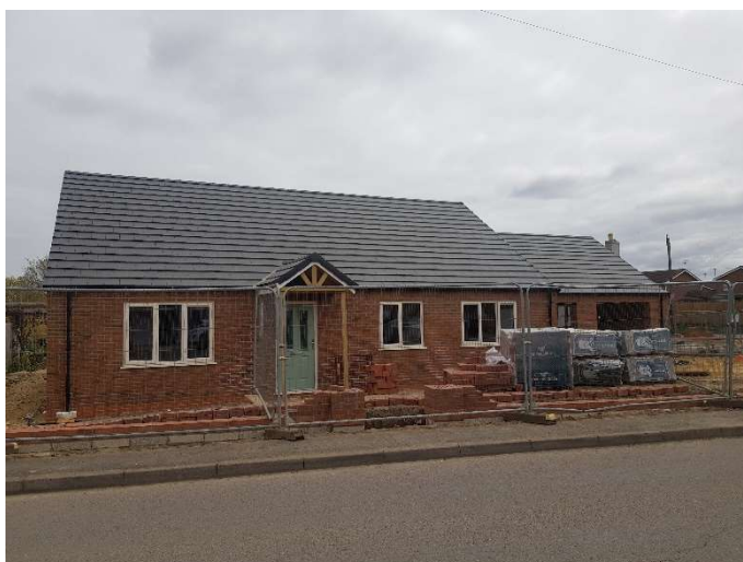
Figure 10 – New build Bungalow, Style B to the North-West on Church Gate.
