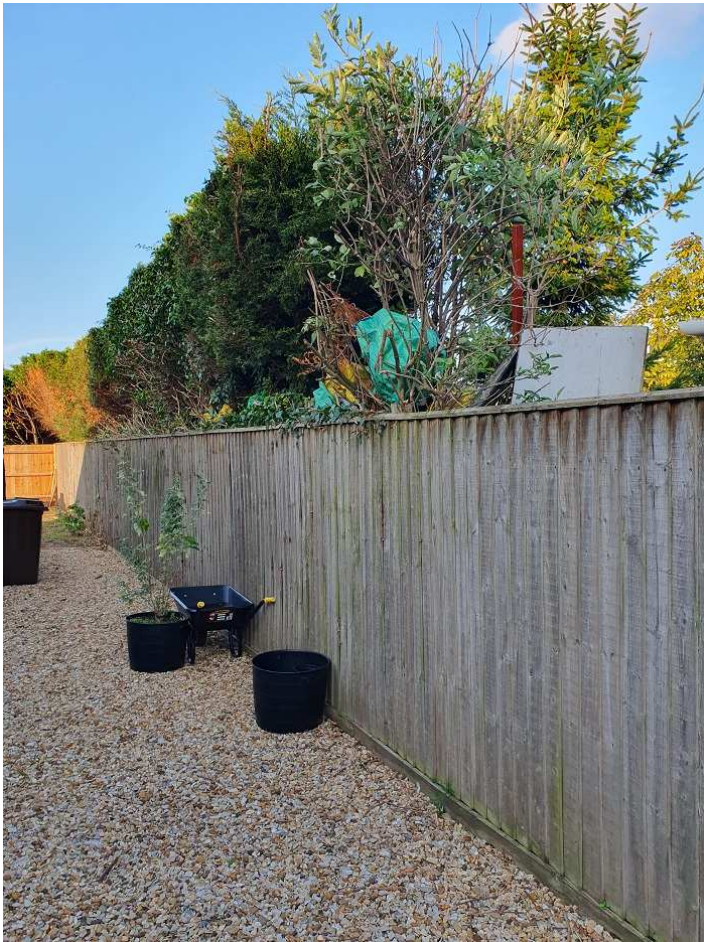
View of fence & hedge looking north east
