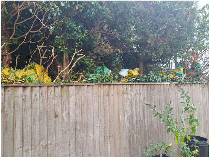
View towards fence with conifer hedge* and bags** inserted into gaps
