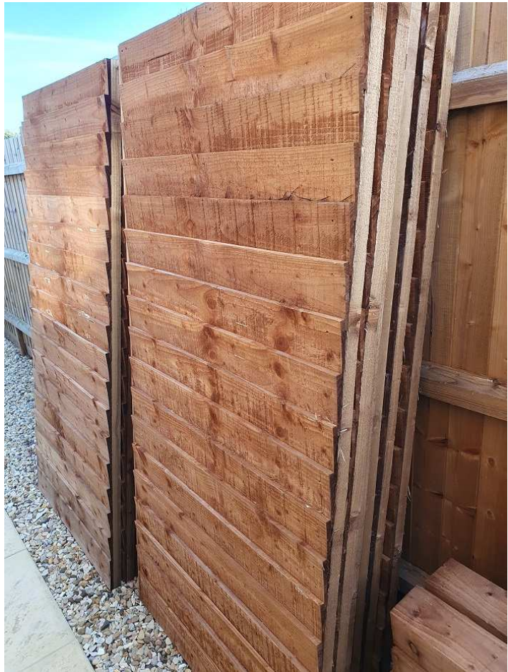
View of proposed close boarded fence extension awaiting installation (note: boards will be vertical when installed to match existing)
