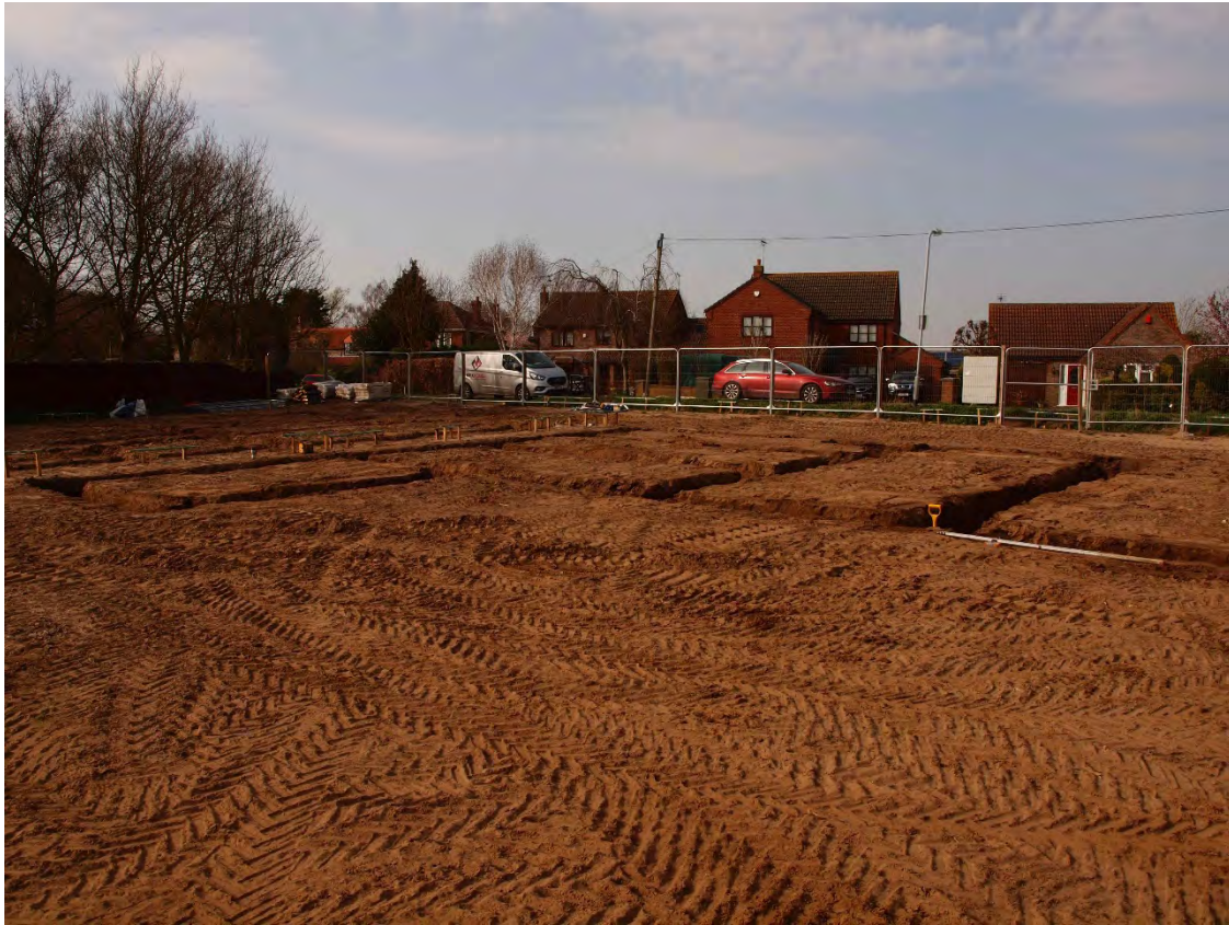
Plate 3: General view of plot 2 looking north-west
