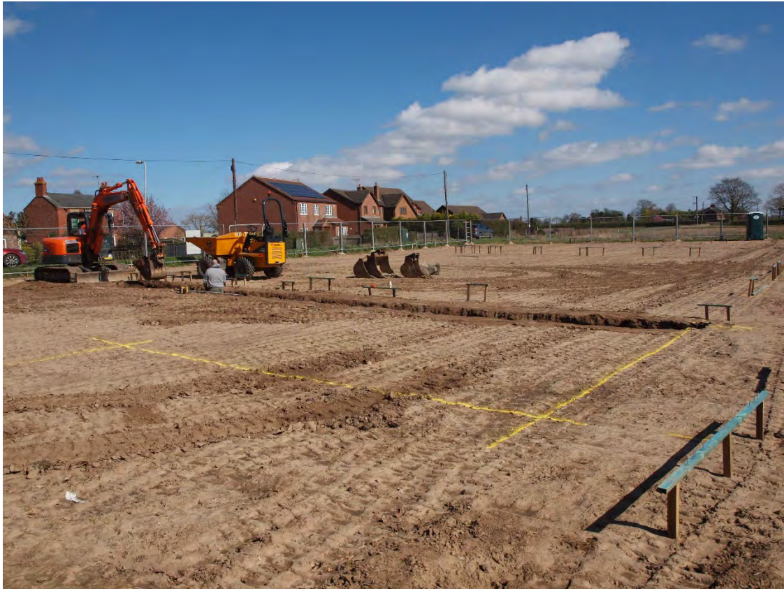
Plate 1: General view of site looking east
