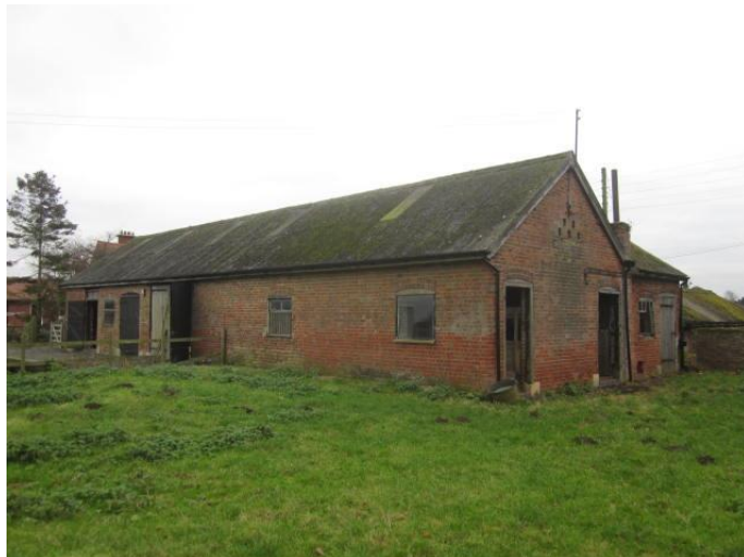
Photograph # 2 North – West Facing Elevation
