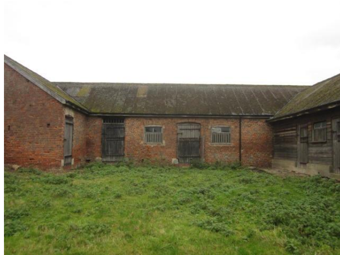
Photograph # 4 South Facing Elevation
