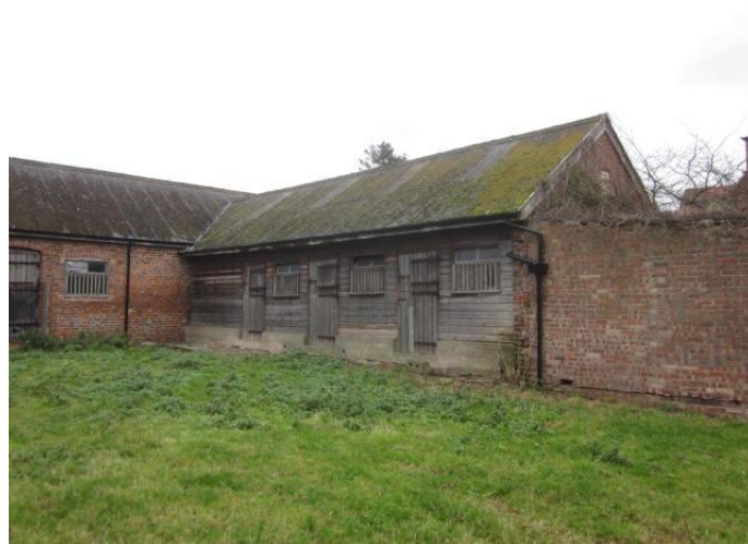
Photograph # 5 West Facing Elevation (timber Infill Wall Panels)
