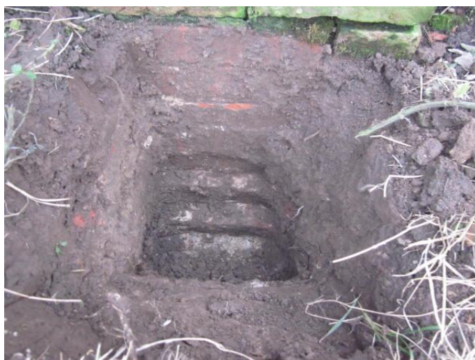
Photograph # 12 Typical Foundation
