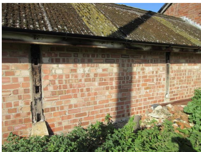
Photograph # 6 (Taken Oct 2021) Low Level Pens – Adjusted Masonry – Later ‘Common’ Units
