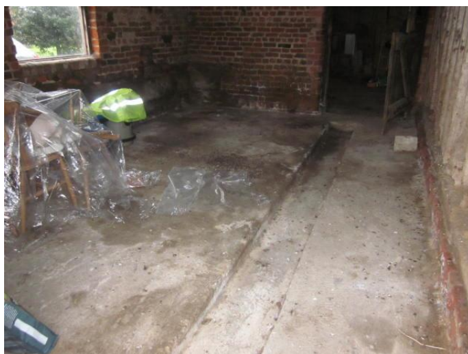
Photograph # 11 Typical Ground Floor
