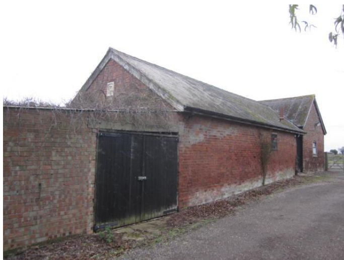
Photograph # 8 East Facing Elevation – Later Garage constructed using 'Common' units
