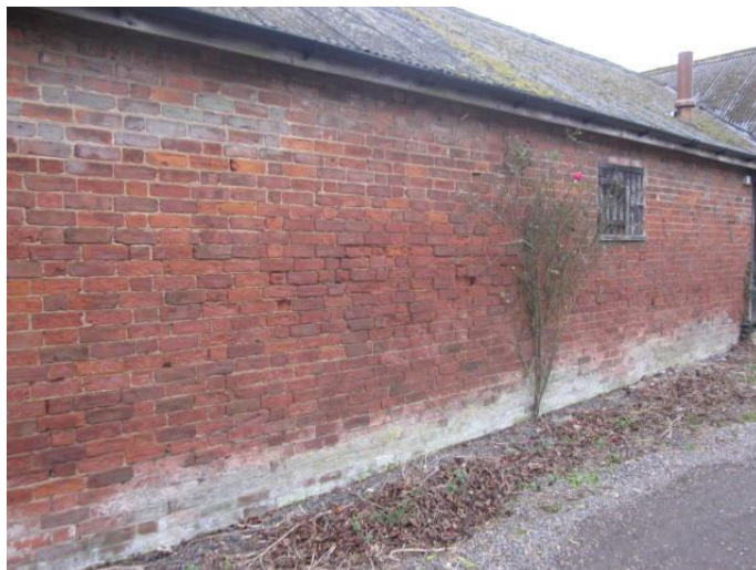
Photograph # 7 East Facing Elevation
