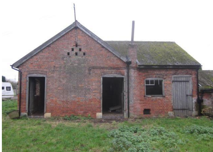
Photograph # 3 West Facing Elevation
