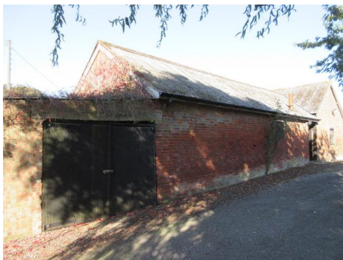
Photograph # 8 (Taken Oct 2021) East Facing Elevation – Later Garage constructed using 'Common' units
