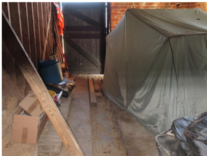
Photograph # 11 (Taken Oct 2021) Typical Ground Floor
