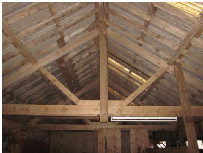
Photograph # 9 Typical Roof
