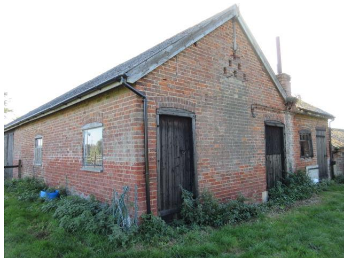
Photograph # 2 (Taken Oct 2021) North – West Facing Elevation
