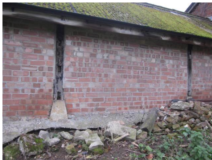
Photograph # 6 Low Level Pens – Adjusted Masonry – Later ‘Common’ Units
