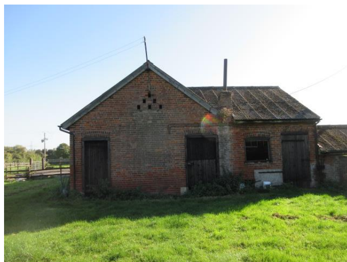
Photograph # 3 (Taken Oct 2021) West Facing Elevation
