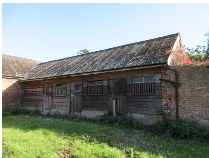
Photograph # 5 (Taken Oct 2021) West Facing Elevation (timber Infill Wall Panels)
