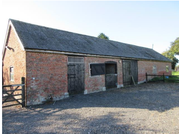
Photograph # 1 (Taken Oct 2021) North Facing Elevation
