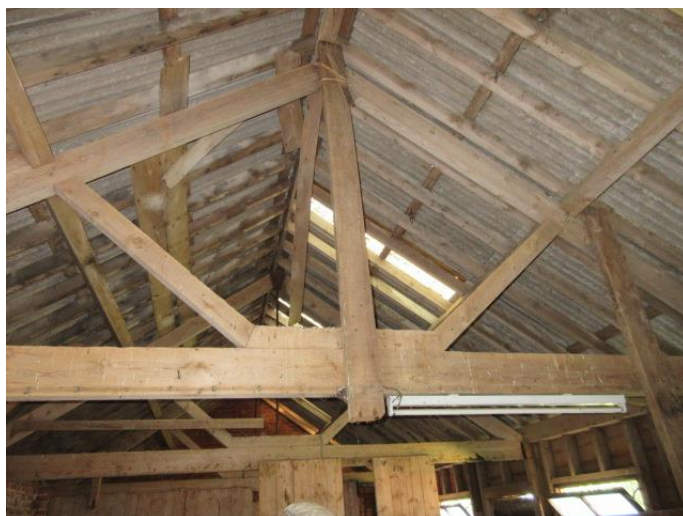
Photograph # 9 (Taken Oct 2021) Typical Roof
