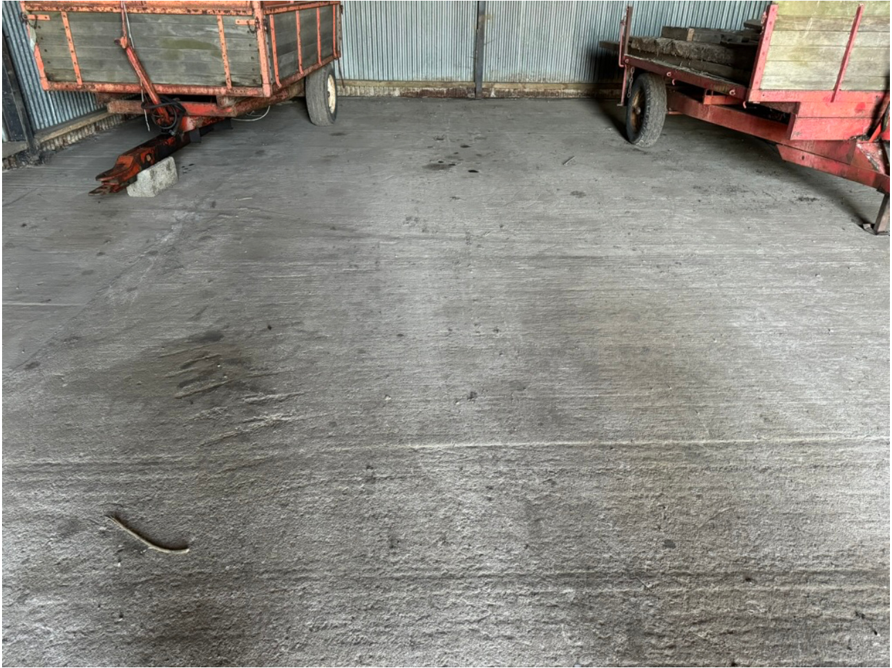
Image 6.0: Existing concrete floor, noted as being intact and functioning as originally intended
