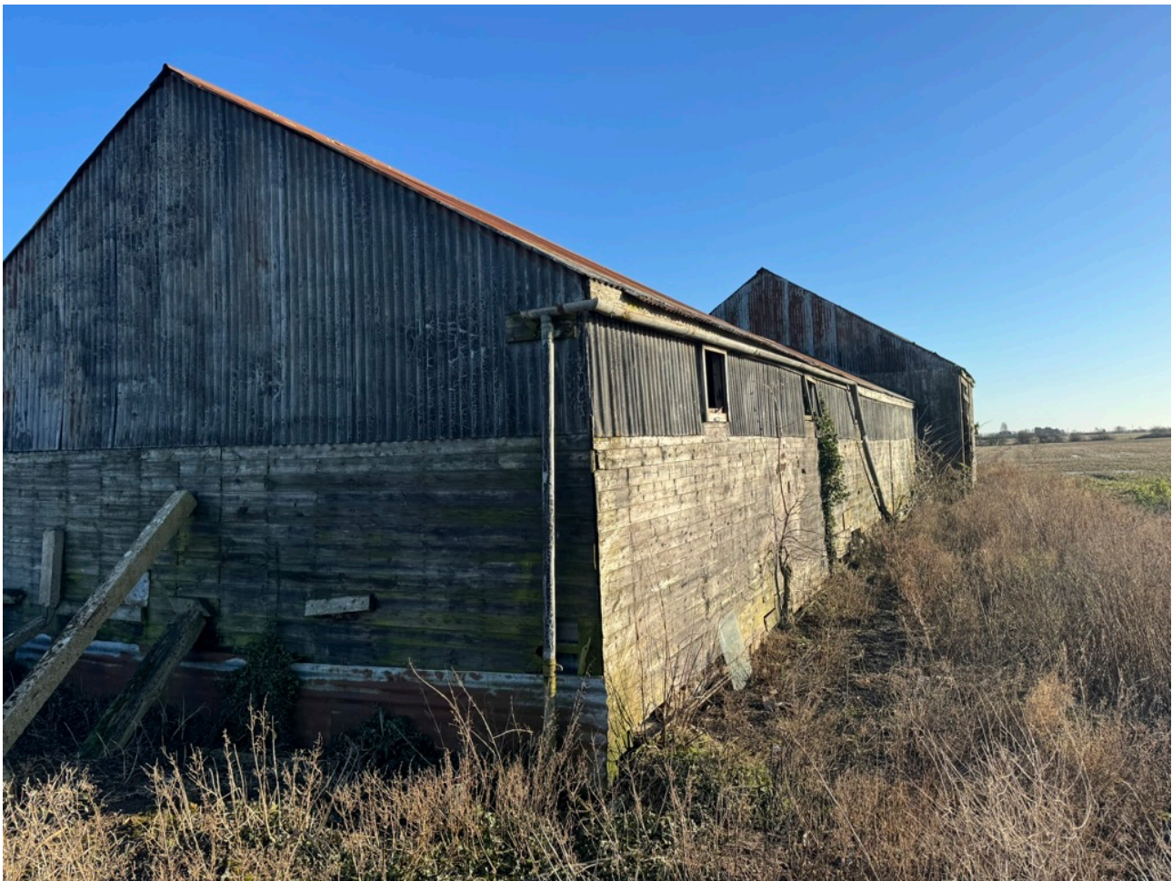
Image 16.0: Gable and rear elevation of Barn 4
