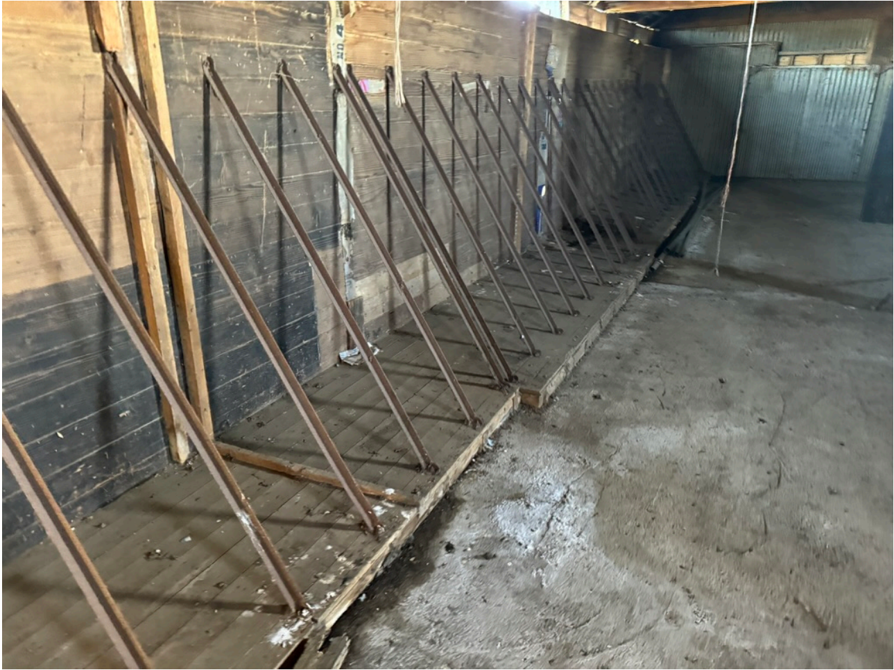
Image 19.0: Props between rear elevation of floor of barn 4
