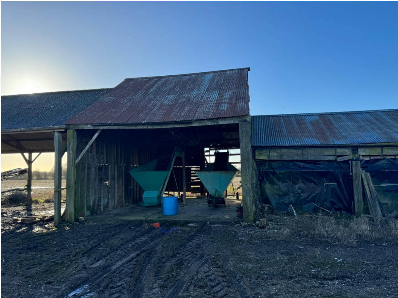
Image 12.0: External view to front of Barn 2
