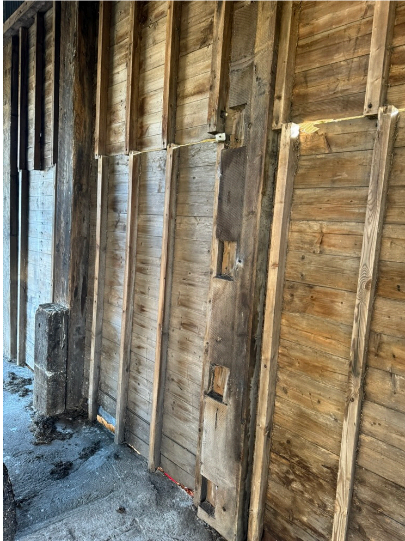
Image 14.0: Timber columns, formed of railway sleepers set to side elevations.
