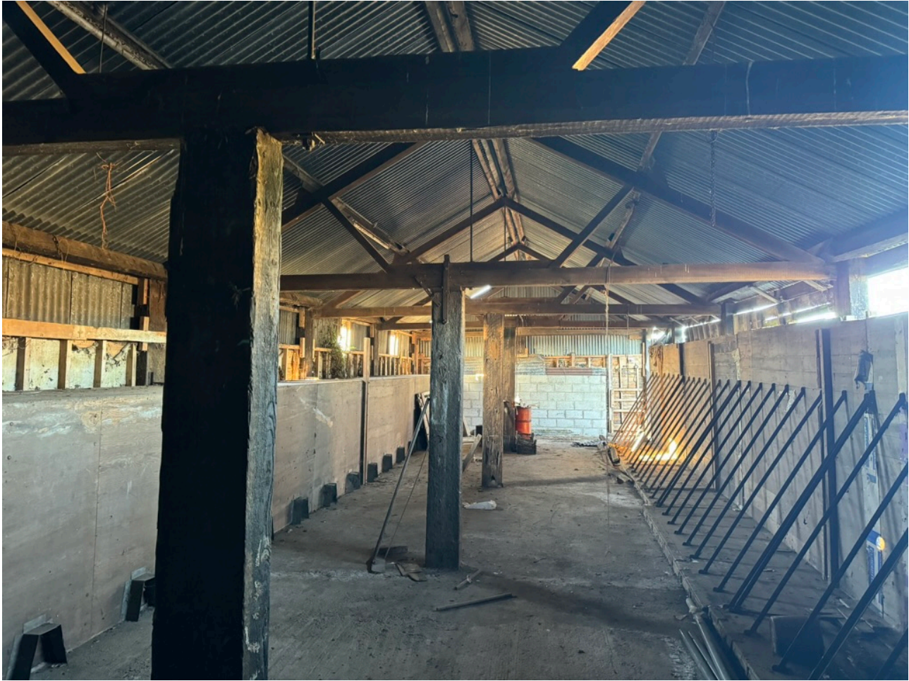
Image 20.0: Hand cut timber roof with timber supports formed from railway sleepers
