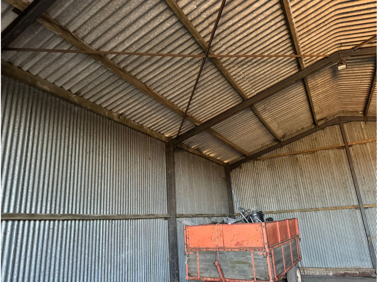
Image 2.0: View of cross bracing, removing longitudinal sway due to wind loading
