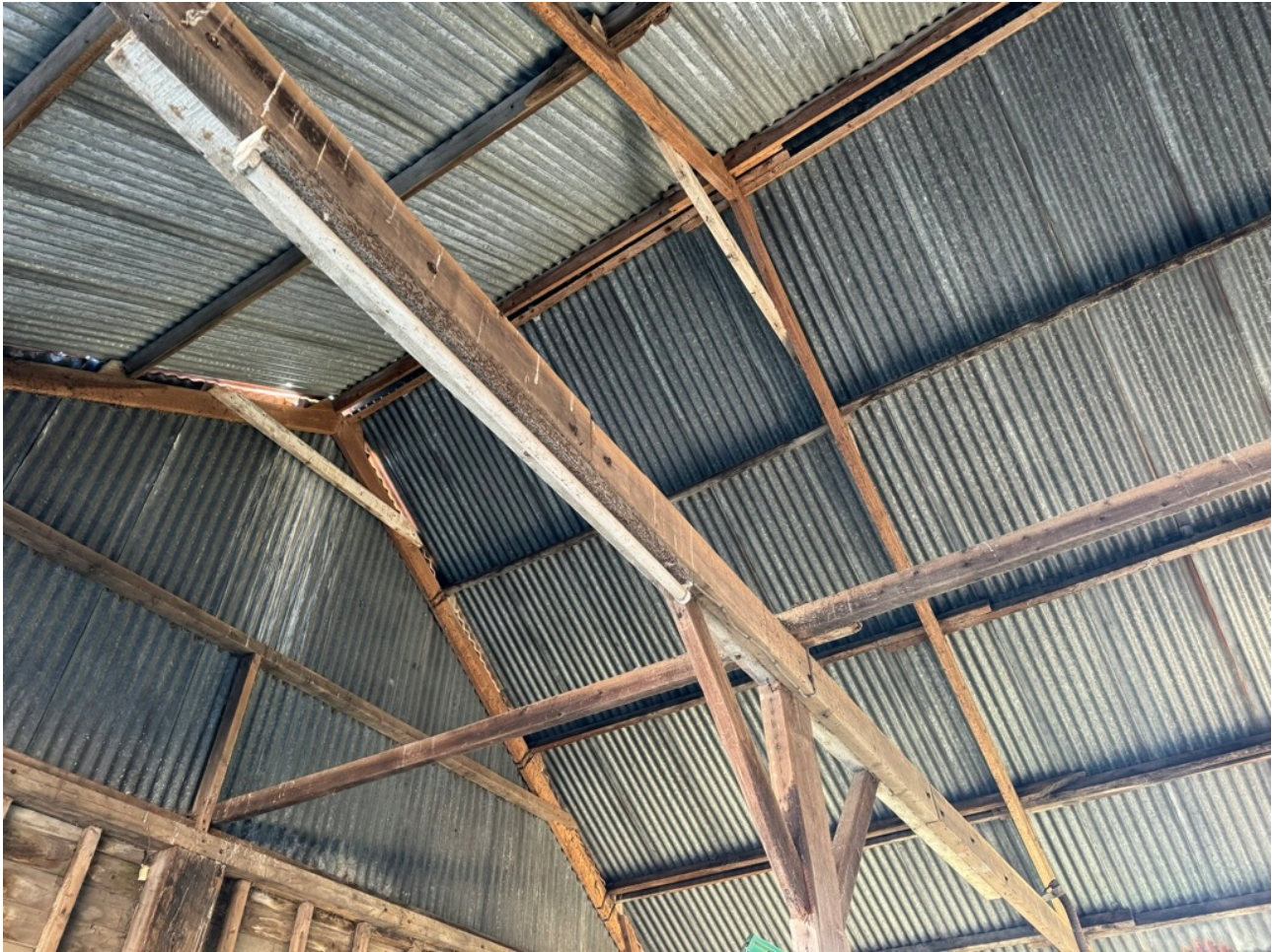
Image 13.0: Internal view of existing roof structure
