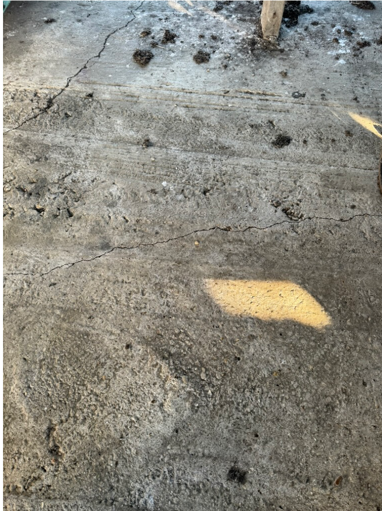
Image 15.0: View of floor slab.
