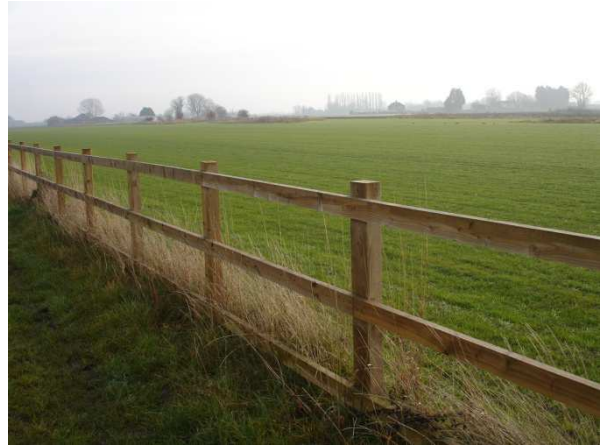
Lincolnshire post and rail fencing to perimeters
