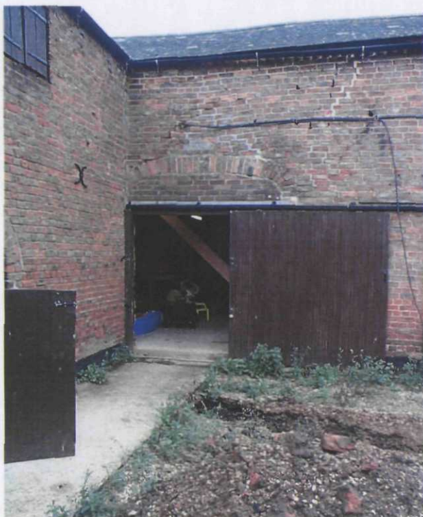
Plate 3 Main Barn, blocking and truncation of arched entrance in northwestern elevation, looking southeast
