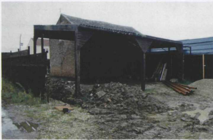
Plate 1 General view of barns (also showing unrecorded modern open barn), looking north
