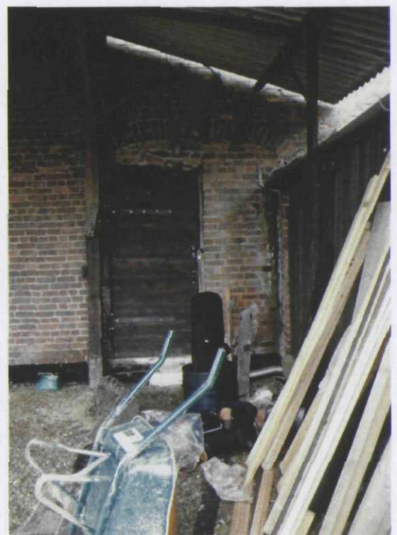
Plate 4 Main Barn, blocked arched entrance in southeasterly elevation, obscured by cattle shed, looking north
