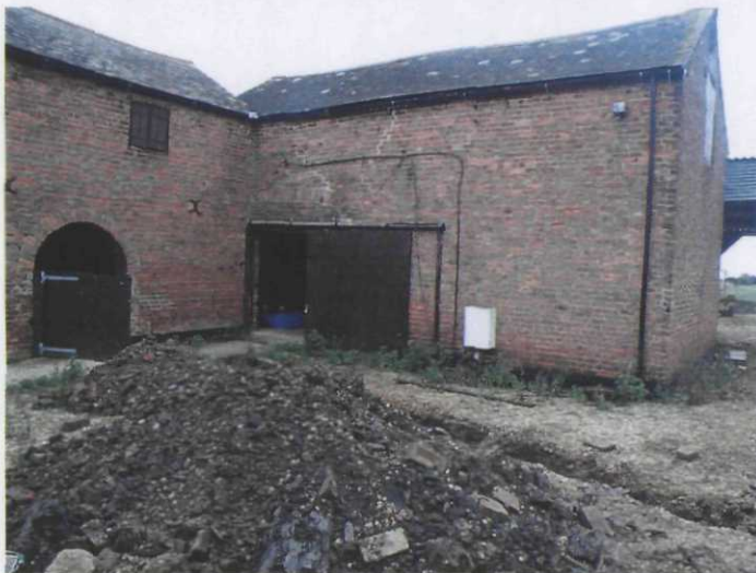
Plate 2 Main Barn, northeastern elevation, looking east
