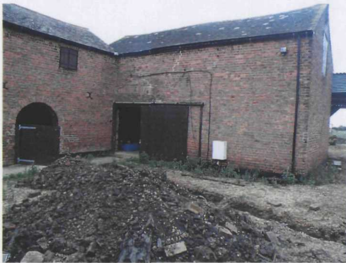
Plate 2 Main Barn, northeastern elevation, looking east
