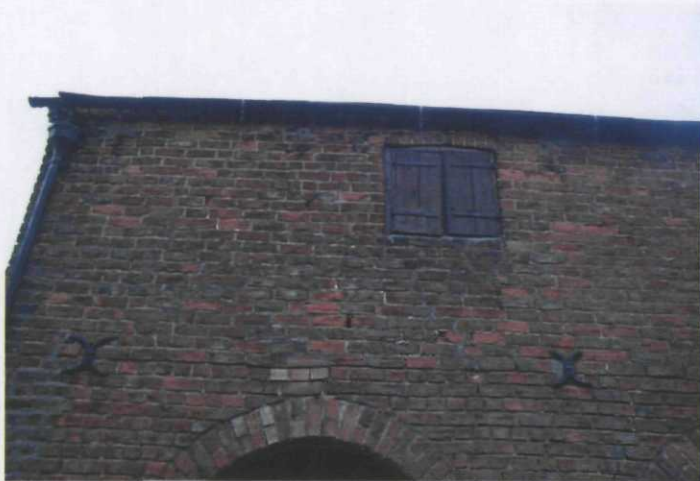
Plate 10 Stable Block, example of timber framed and shuttered window, looking northeast
