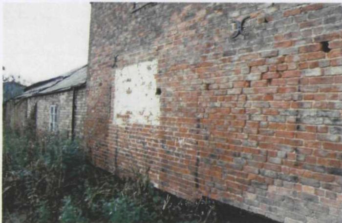
Plate 12 Stable Block, northeastern elevation, showing scarring of removed lean-to structure, looking south
