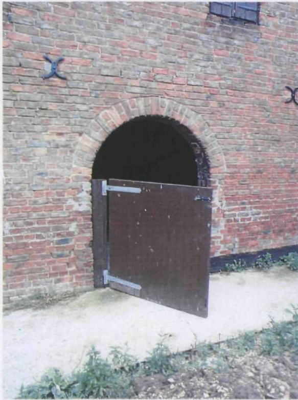
Plate 9 Stable Block, arched entrance with stable door, looking east
