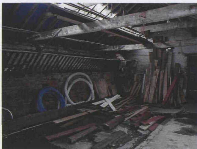
Plate 19 Cattle Shed, northwestern compartment showing hay rack, looking east-northeast
