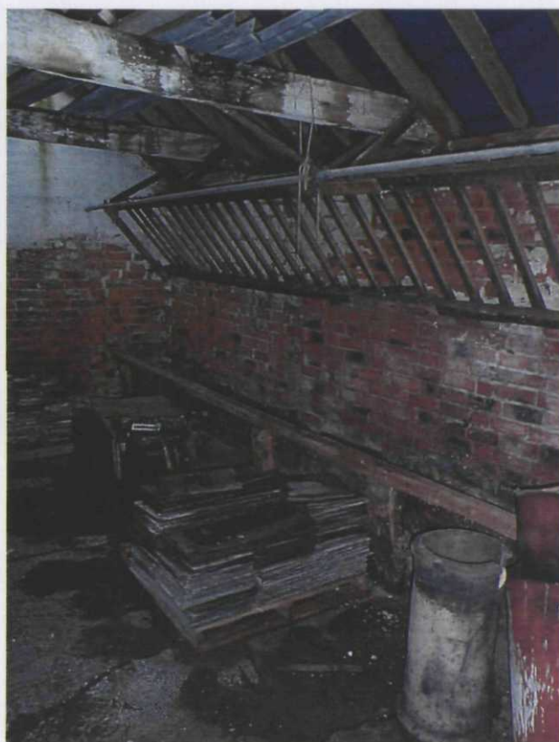
Plate 20 Cattle Shed, southeastern compartment showing feed trough and hay rack, looking north-northwest
