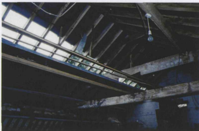
Plate 18 Cattle Shed, showing roofing trusses, looking east-northeast
