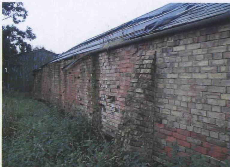
Plate 17 Cattle Shed, northeastern elevation with brick buttresses, looking south
