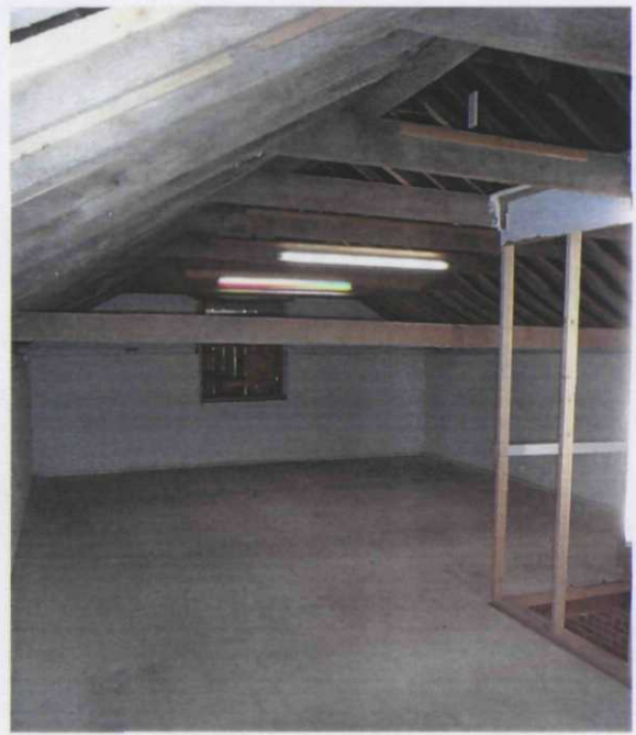
Plate 7 Main Barn, first roof showing re-roofing and newly inserted floor, looking east
