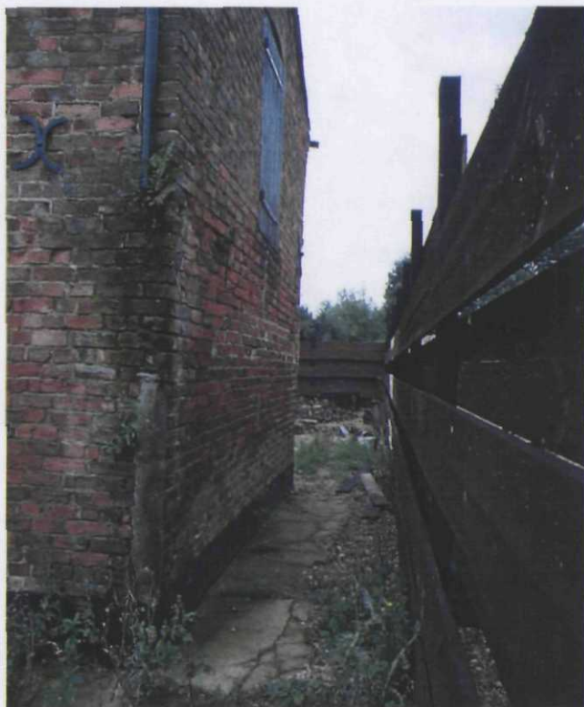
Plate 11 Stable Block, northwestern gable showing door to overhead hay loft, looking south-southwest
