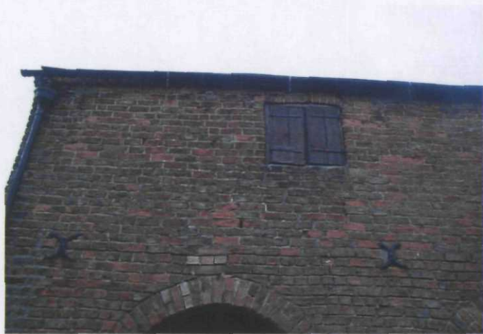
Plate 10 Stable Block, example of timber framed and shuttered window, looking northeast
